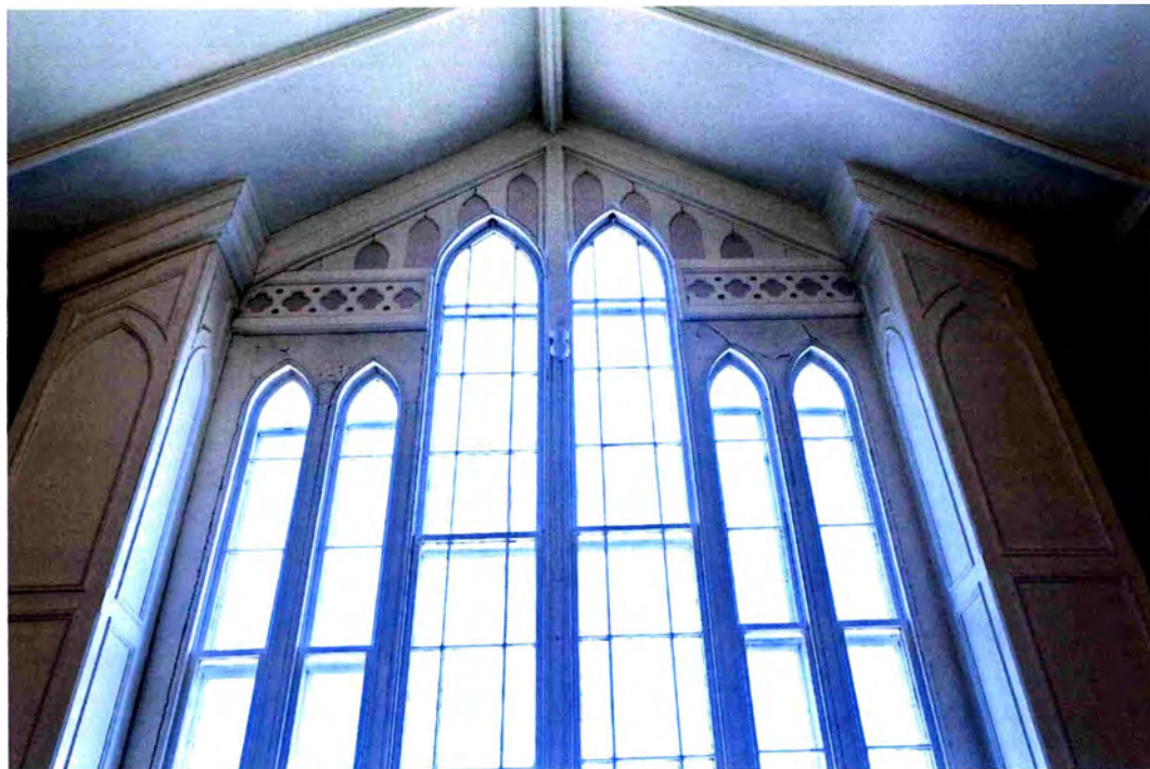
Photo 14. Interior view north of large window above gallery.
