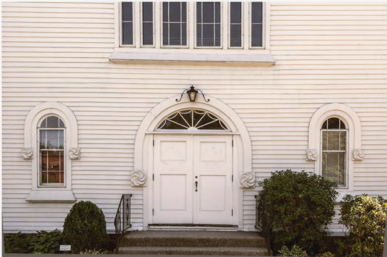
Photo 2. Plainville Congregational Church, Plainville, Hartford County, Connecticut, view south, showing main entrance and flanking round headed windows with fluted bosses and fanlight over front door. August 29, 2011, Tod Bryant.
