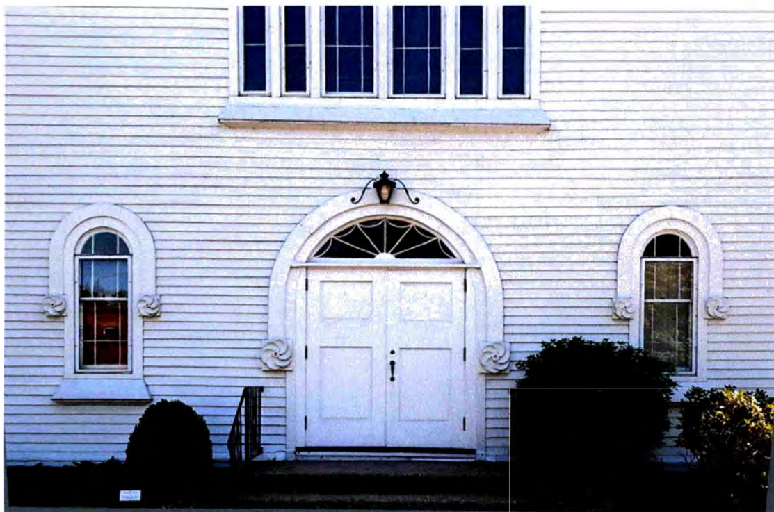
Photo 2. Facade, view south, showing main entrance and flanking windows with rounded arches and rosettes and fanlight.
