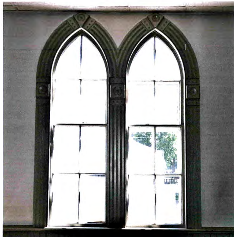
photo 20. Music room addition interior, view south showing pointed arch windows and moldings.
