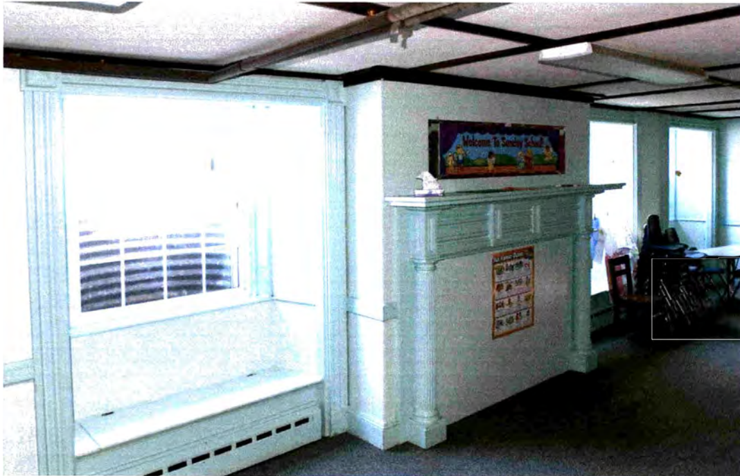
Photo 21. Fireplace room, view southwest showing fireplace.
