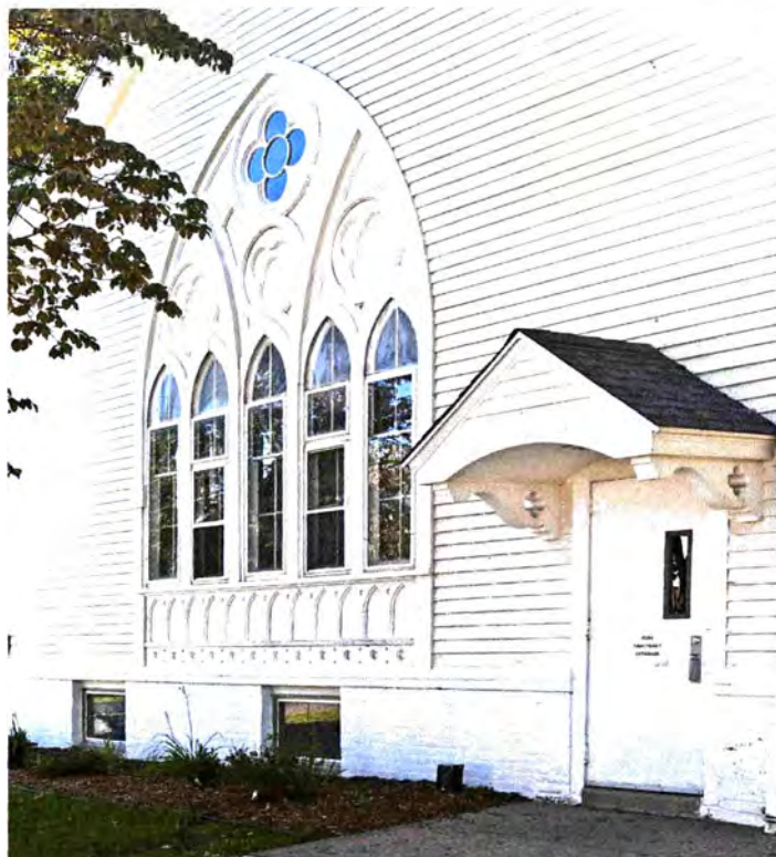
Photo 10. Music room addition, west elevation, view southeast, showing large lancet arch window group.
