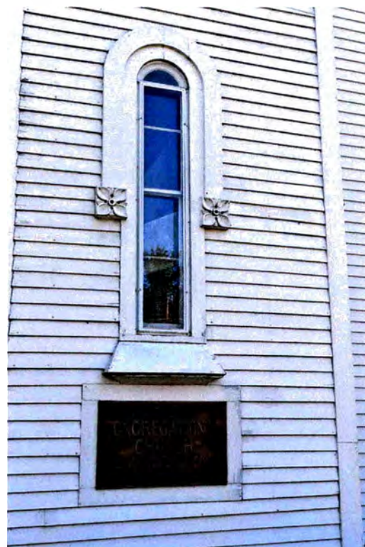
Photo 6. Plainville Congregational Church, Plainville, Hartford County, Connecticut, view south, tower, north elevation, showing round headed window and fluted bosses. August 29, 2011, Tod Bryant.
