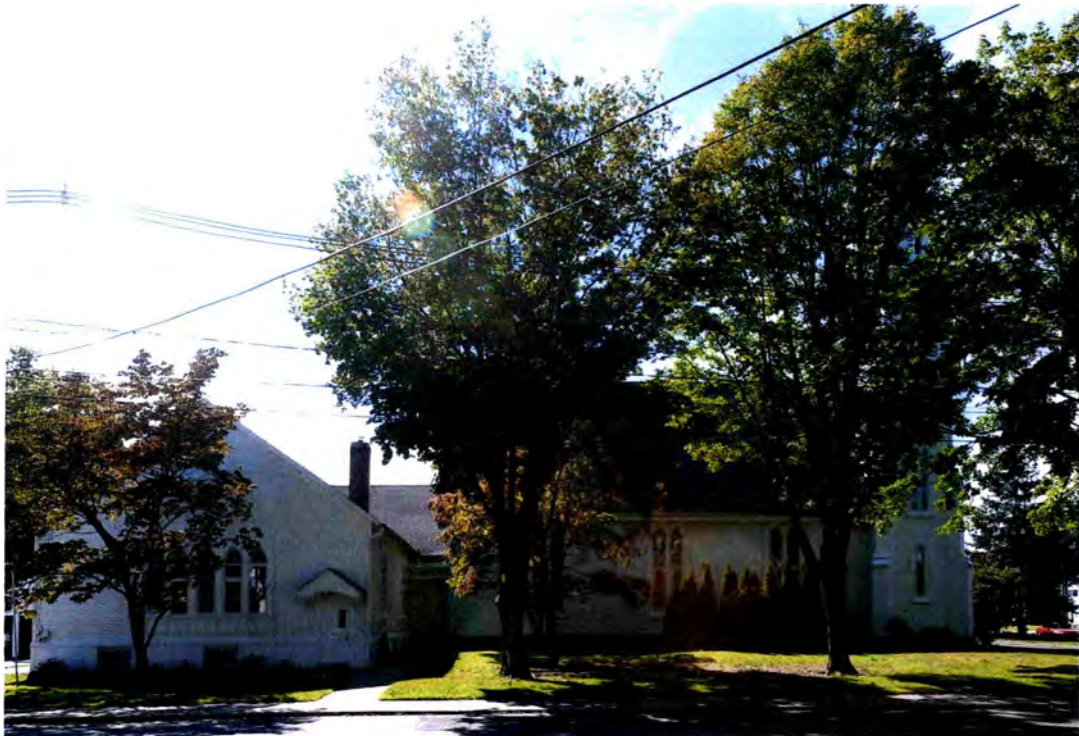
Photo 8. Plainville Congregational Church, Plainville, Hartford County, Connecticut, view west showing east elevation, August 29, 2011, Tod Bryant..
