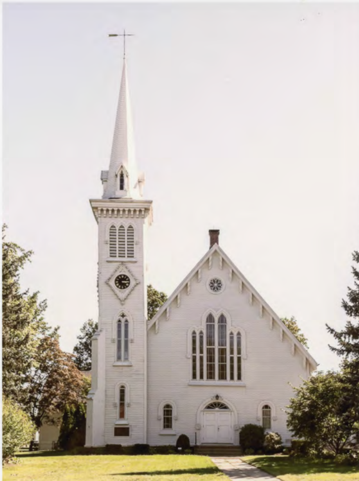
Photo 1. Plainville Congregational Church, Plainville, Hartford County, Connecticut, view south, showing facade. August 29, 2011, Tod Bryant.
