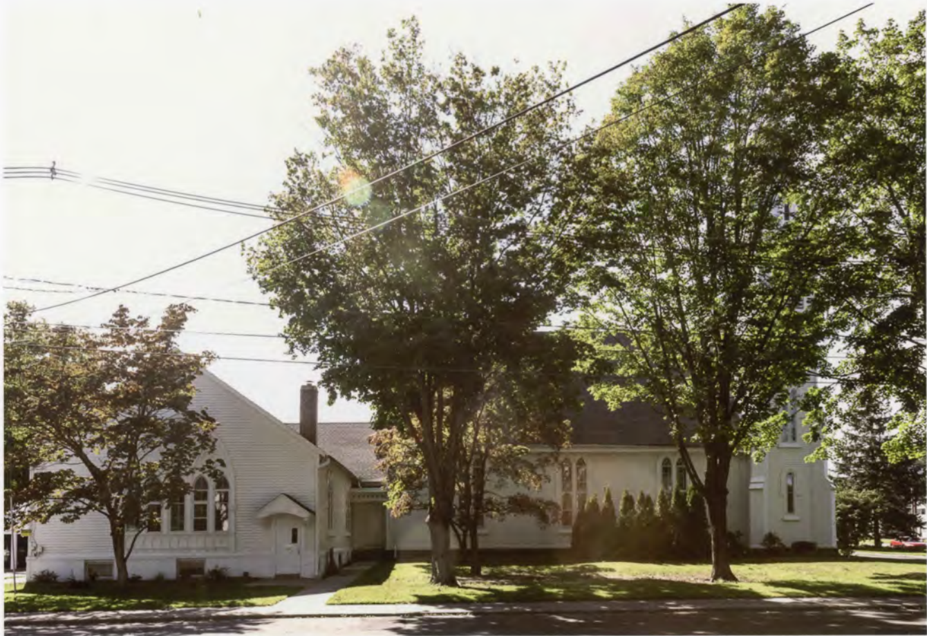
Photo 8. Plainville Congregational Church, Plainville, Hartford County, Connecticut, view west showing east elevation. August 29, 2011, Tod Bryant.
