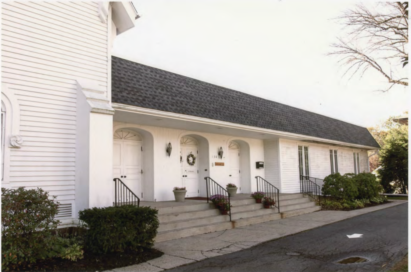
Photo 9. Plainville Congregational Church, Plainville, Hartford County, Connecticut, view southeast, showing facade of new entrance, October 28, 2011, Tod Bryant.
