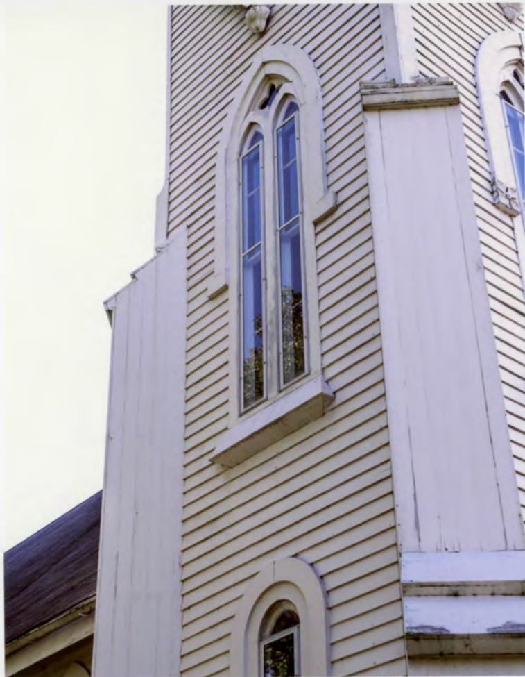
Photo 5. Plainville Congregational Church, Plainville, Hartford County, Connecticut, view southwest, showing tower windows and buttresses. August 29, 2011, Tod Bryant.
