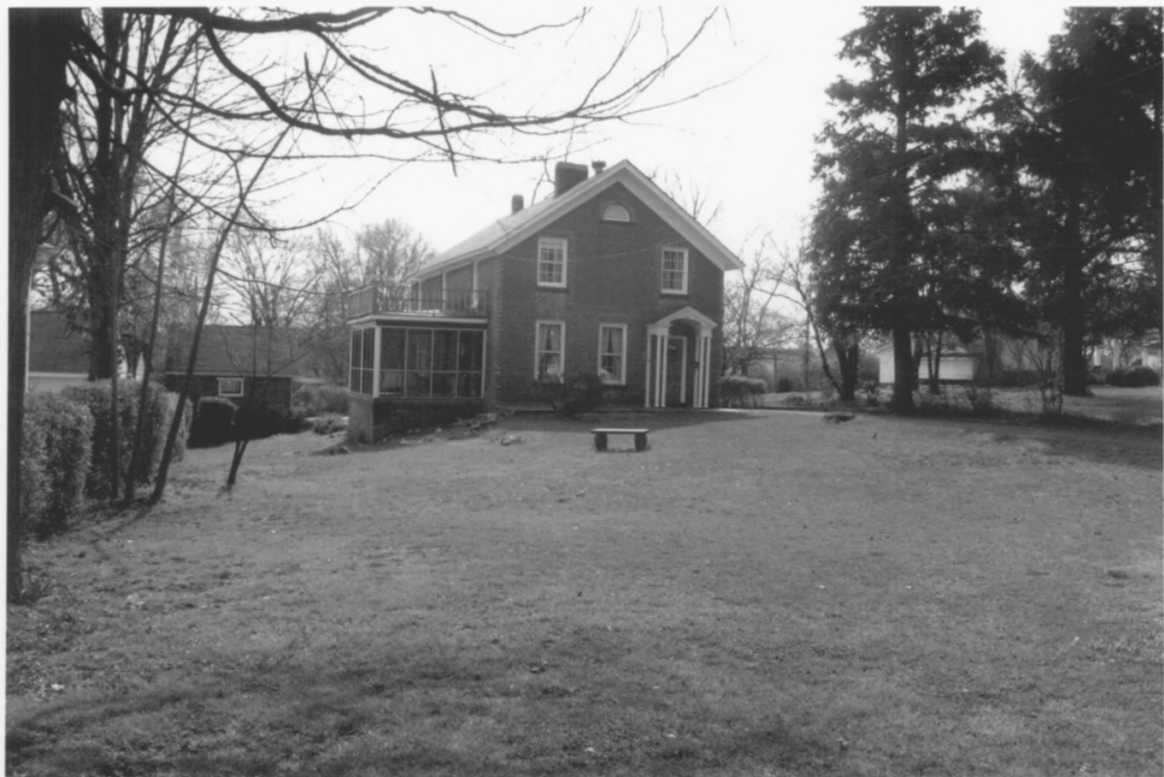
Ocoee Street Historic District Bradley County TN
