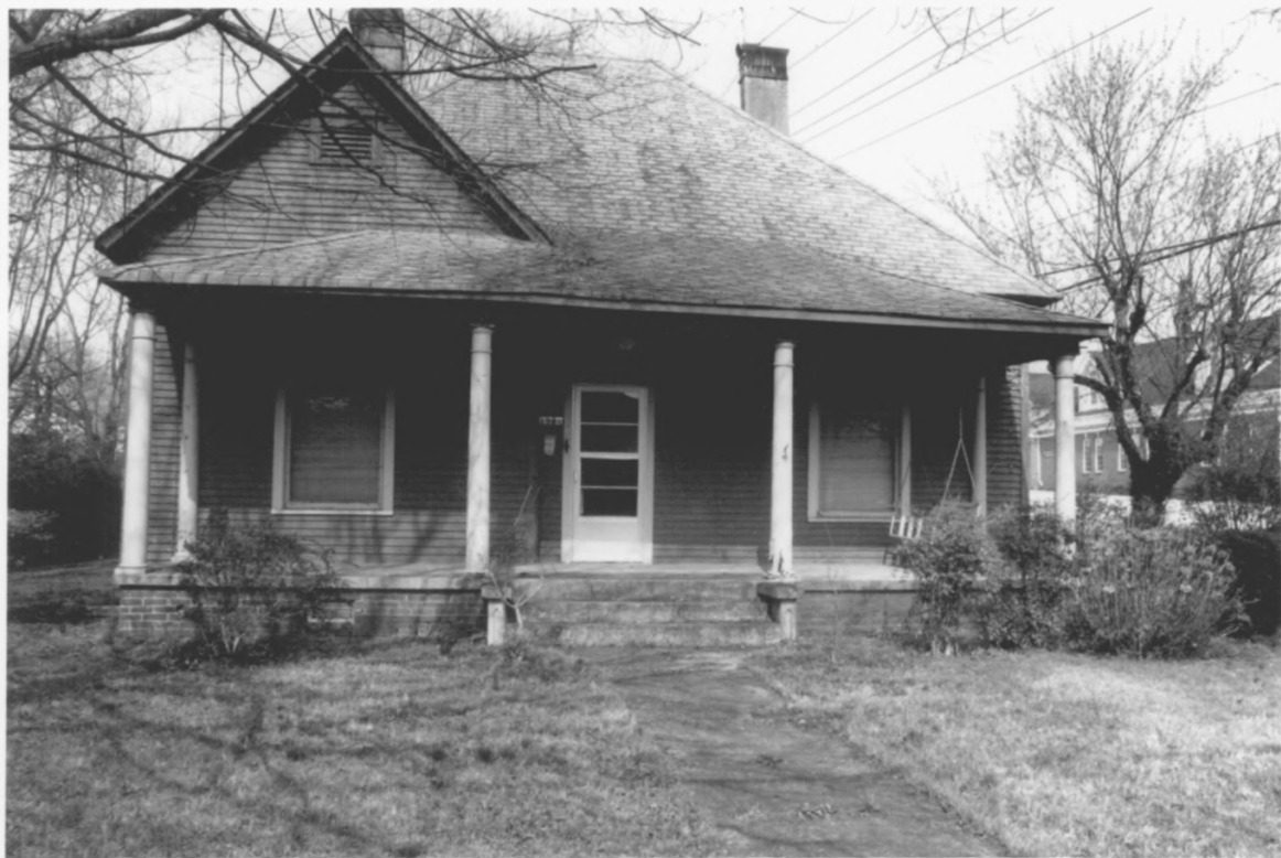
Ocoee Street Historic District Bradley County TN
