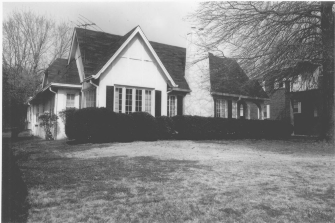
Ocoee Street Historic District Bradley County TN
