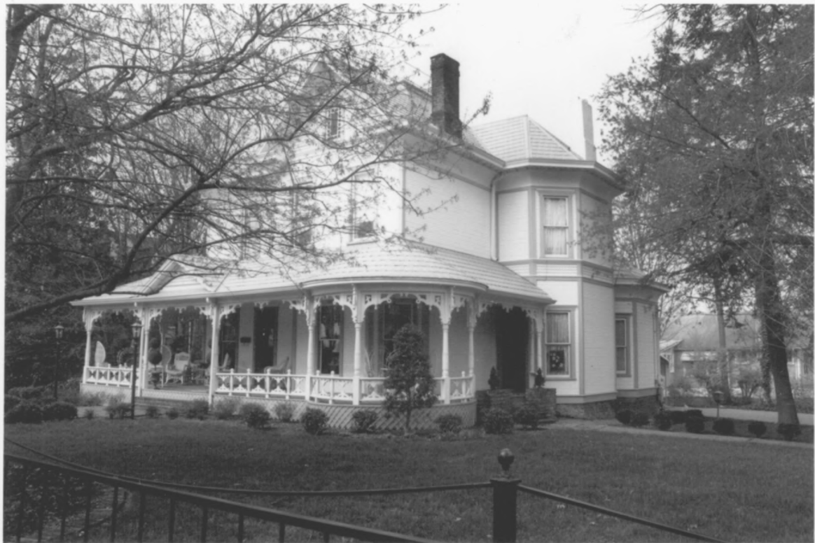
Ocoee Street Historic District Bradley County TN
