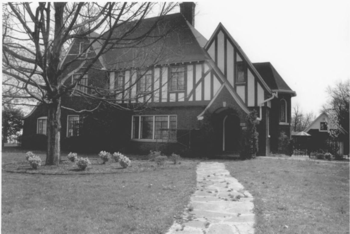
Ocoee Street Historic District Bradley County TN
