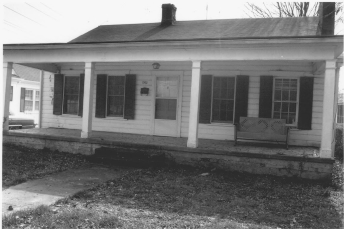
Ocoee Street historic District Bradley County TN
