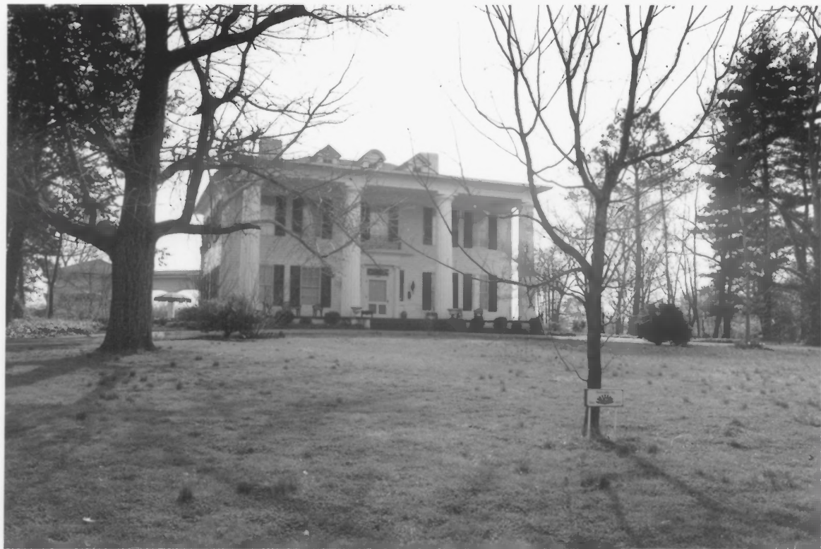
Ocoee Street Historic District Bradley County TN
