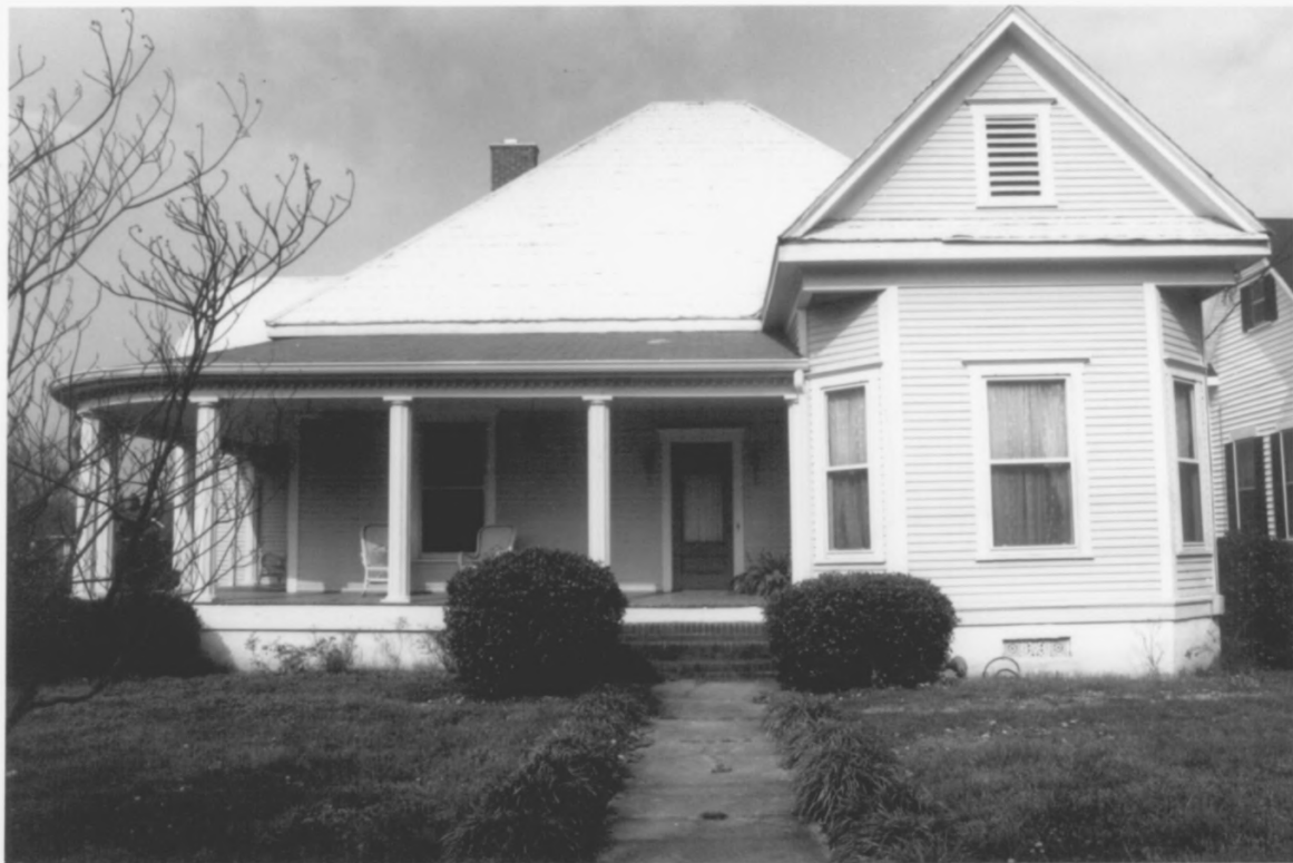
Ocoee Street Historic District Bradley County TN
