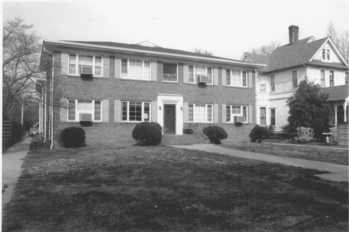
Ocoee Street Historic District Bradley County TN
