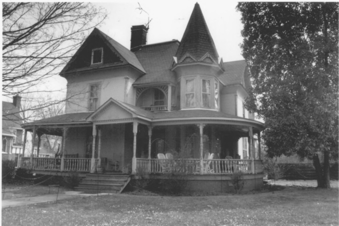
Ocoee Street Historic District Bradley County TN
