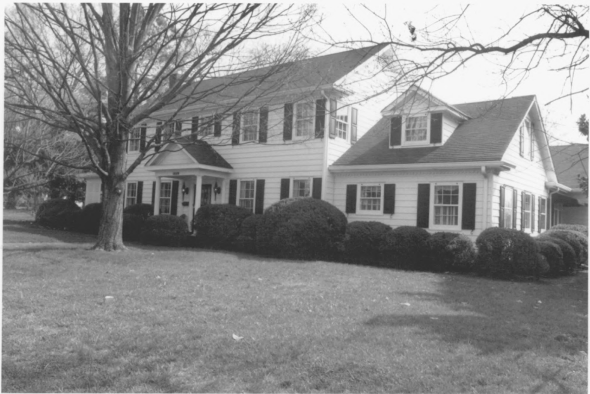
Ocoee Street Historic District Bradley County TN
