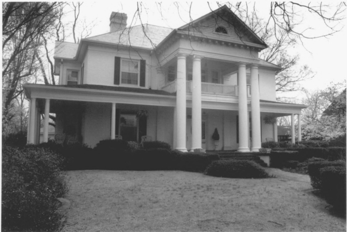
Ocoee Street Historic District Bradley County TN
