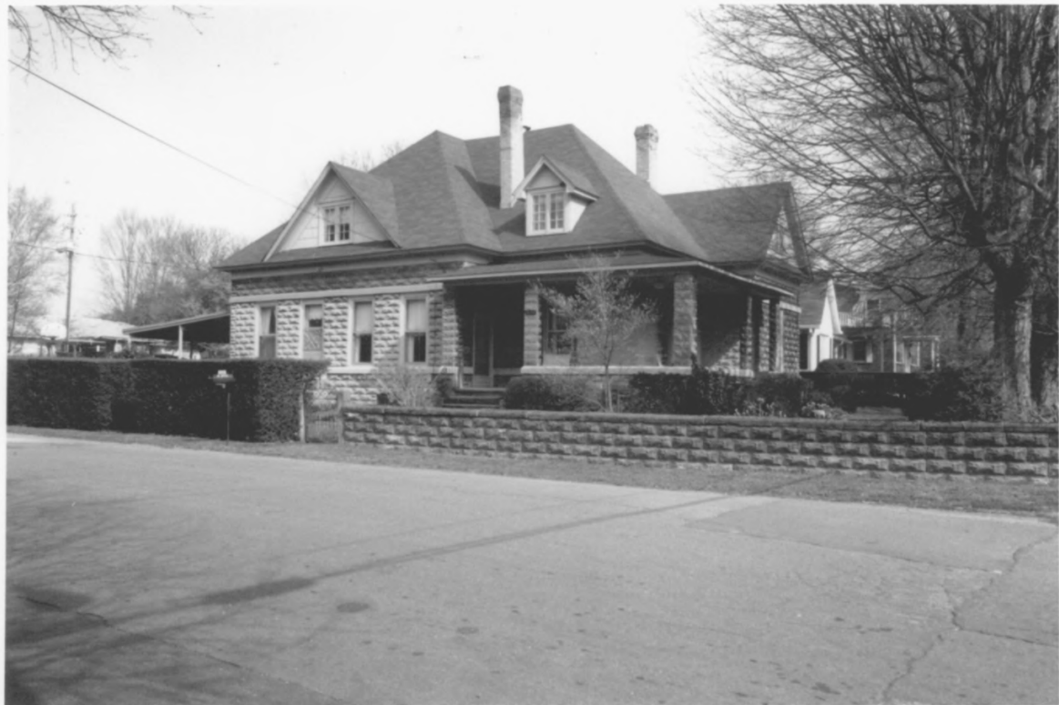
Ocoee Street Historic District Bradley County TN
