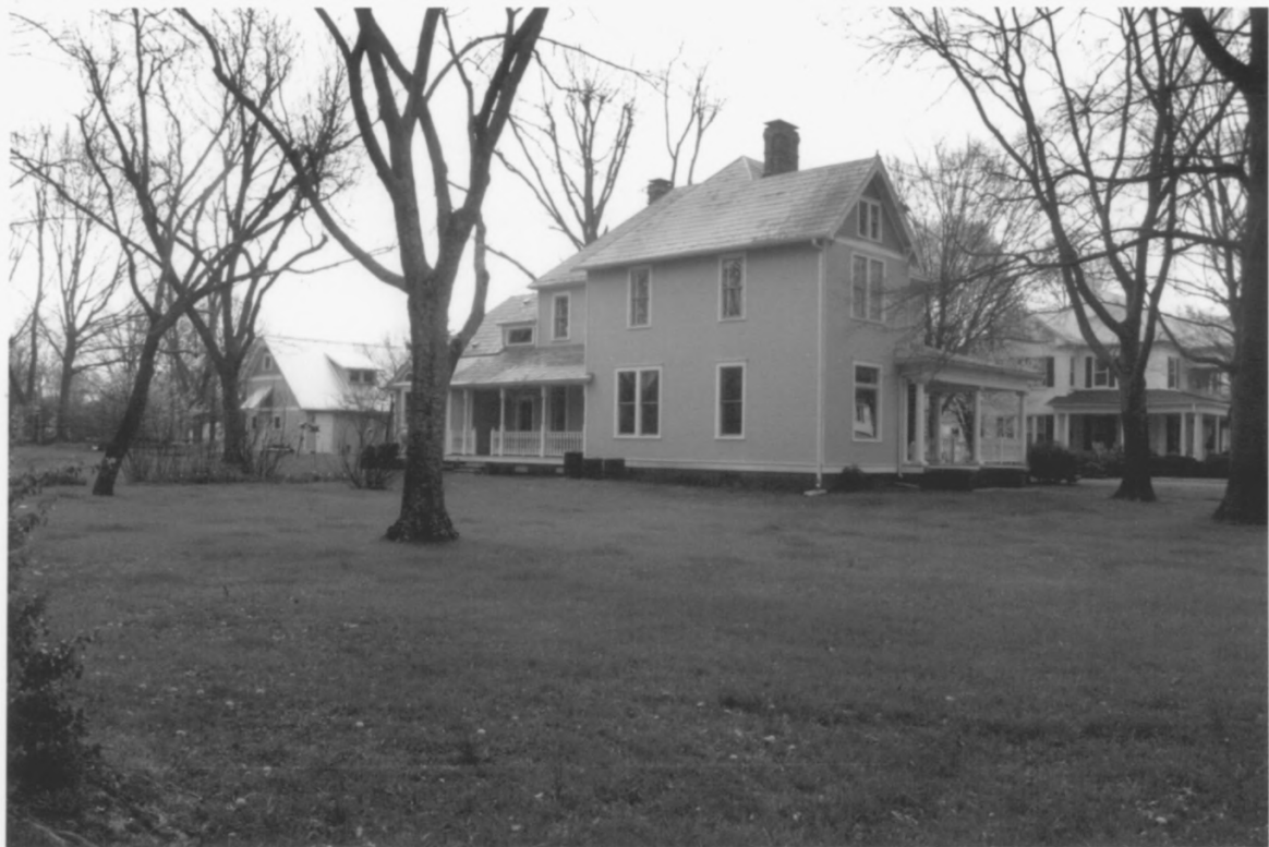
Ocoee Street Historic District Bradley County TN
