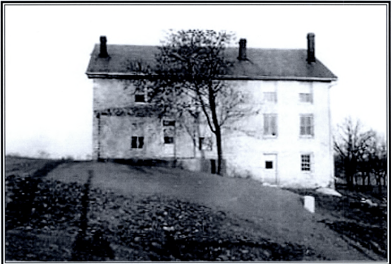
Fig. 1 This undated photo shows the facade (W elevation) of the house associated with the nominated property, with the “ghost” of the front porch clearly visible.
