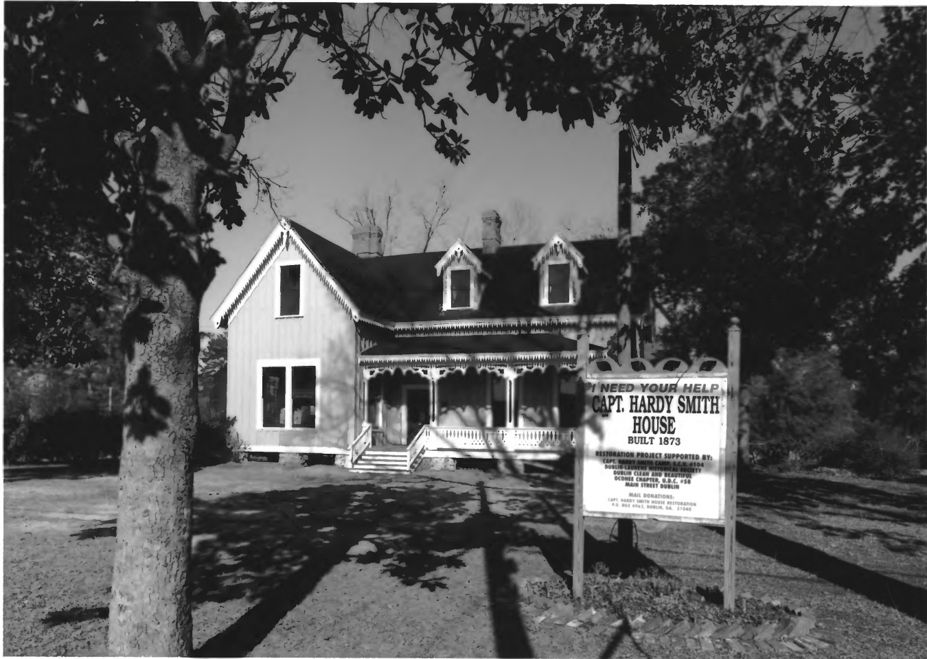
STUBBS PARK-STONEWALL STREET HISTORIC DISTRICT DUBLIN, LAURENS COUNTY, GEORGIA PHOTOGRAPH 29 OF 62
