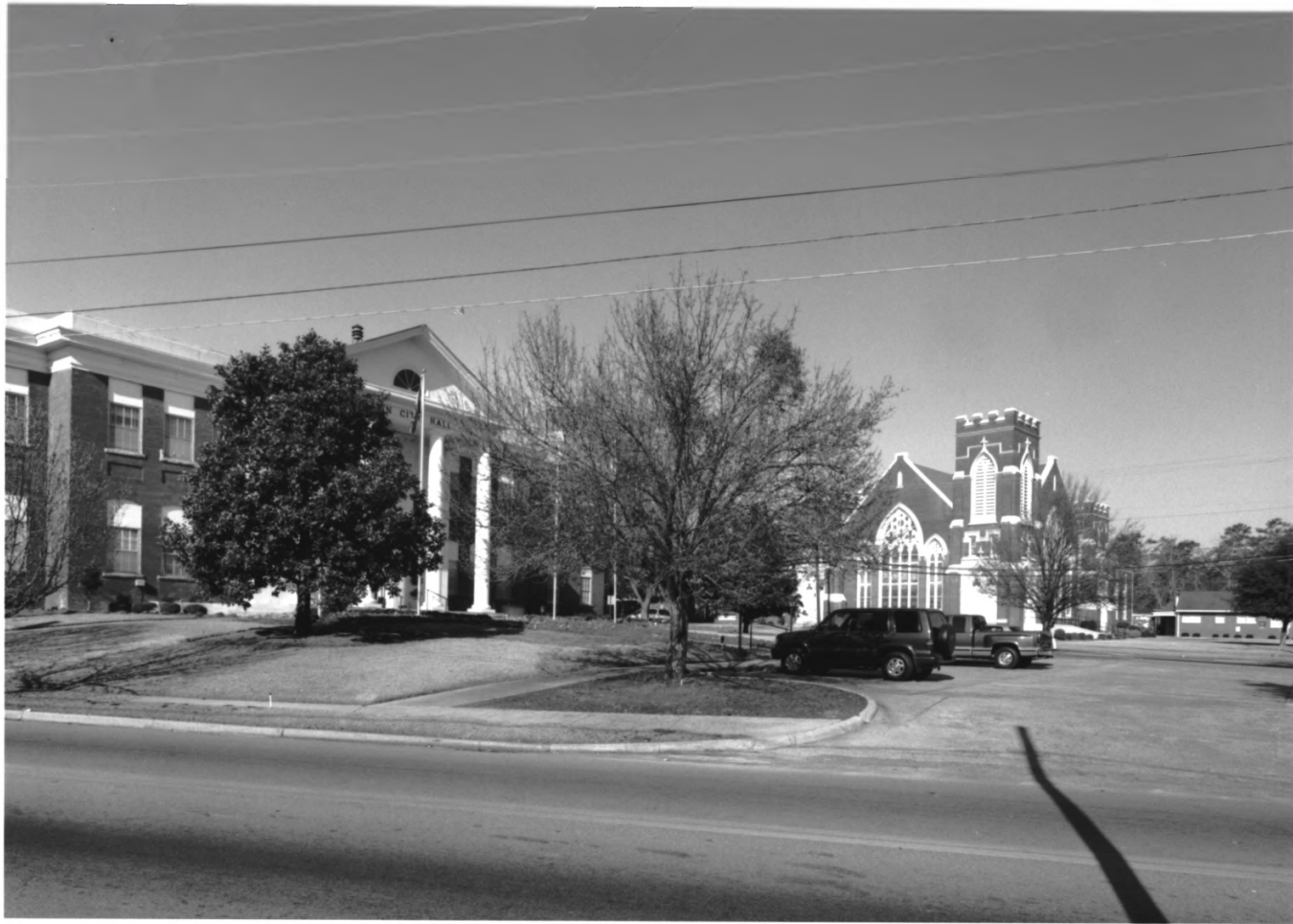
STUBBS PARK-STONEWALL STREET HISTORIC DISTRICT DUBLIN, LAURENS COUNTY, GEORGIA PHOTOGRAPH 31 OF 62
