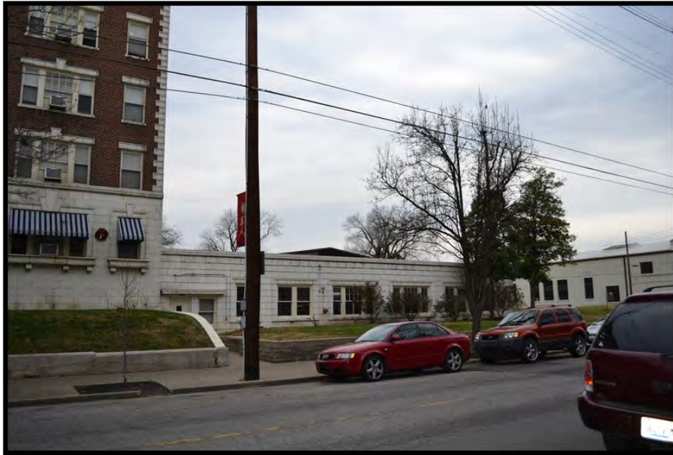
Figure 13. Garage façade, looking northwest from South Fourth Street. (Photo 0012).
