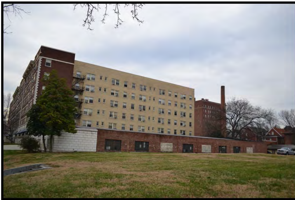
Figure 18. North elevation, looking southwest. (Photo 0018).
