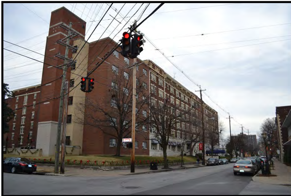
Figure 9. Primary façade, looking northwest from corner of West Ormsby Street. (Photo 0006).
