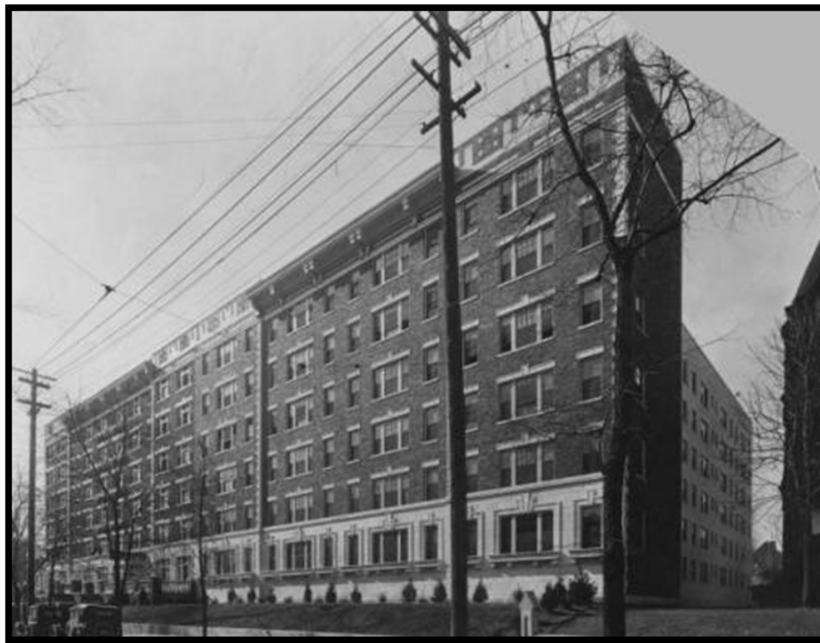
Figure 36. The Puritan Apartments in 1931, photo taken to show the recent annex addition to the building’s north elevation and primary façade. 75
