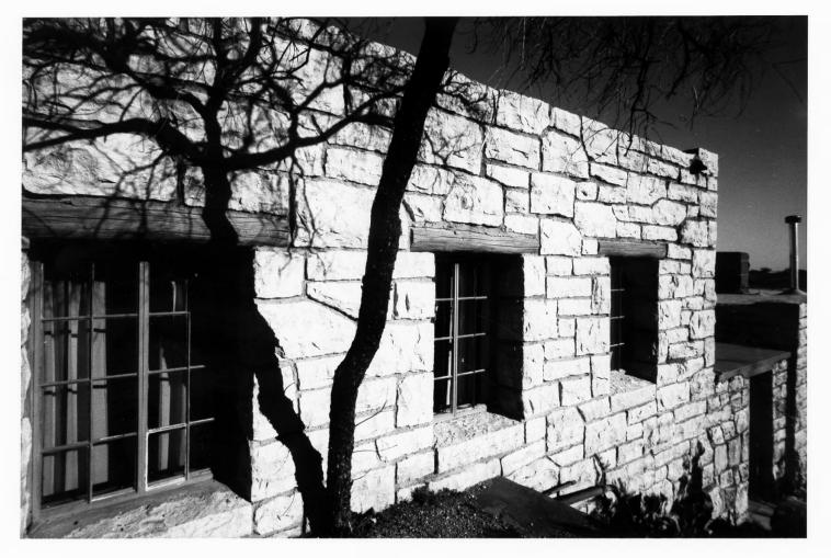
1. Bunk House and Mess Hall, NPS Bldg #16. West side, rough-cut limestone walls, steel casement windows, halved log lintels. (Sig.)
