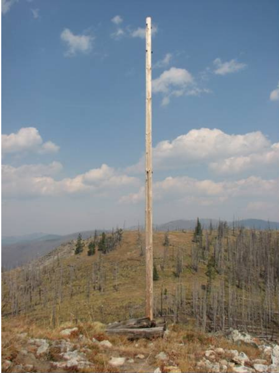
MT_RavalliCounty_GirdPointLookout_0011. Looking northeast to the communications pole.
