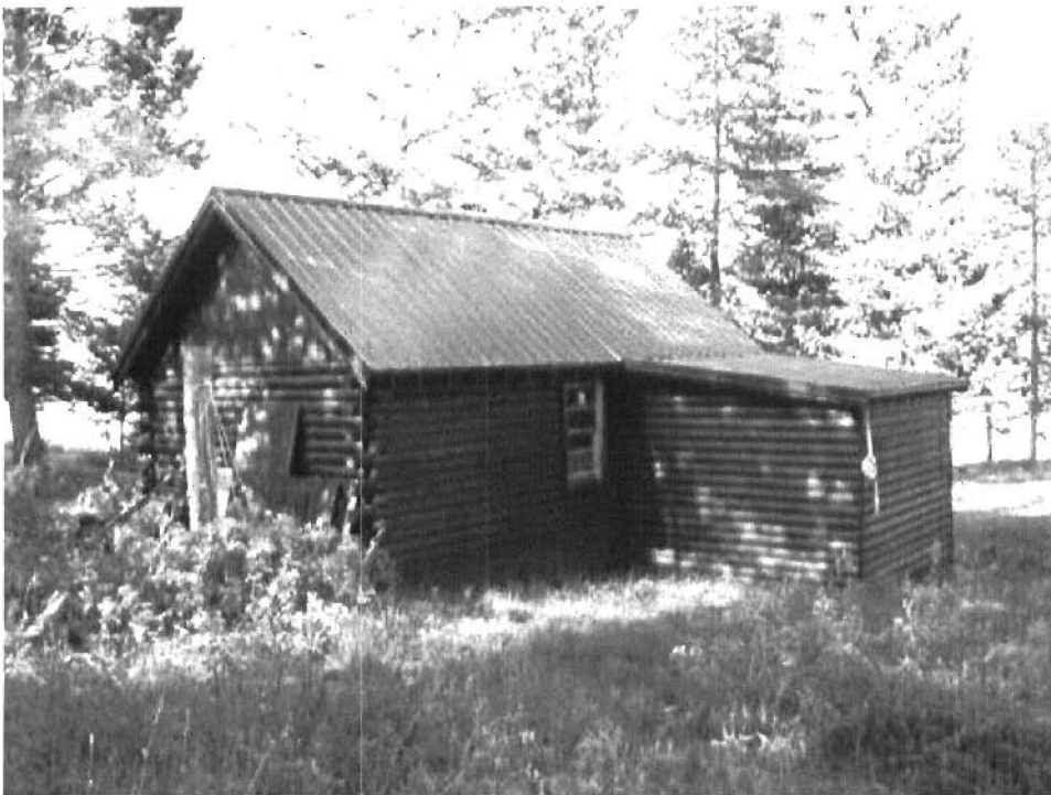
MT_GallatinCo_LonesomehurstCabin_0008 of 0014. South and west sides of boathouse, view to northeast
