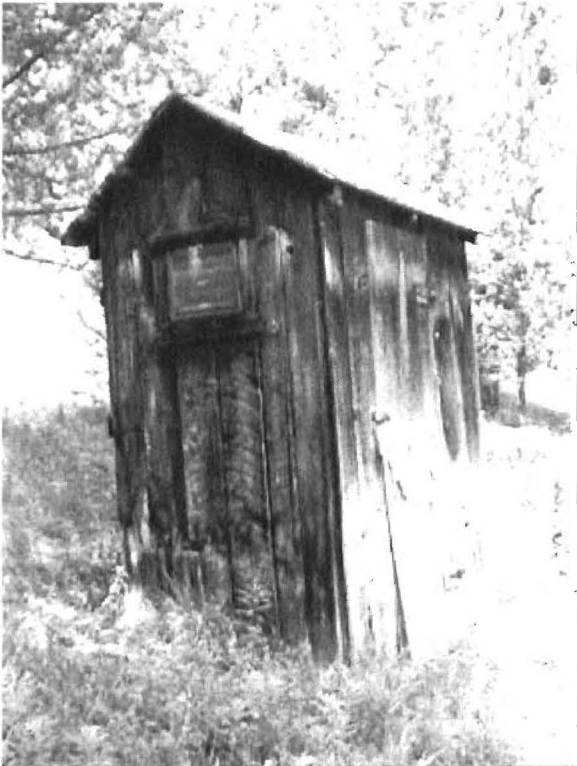
MT_GallatinCo_LonesomehurstCabin_0006 of 0014. South and east side of outhouse, view to north
