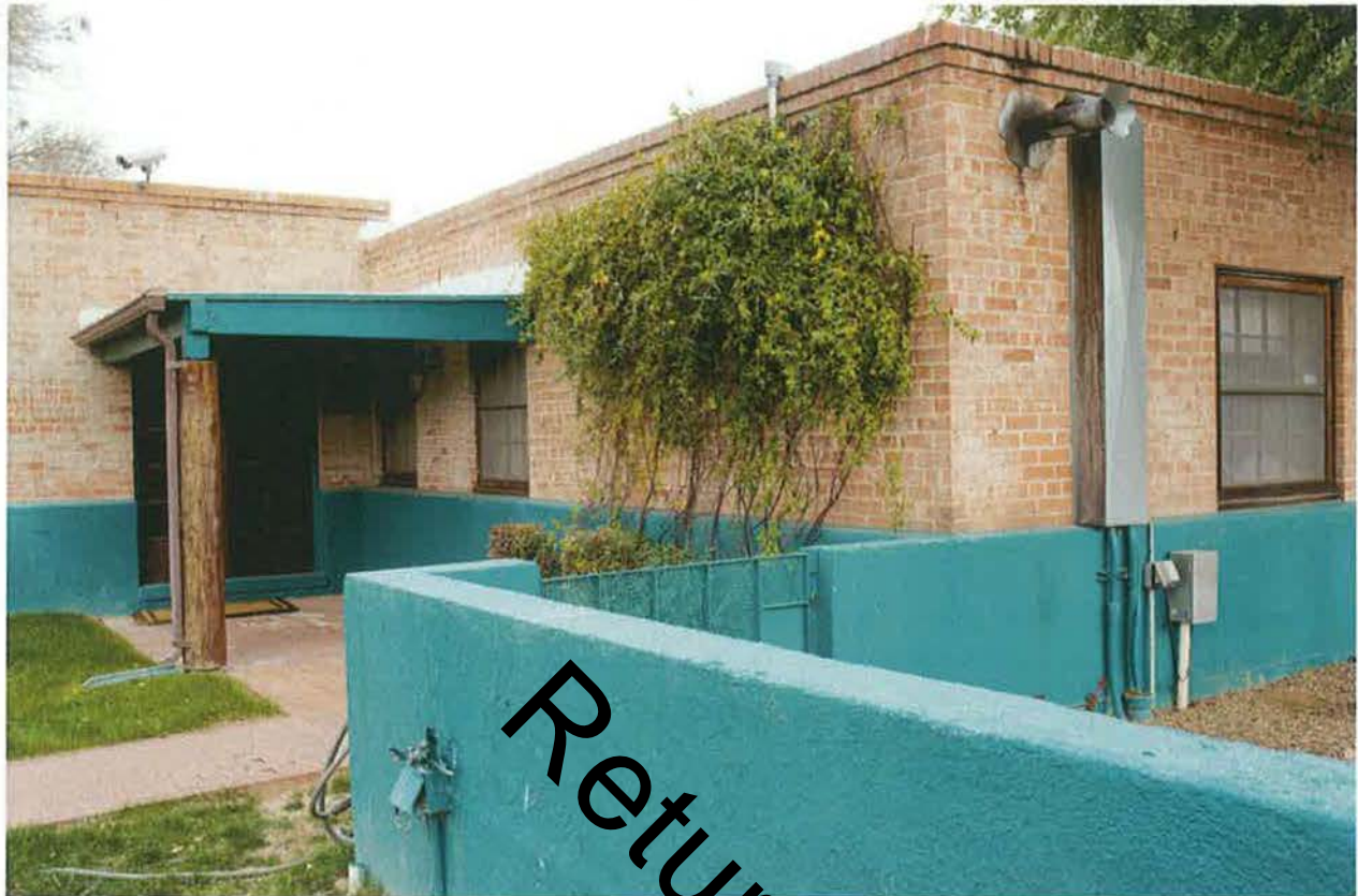
Photograph 7. Detail of wall and gate around courtyard southwest corner (A.T.Willett 2017) (AZ_PimaCounty_WoodrowResidence_0007).
