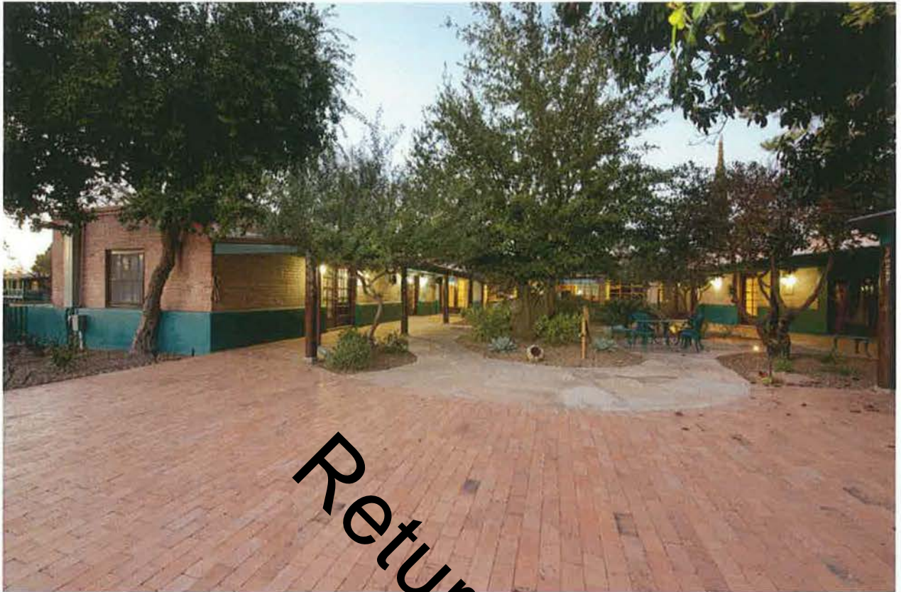
Photograph 5: South elevation of the Woodrow Residence, view facing north-northwest (A.T.Willett 2017) (AZ_PimaCounty_WoodrowResidence_0005).
