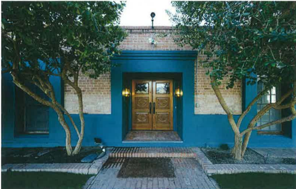
Photograph 2: Detail of north elevation of the Woodrow Residence, view facing south (A.T.Willett 2017) (AZPimaCounty_WoodrowResidence_002).
