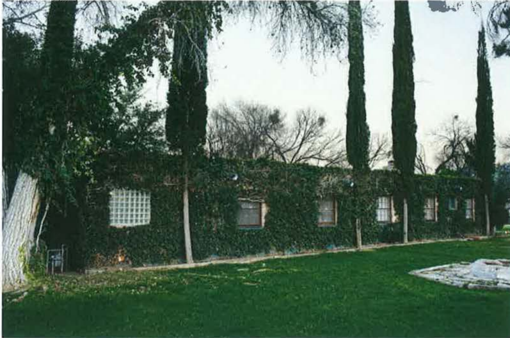
Photograph 4: East elevation of the Woodrow Residence, view facing west (A.T.Willett 2017)(AZPimaCounty_WoodrowResidence_004).
