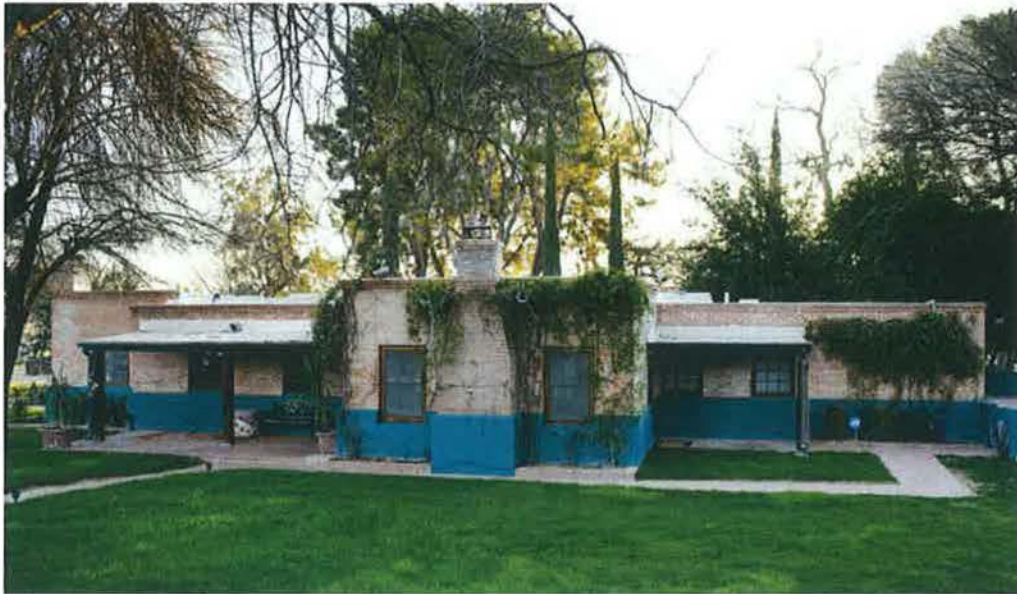
Photograph 3: West elevation of the Woodrow Residence, view facing east (A.T.Willett 2017)(AZPimaCounty_WoodrowResidence_003).
