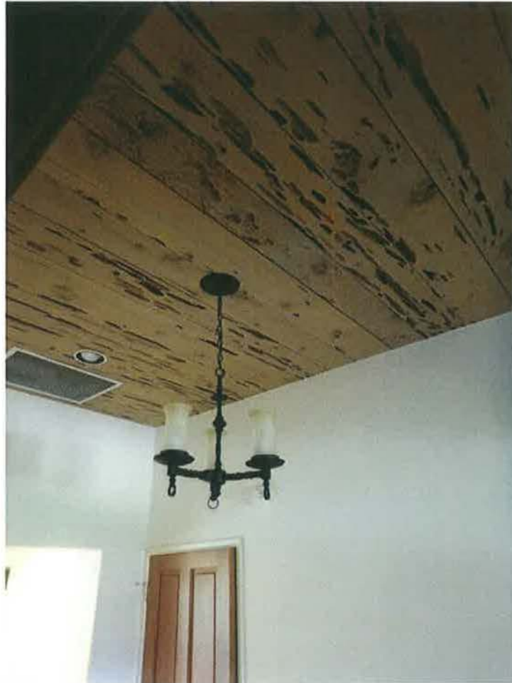
Photograph 10. Detail of pecky cedar ceilings (J. Levstik 2017) (AZPimaCounty_WoodrowResidence_010).
