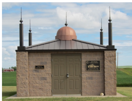
Exterior and interior views of the new structure
