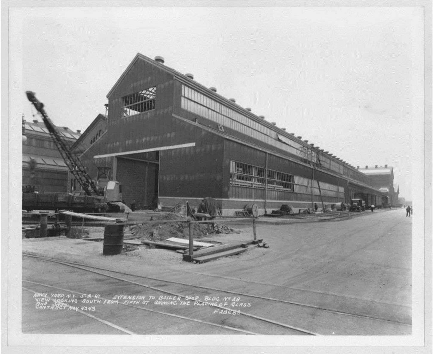
19. 1941 view southwest on Fifth Street showing the 1940-41 addition to Building 28 (boiler shop, ca. 1895, first addition 1900). This addition connected Buildings 28 and 128 with Building 123 (power house, 1900), a gable-roofed brick structure partially shown at left. ( Brooklyn Navy Yard Archives )
