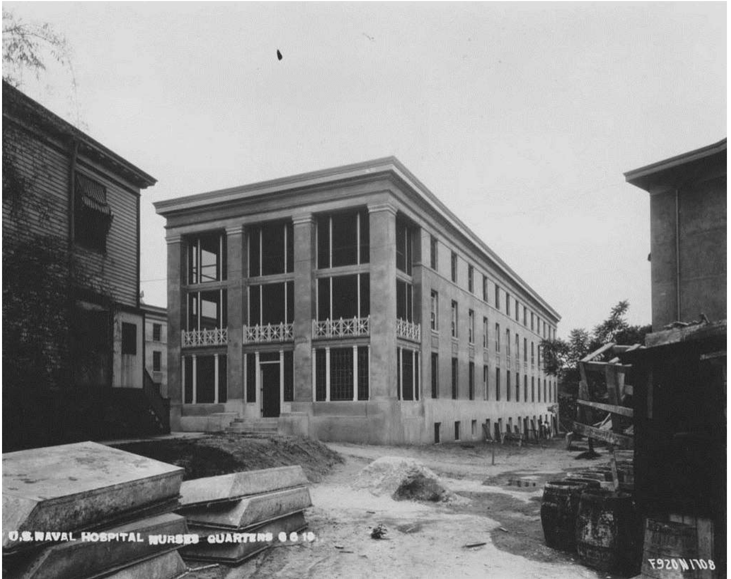
27. 1919 view of the east wing of Building RG (nurses quarters, 1919). The building provided housing for approximately 130 nurses, all part of the Nurse Corps, which was founded in 1908. ( Brooklyn Navy Yard Archives )
