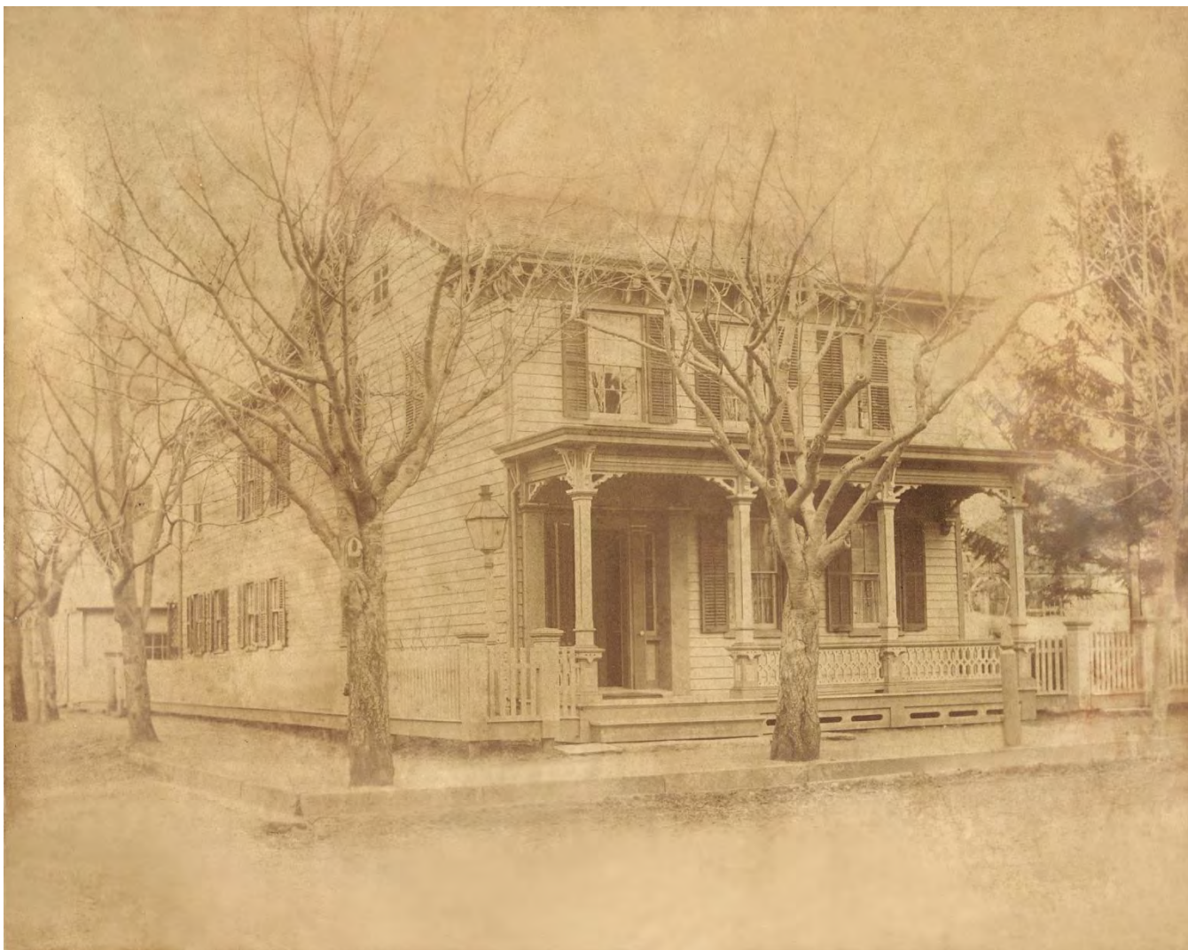
Historic photograph, ca. 1890, front (south) & west facades, view facing northeast. Collection of Walter Foote.
