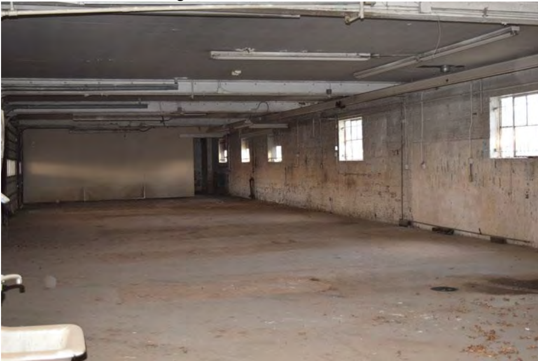
Photo 12: Service area. Camera facing east.
