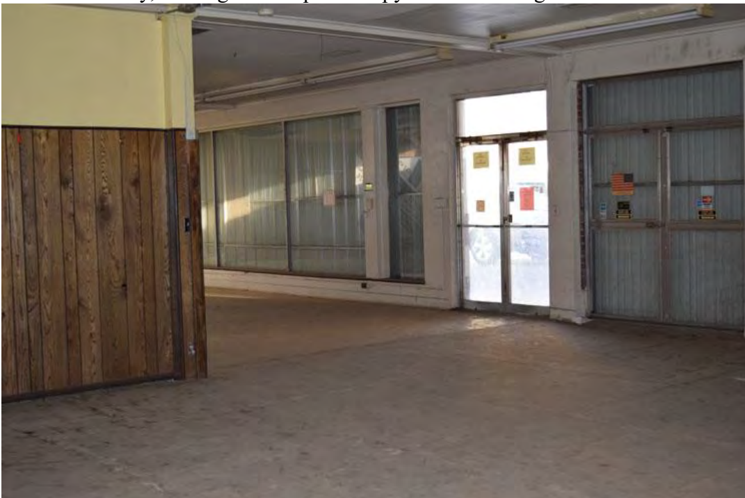
Photo 10: Showroom entry, looking out to open canopy. Camera facing northwest.
