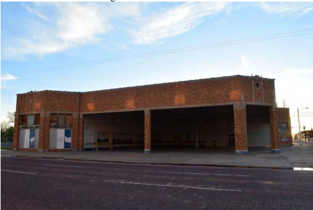
Photo 4: East elevation. Camera facing west.
