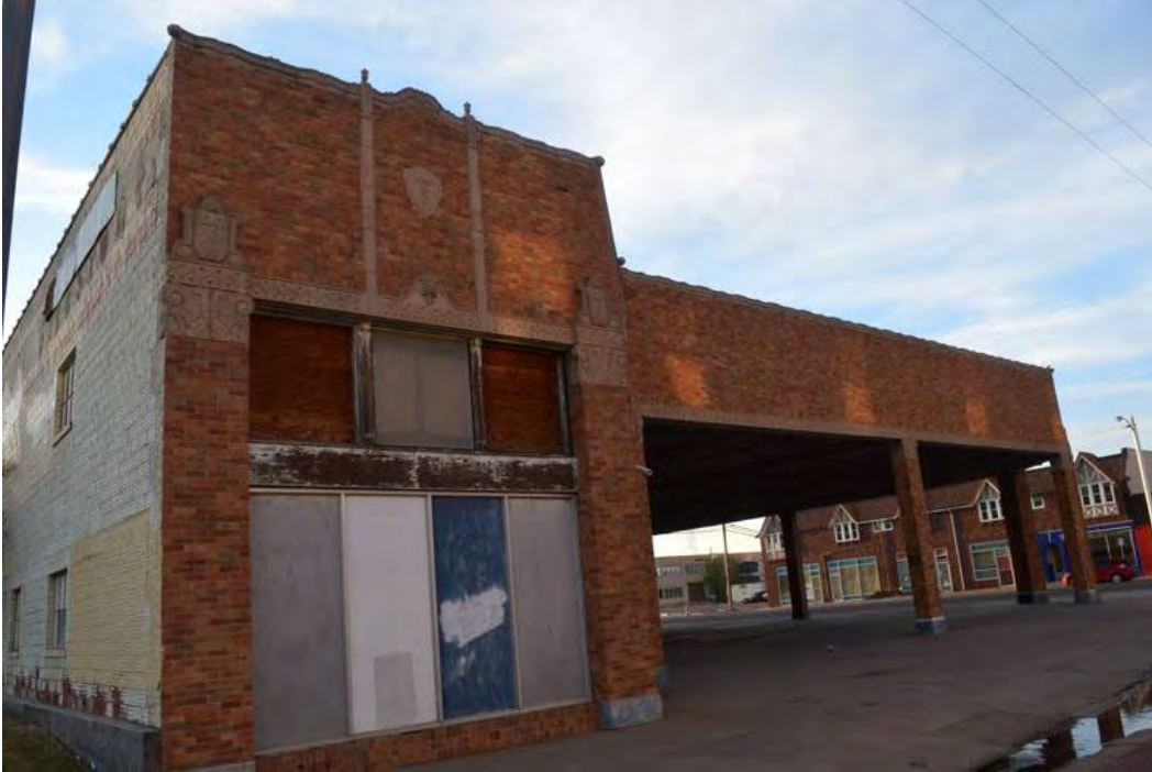
Photo 5: Detail of east elevation. Camera facing northwest.
