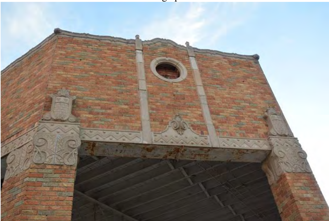
Photo 6: Detail of northeast corner. Camera facing up and to the west.
