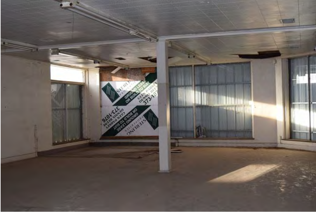
Photo 13: Showroom on northwest corner of building. Camera facing north.
