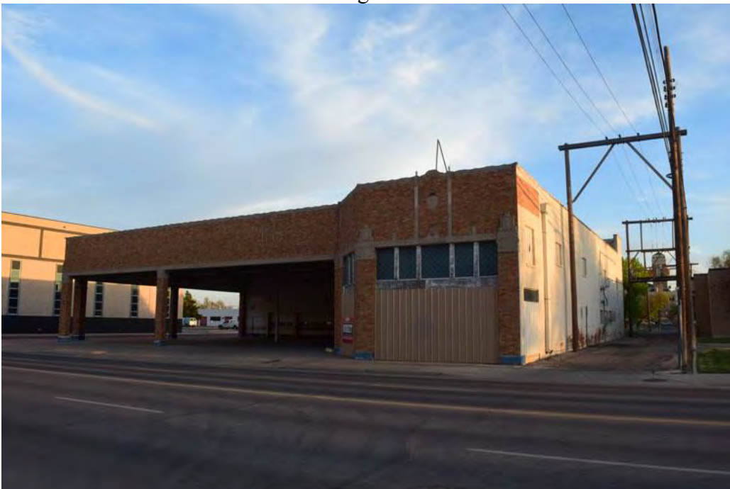
Photo 2: North elevation. Camera facing southwest.
