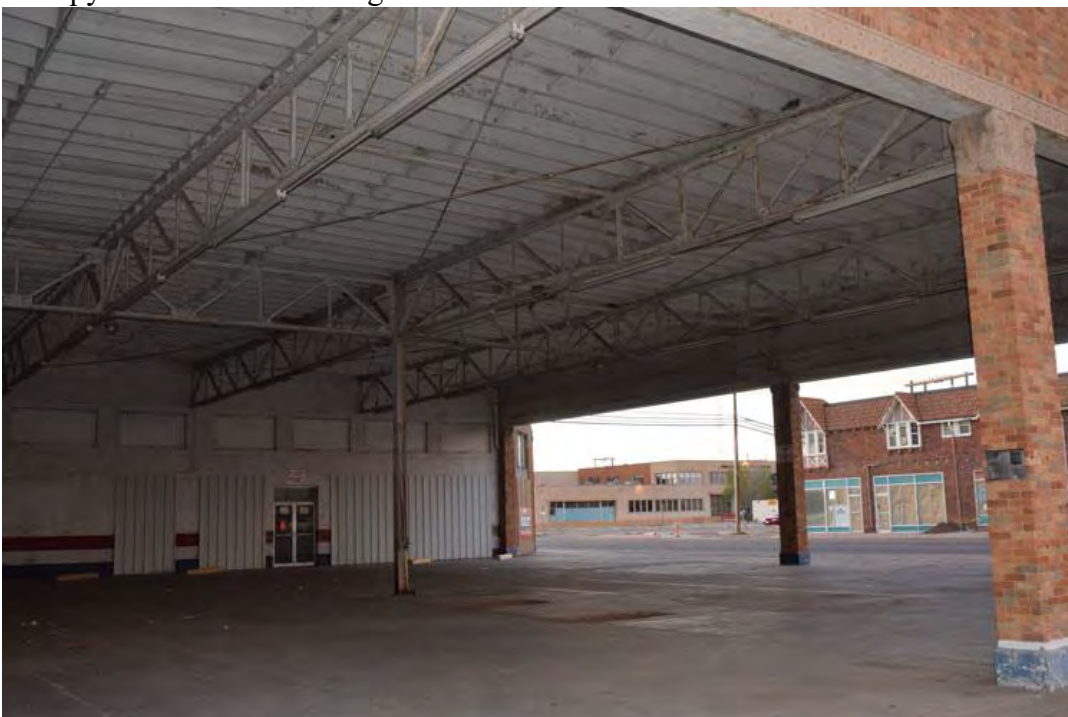
Photo 8: Canopy detail. Camera facing northwest.
