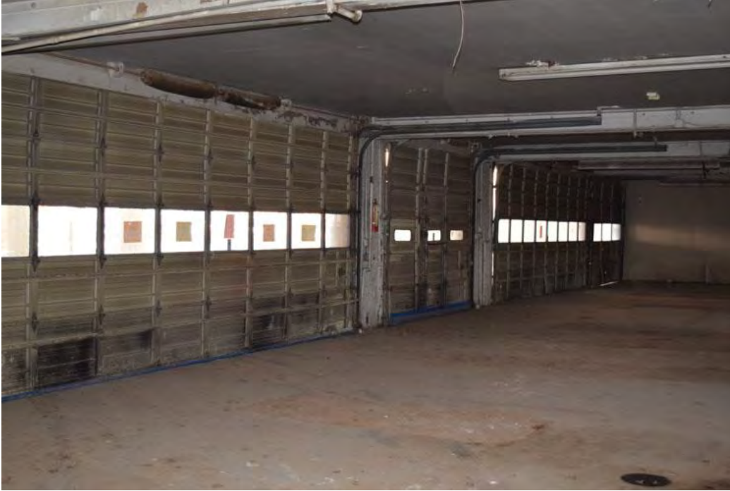
Photo 11: Service area doors. Camera facing northeast.
