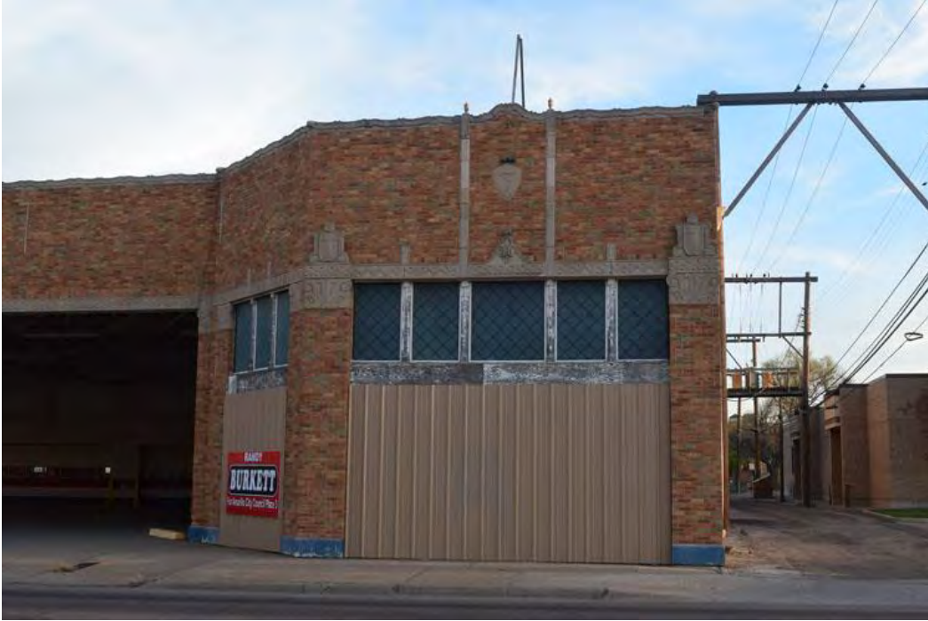
Photo 3: Detail of north elevation. Camera facing south.
