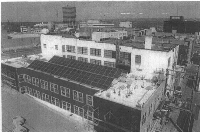
2005 photo looking north from neighboring building onto Acme Building roof and south sidewall.
