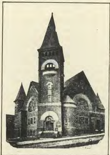
Union Square Baptist Church STREET
