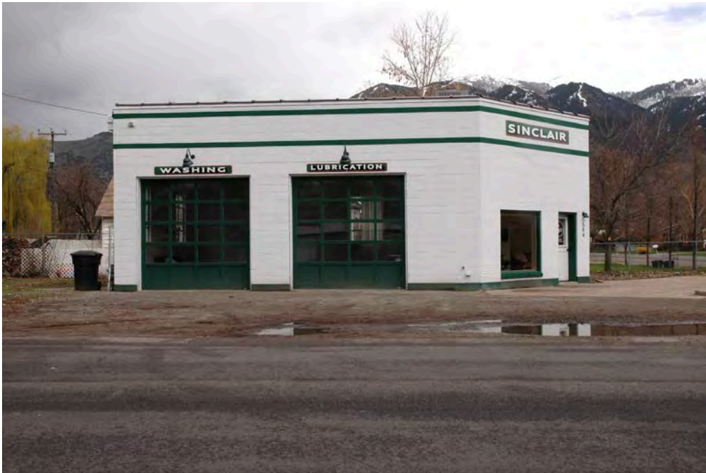
Photograph 2 West elevations of River Heights Sinclair Station. Camera facing east.
