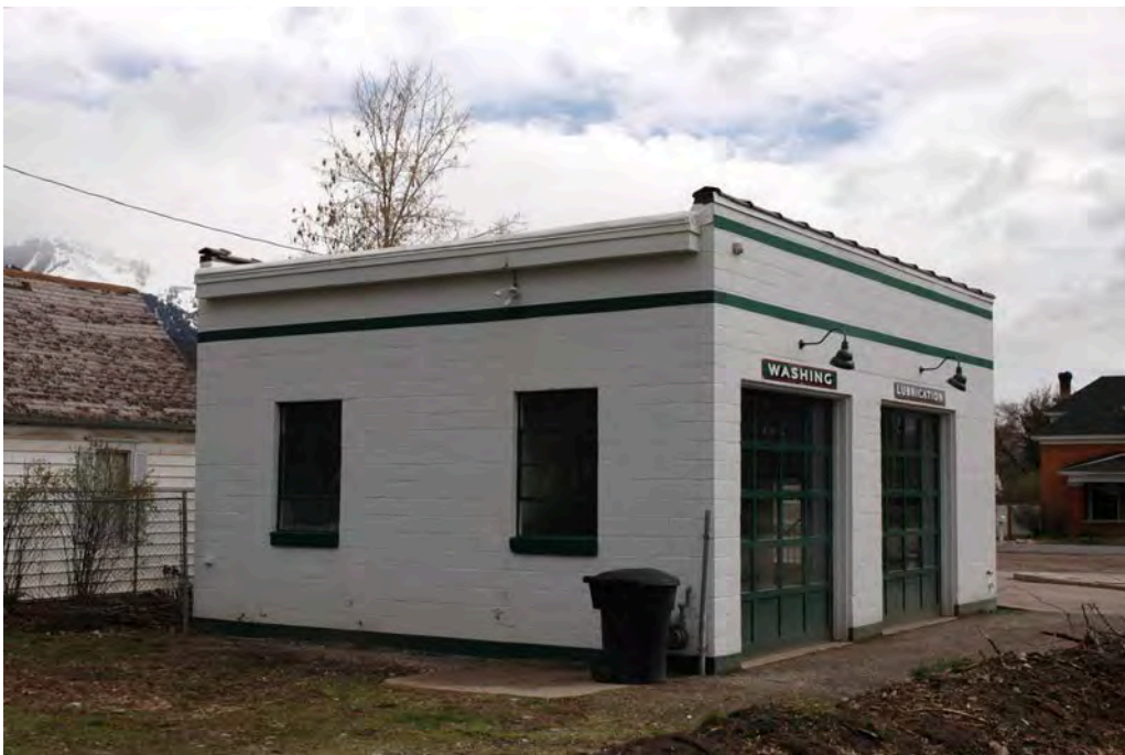
Photograph 3 North and west elevations of River Heights Sinclair Station. Camera facing south.
