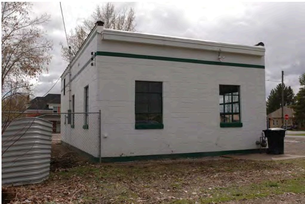
Photograph 5 North and east elevations of the River Heights Sinclair Station. Camera facing southwest.
