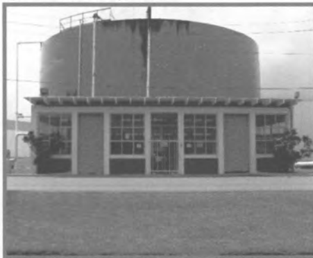
Fig. 41 Water Pump House
