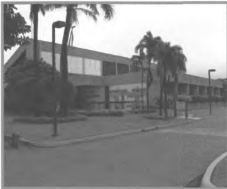
Fig. 37 Executive Offices Building
