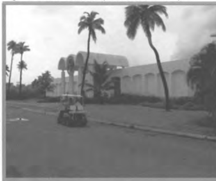
Fig. 11 Visitor Center (Warehouse # 7)
