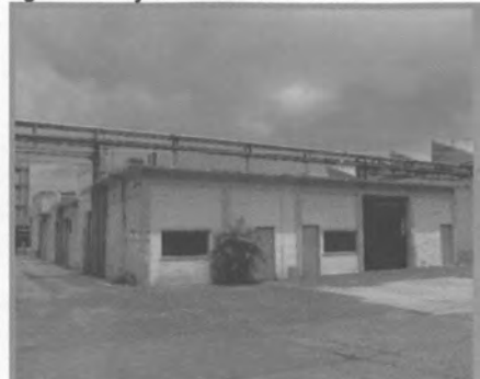
Fig. 35 Safety & Construction Office
