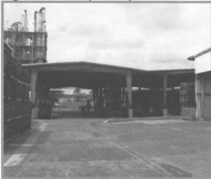
Fig. 31 Barrels Repair Shop
