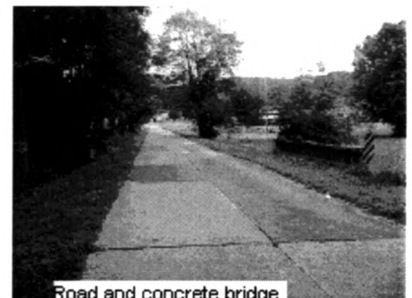
Road and concrete bridge
