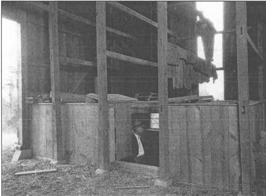
Figure 11. Example of a semi-subterranean stripping room
