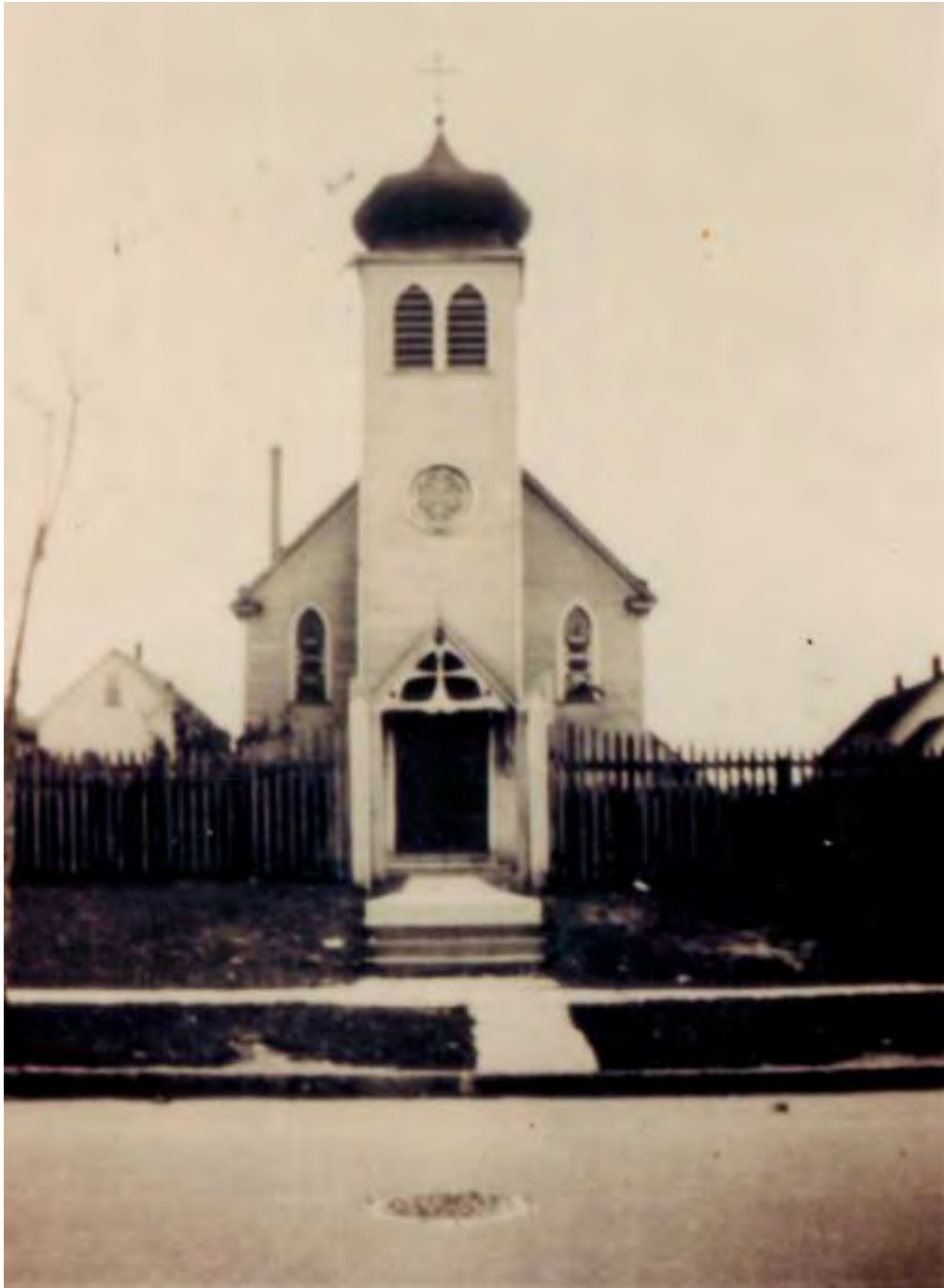
View of the old church, showing bell tower addition (ca. 1906-1917)
