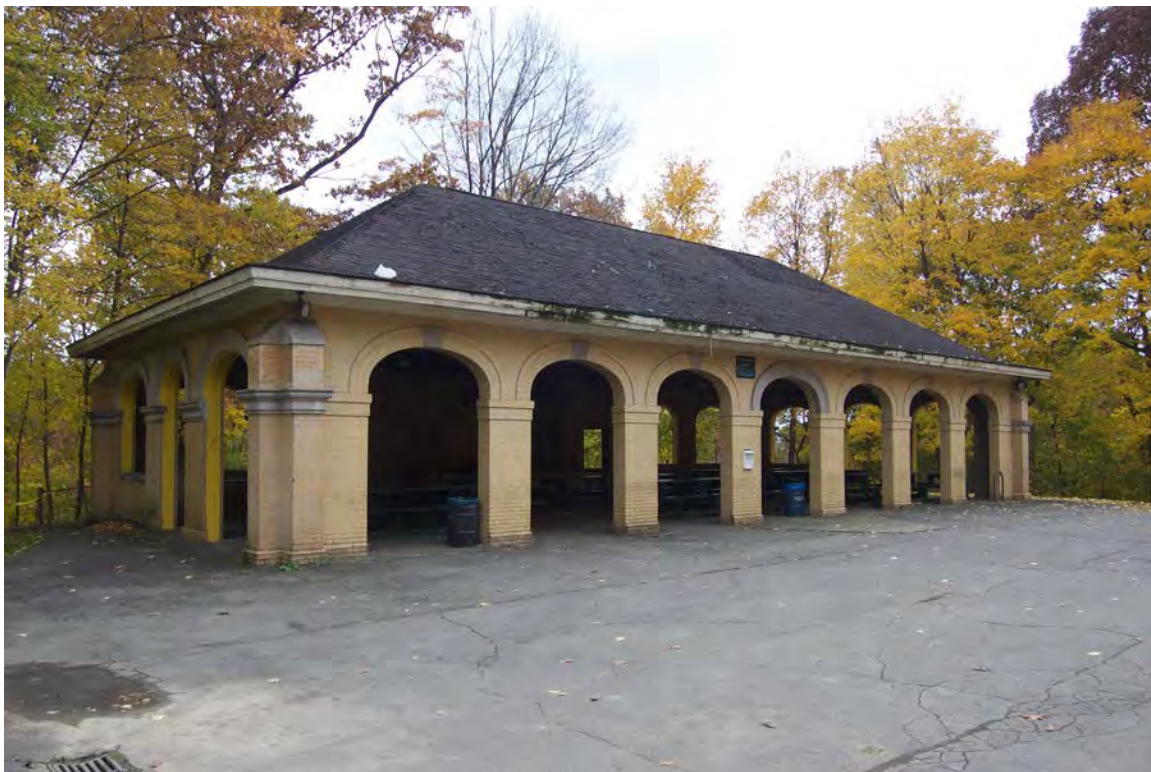
Photo 17. Rhododendron Shelter (1902), Lake Drive
