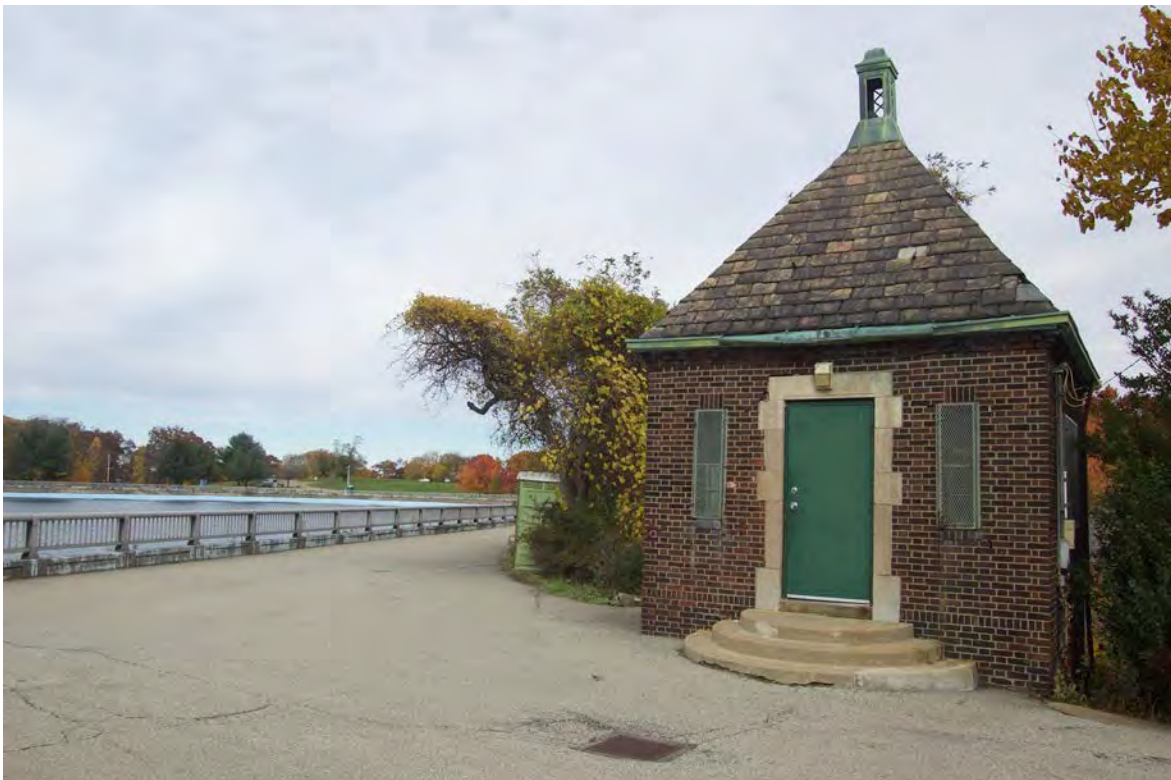
Photo 26. Reservoir service building, Reservoir No. 1
