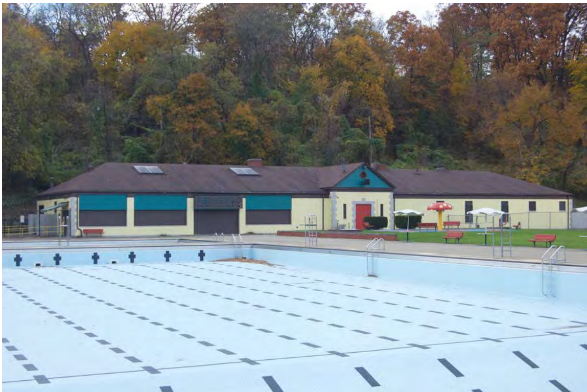
Photo 30. Pool house (1932; remodeled), Lake Drive
