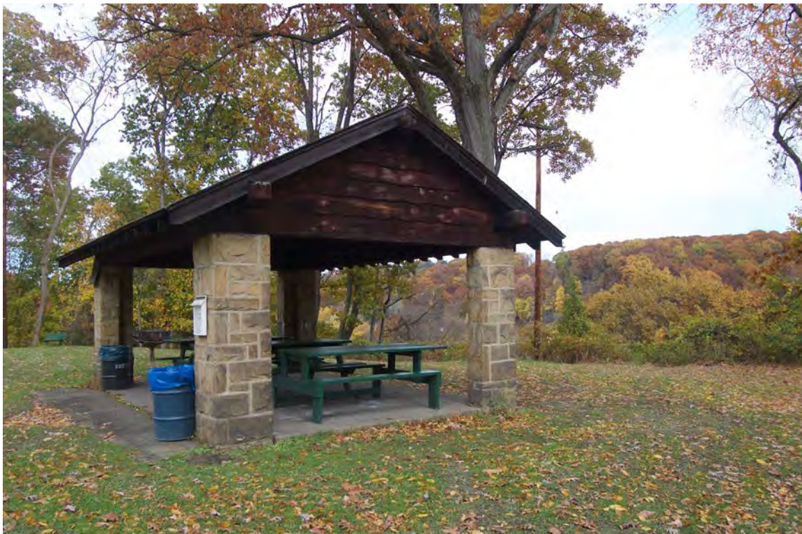
Photo 16. Elm Grove Shelter, Lake Drive
