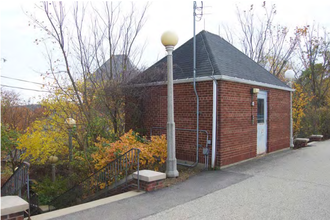
Photo 27. Reservoir service building, Reservoir No. 1
