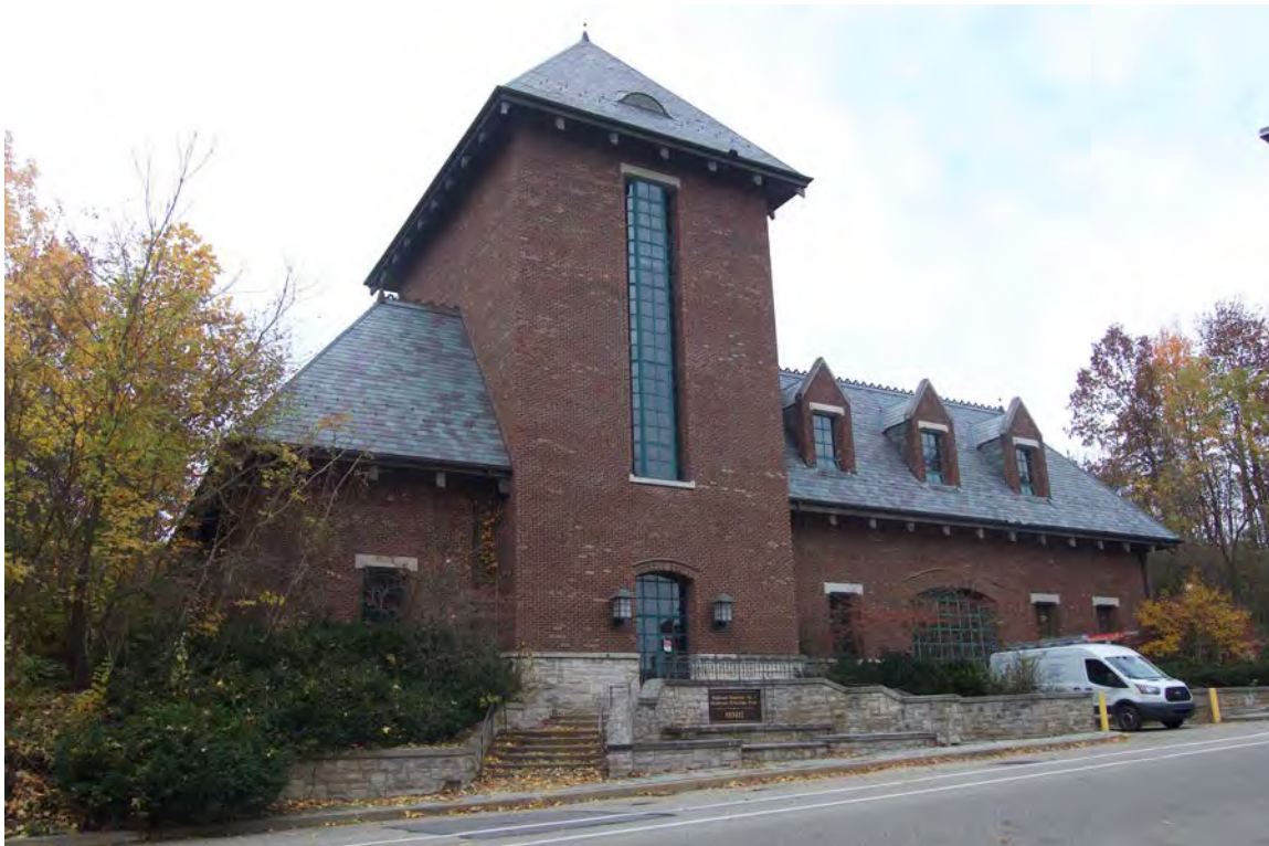
Photo 29. Microfiltration plant, Reservoir Drive
