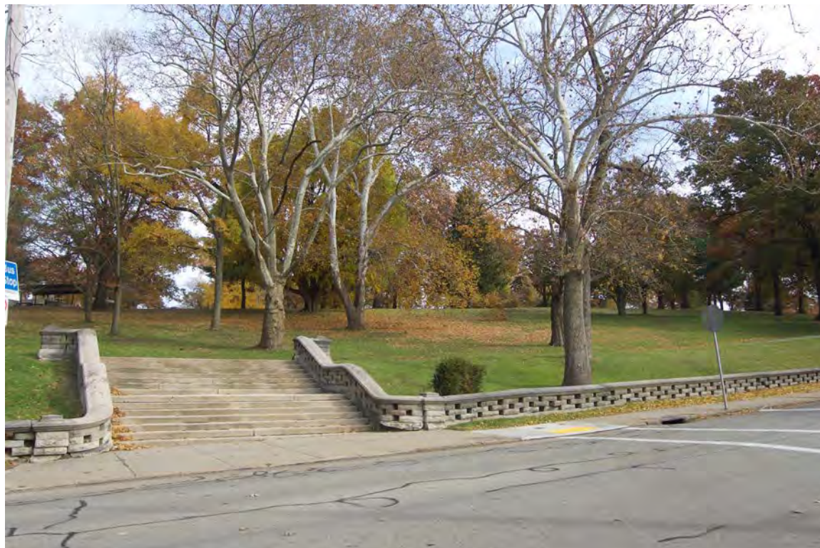
Photo 40. Stone wall and steps, Bunker Hill St.
