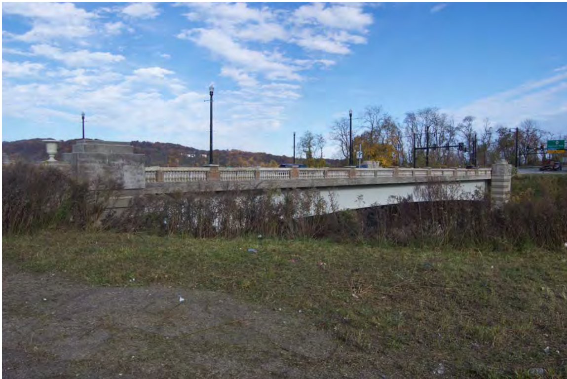
Photo 37. Heth's Run Bridge carries Butler Street over the Heth's Run ravine
