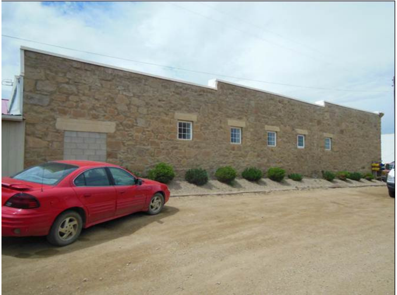
MT_FergusCounty_Stafford'sGrocery_0005. East wall. View looking north-northwest
