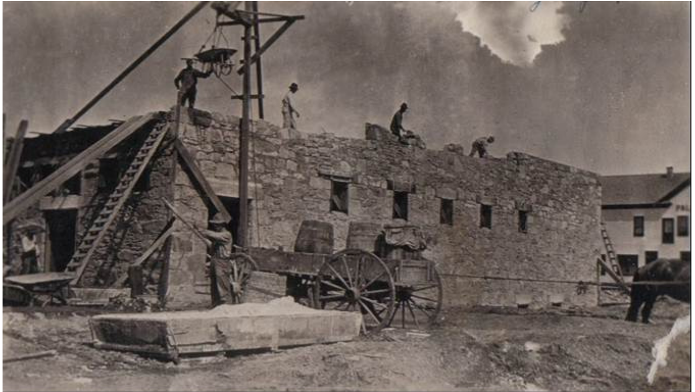
Construction of Stafford's Grocery Store, circa 1914.
