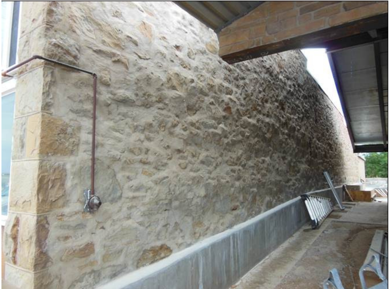
MT_FergusCounty_Stafford'sGrocery_0012. West Wall. View to the south-southeast
