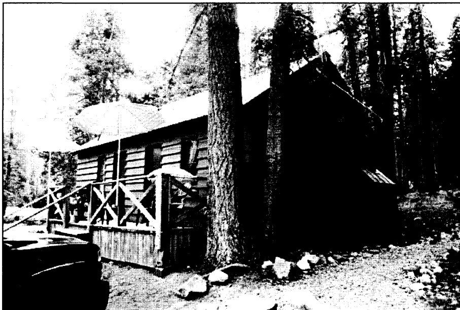
Manager's cabin (contributing), east and north elevations, view to southwest.
