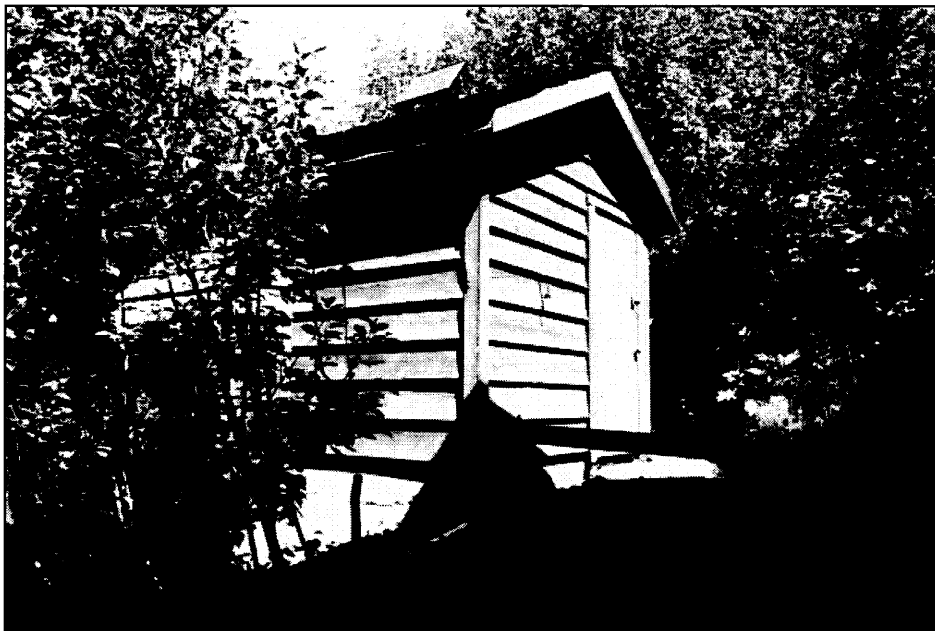
Chlorination building (noncontributing), south and east elevations, view to northwest.
