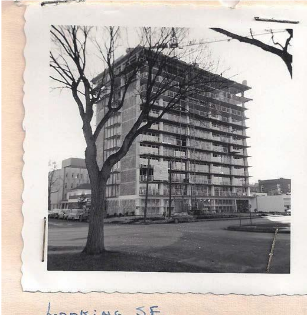
Figure 7: Building under construction looking southeast, c. 1962. (Sky Park Manor Collection)
