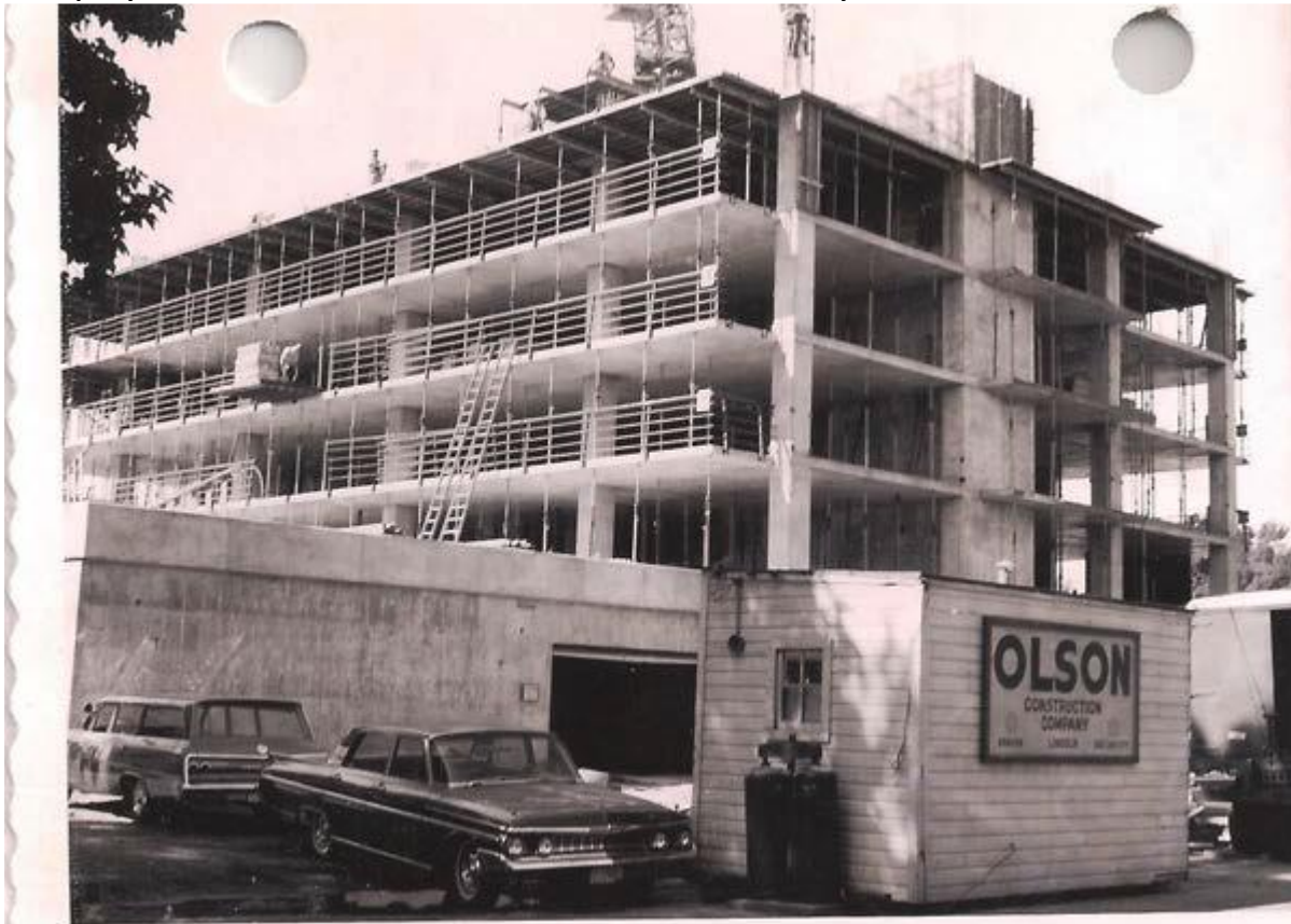
Figure 6: Building under construction looking northeast, c. 1962. (Sky Park Manor Collection)
