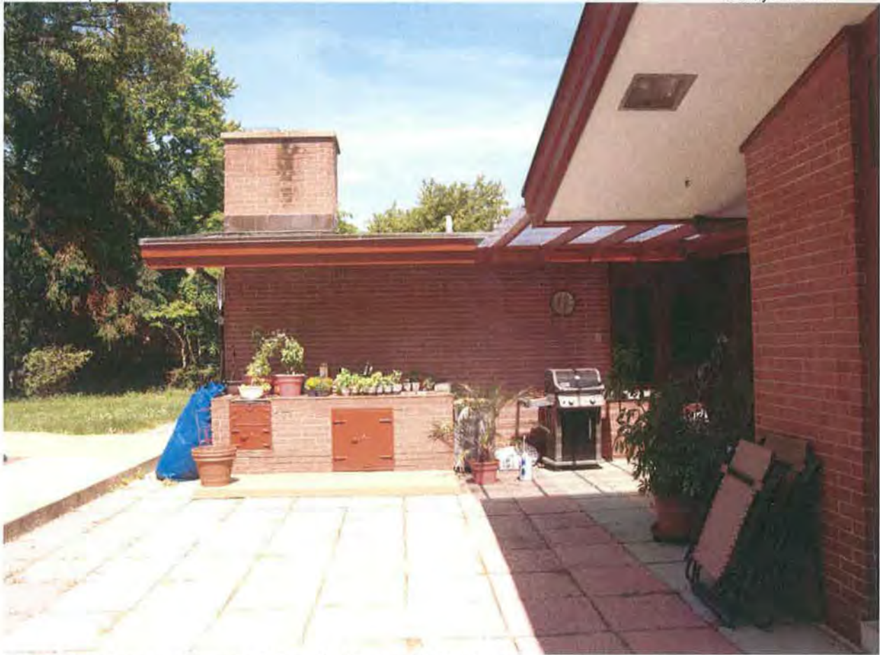
MD_PrinceGeorgesCounty_MarenkaHouse_006 Ell, east elevation, looking west
