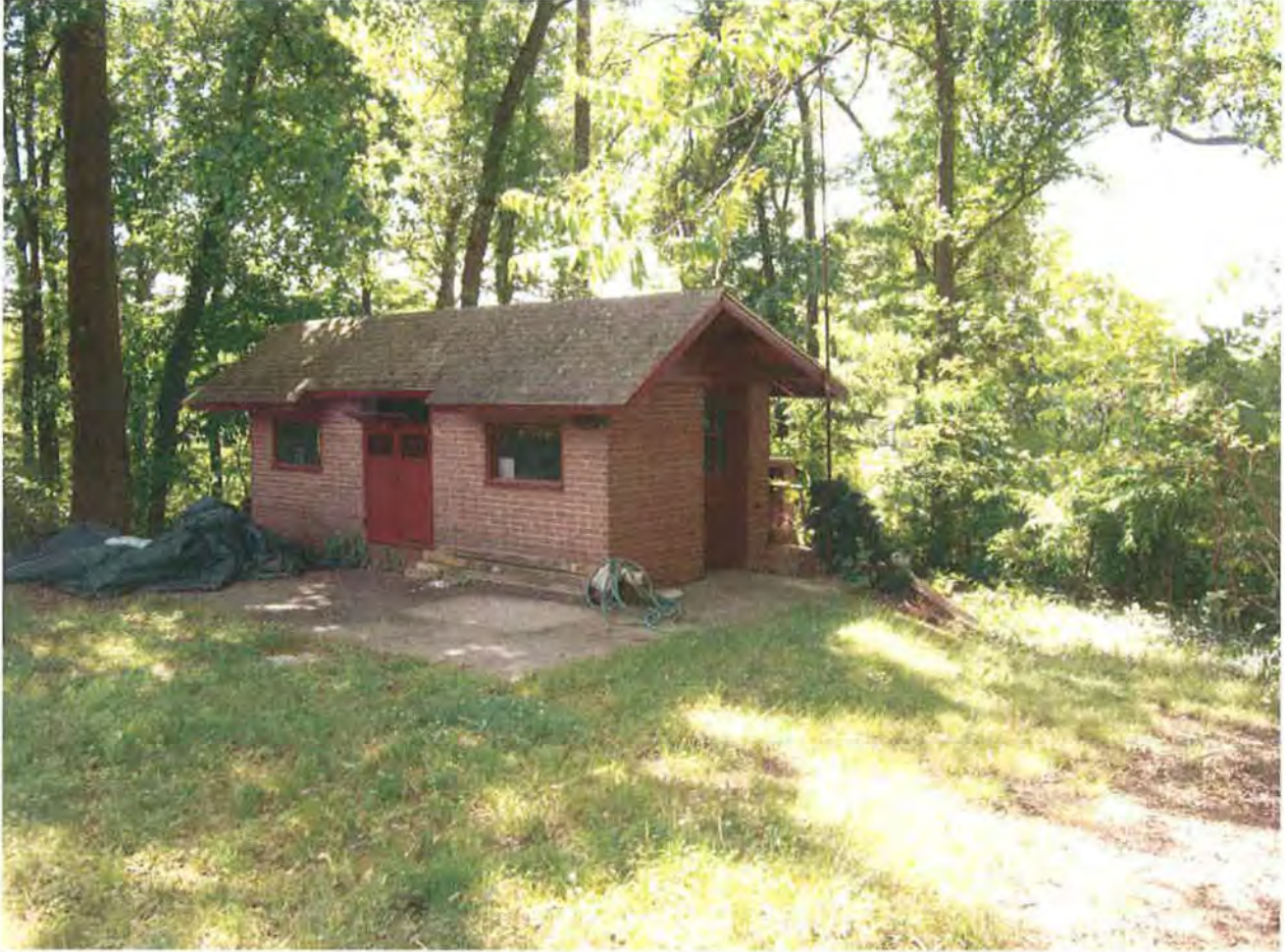
MD_PrinceGeorgesCounty_MarenkaHouse_016 Pigeon cote, north and west elevations
