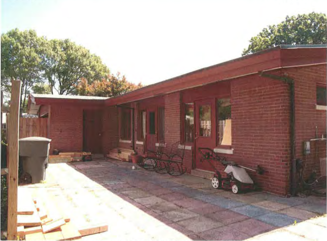
MD_PrinceGeorgesCounty_MarenkaHouse_005 Ell, west elevation, looking northeast
