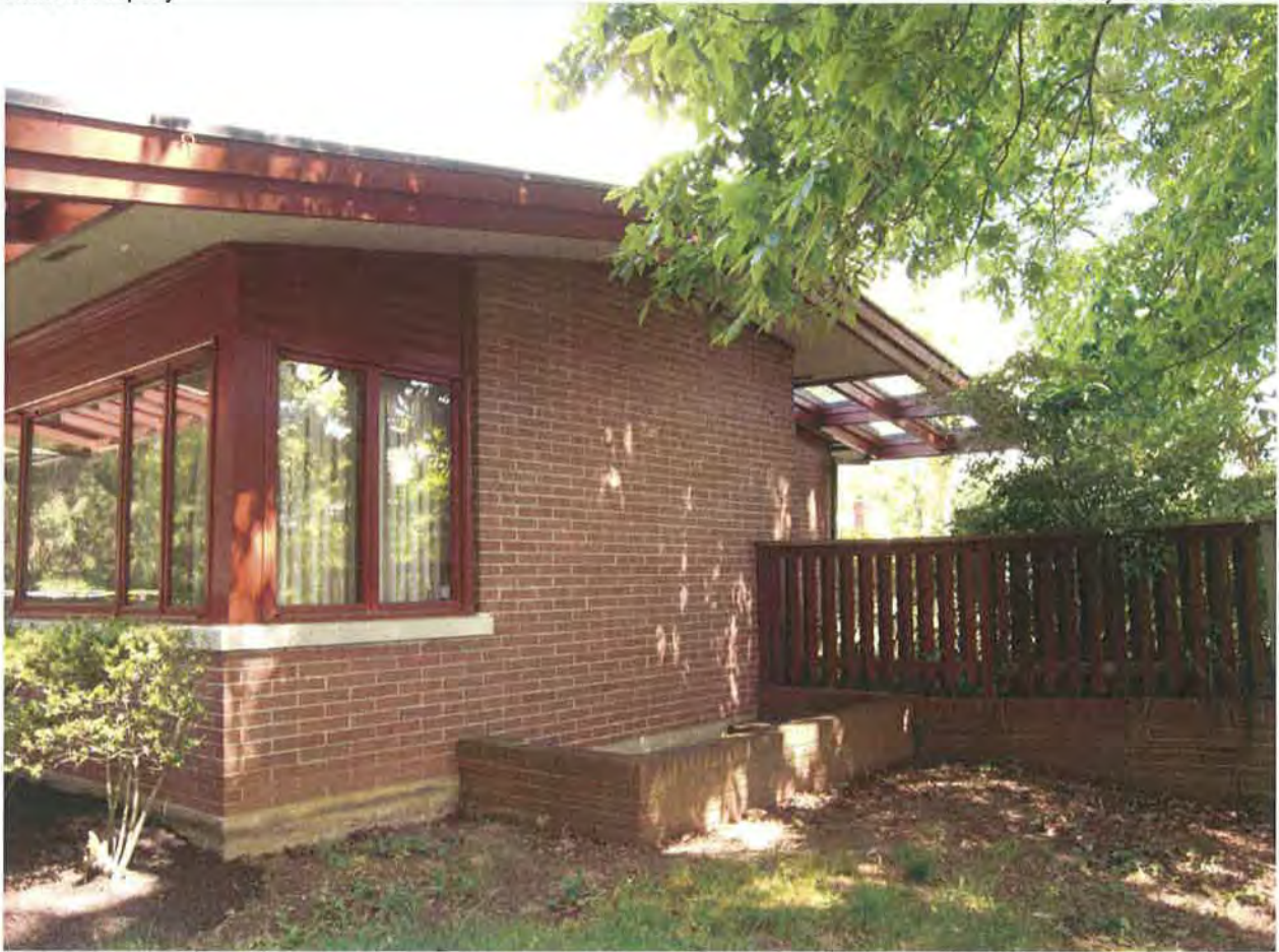
MD_PrinceGeorgesCounty_MarenkaHouse_003 East Elevation, looking southwest
