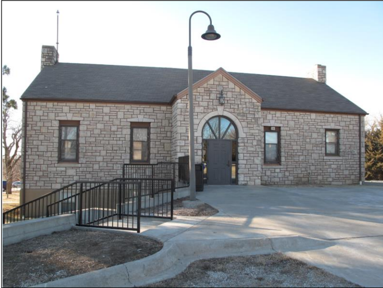
Figure 4: Prairie Band Potawatomi Nation Community Building at Mayetta in Jackson County, Kansas. Photo by KSHS, January 2015.
