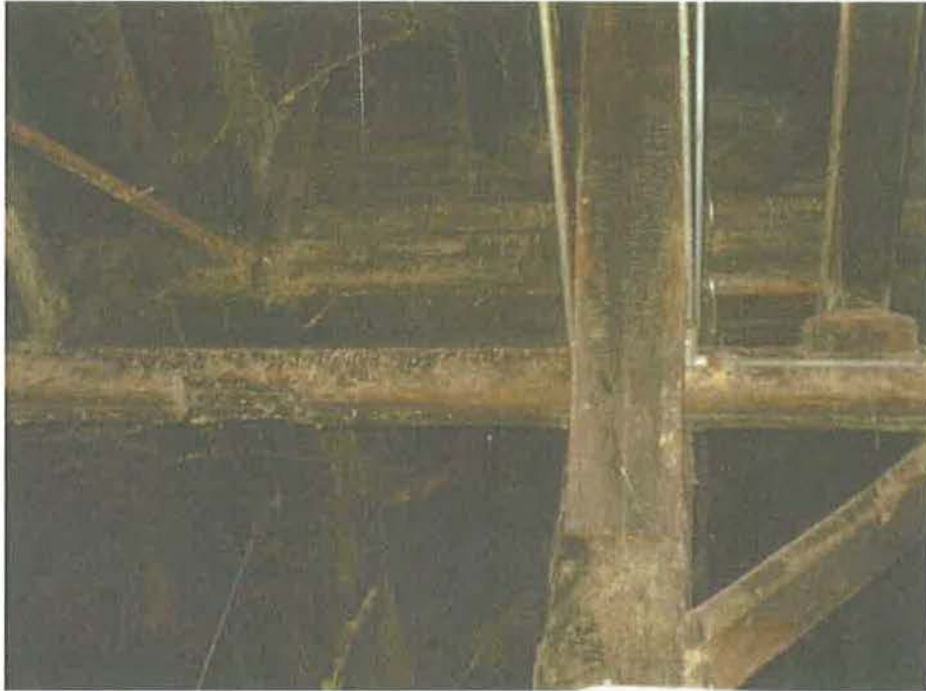
Photo 7: First-floor framing – post, beam and diagonal kicker
