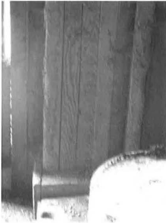
Photo 5: Typical built-up perimeter post
