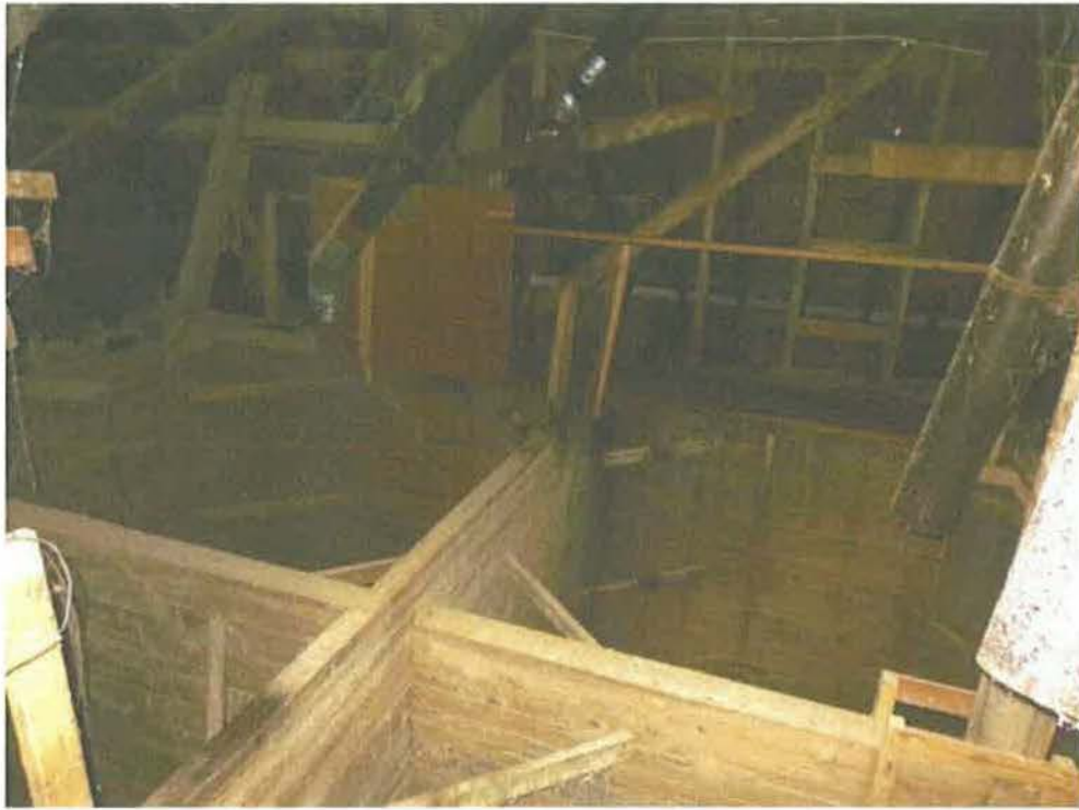
Photo 9: Top of grain bins with roof framing beyond.
