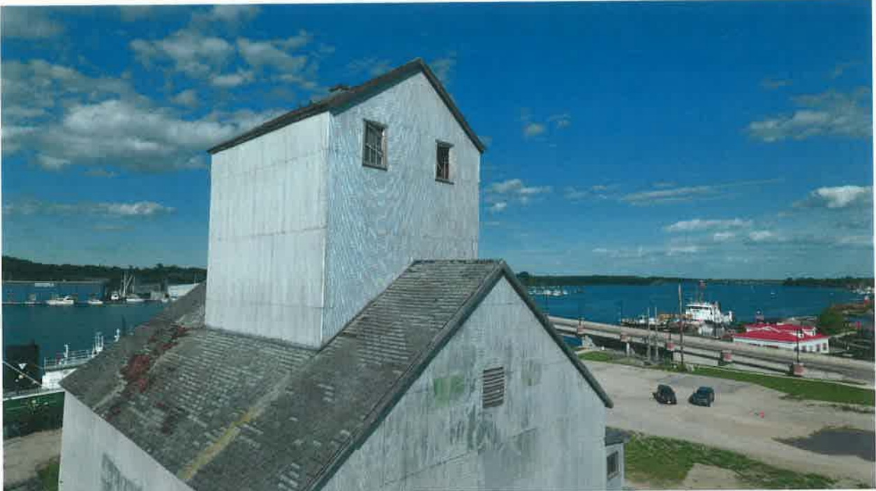
2017 Photos of the Midland (Former Tewles & Brandies) Elevator
