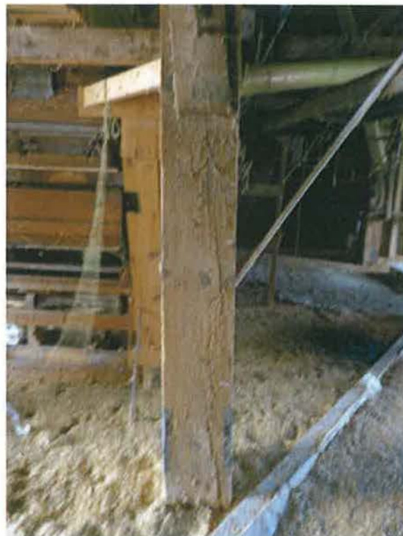
Photo 4: Interior solid posts
