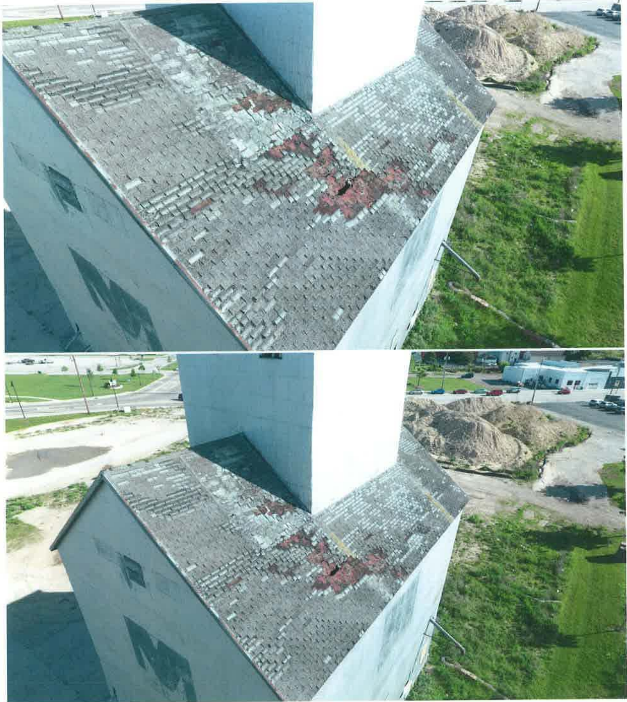
2017 Photos of the Midland (Former Tewles & Brandies) Elevator
