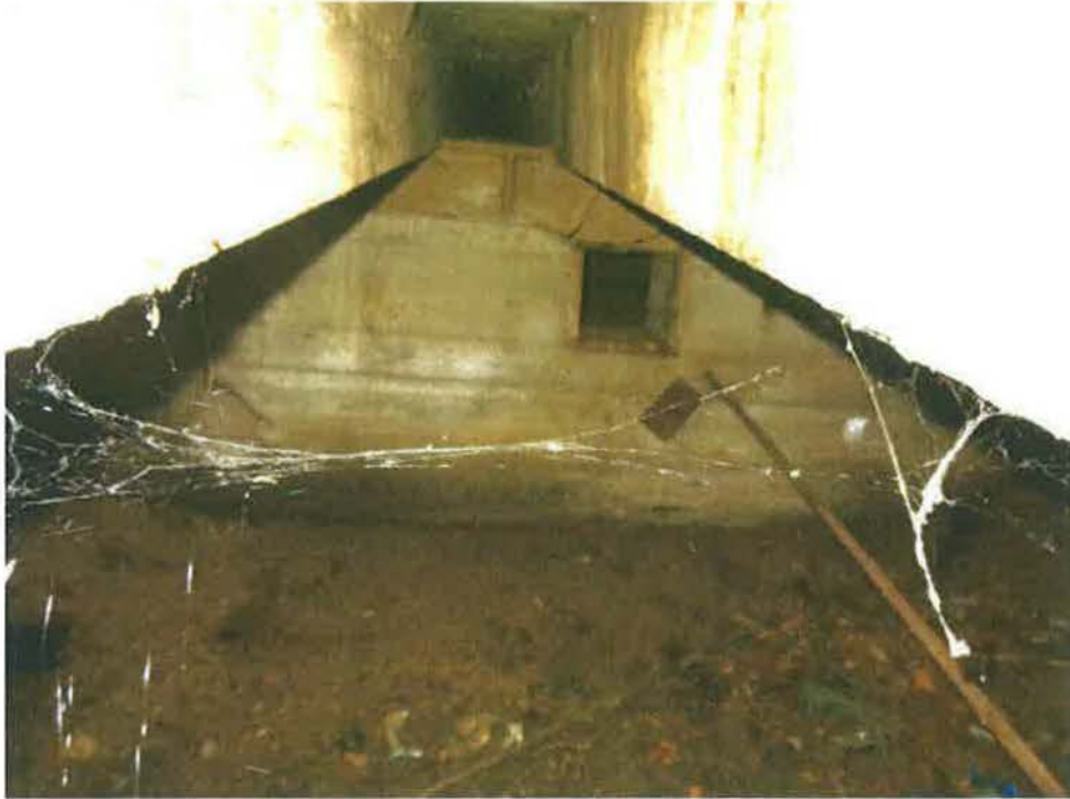
Photo 1: Foundation wall at shallow basement
