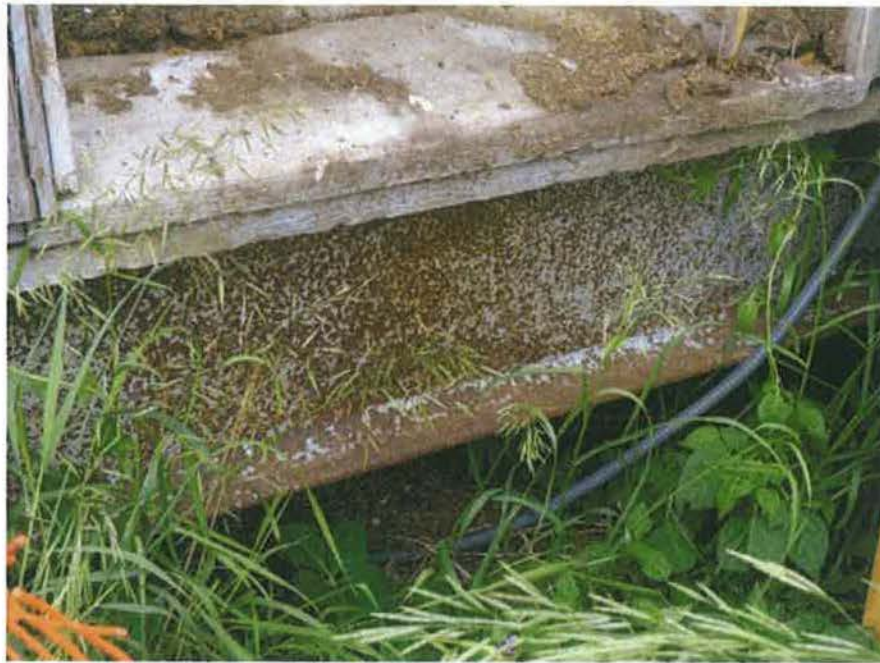
Photo 3: Steel beam under north wall
