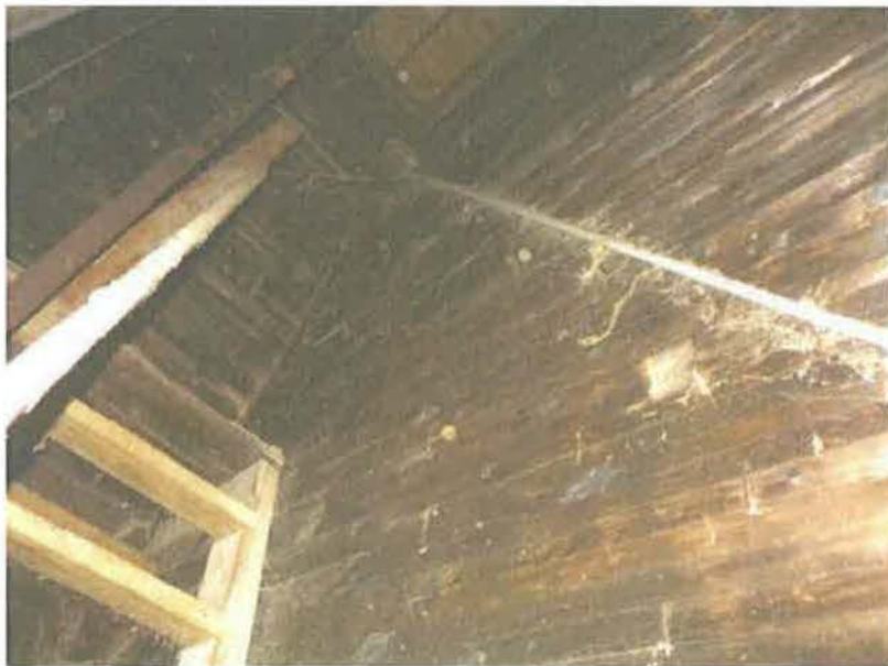
Photo 8: Grain bin showing cribbed-construction
