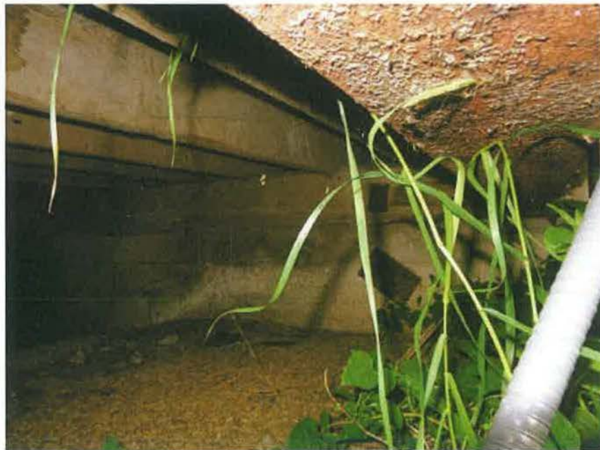
Photo 2: Foundation grade-beam with wood joists above
