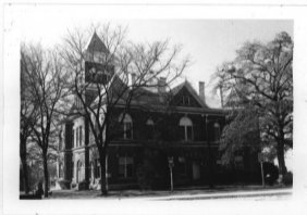
MADISON COUNTY COURTHOUSE
