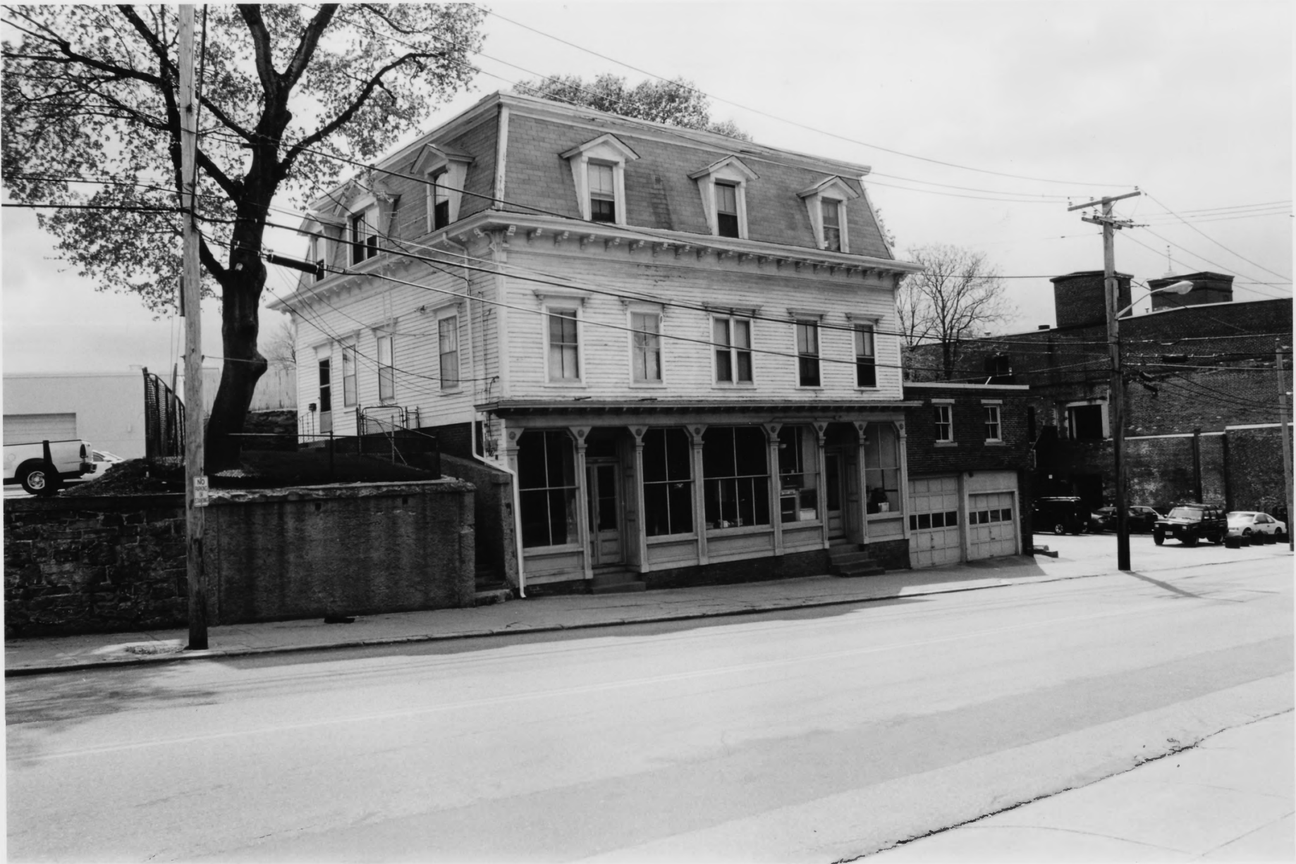
Nickerson-Charland Building Exchange Street Historic District Pawtucket, Providence County, Rhode Island Photograph No. 9
