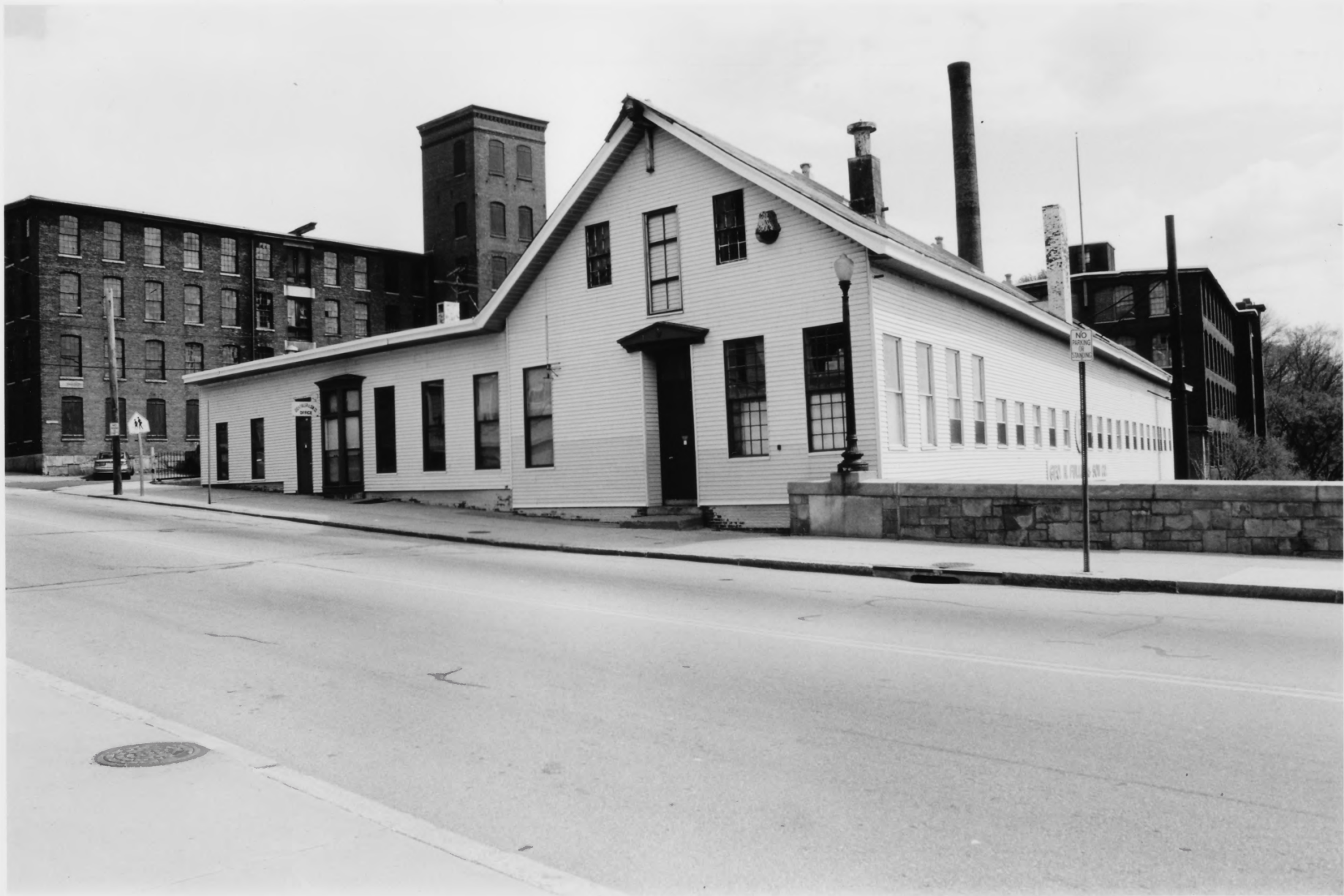
George H. Fuller & Son Company Exchange Street Historic District Pawtucket, Providence County, Rhode Island Photograph No. 4
