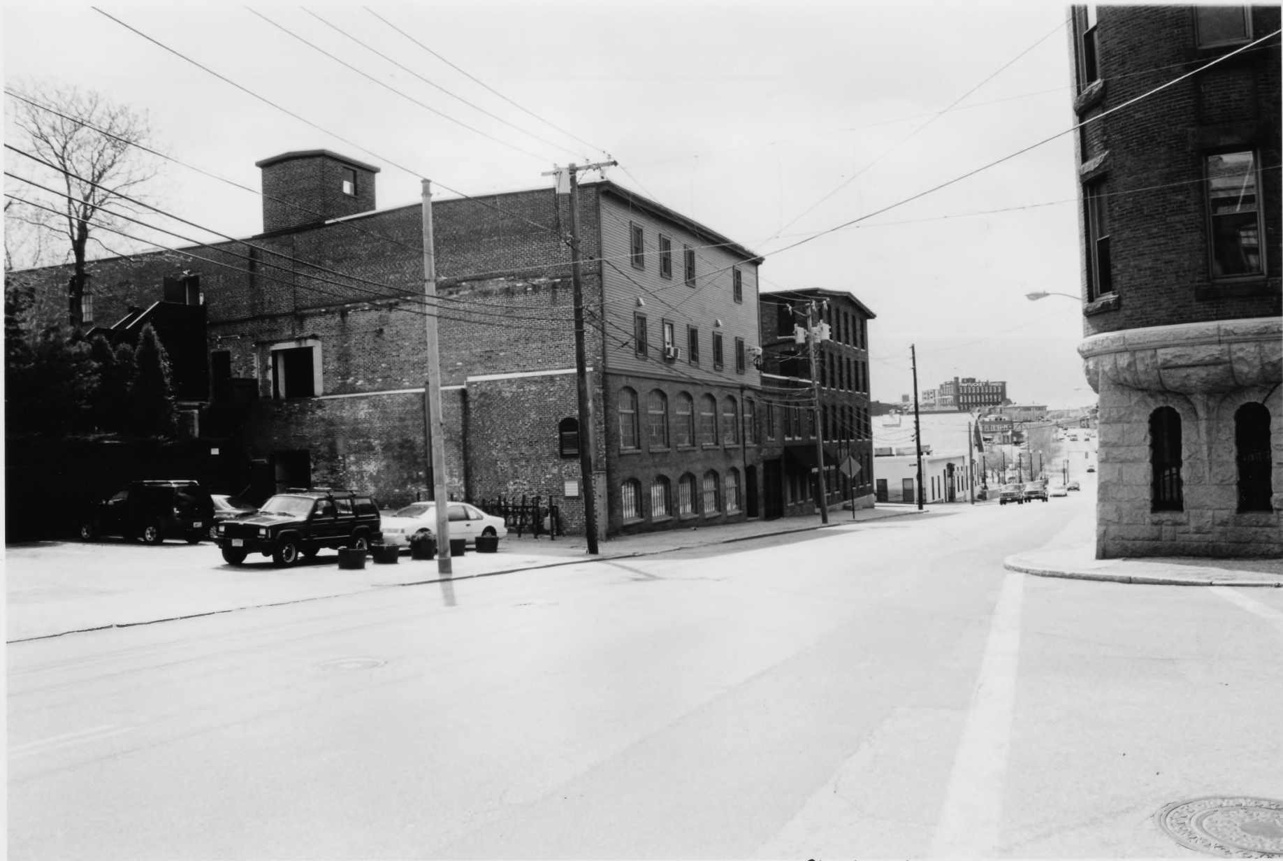
Rhode Island Card Board Company Exchange Street Historic District Pawtucket, Providence County, Rhode Island Photograph No. 10
