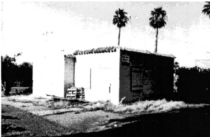
Monterey Park Pumphouse
