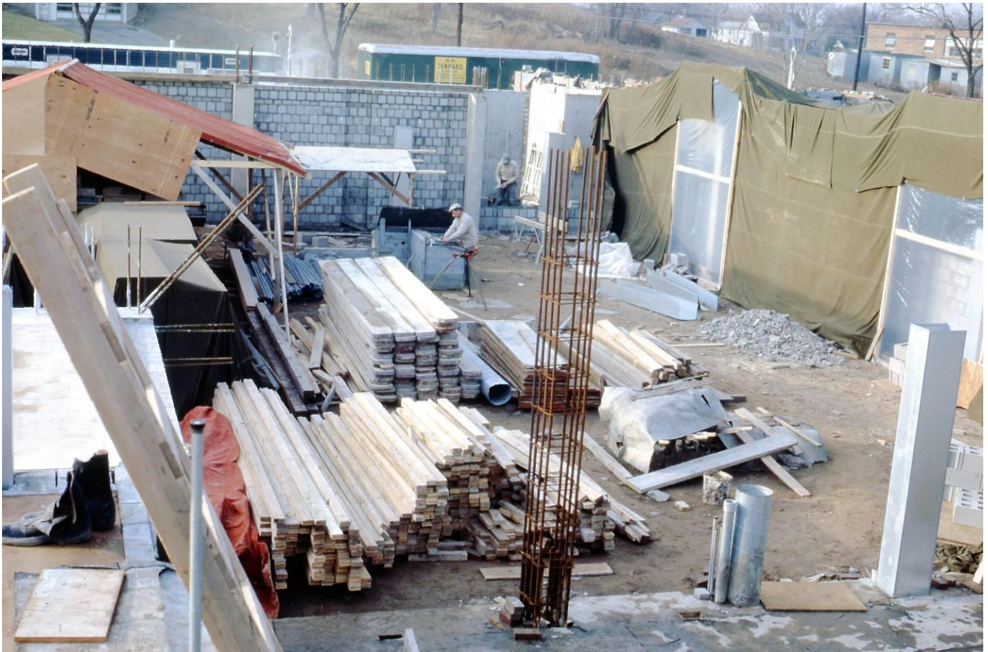
Figure 23: First Unitarian Church – Building Construction (ca. 1961)
