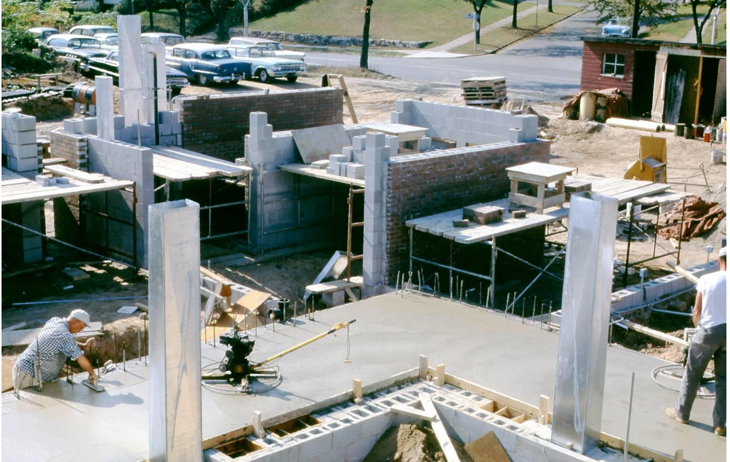
Figure 24: First Unitarian Church – Building Construction (ca. 1961)
