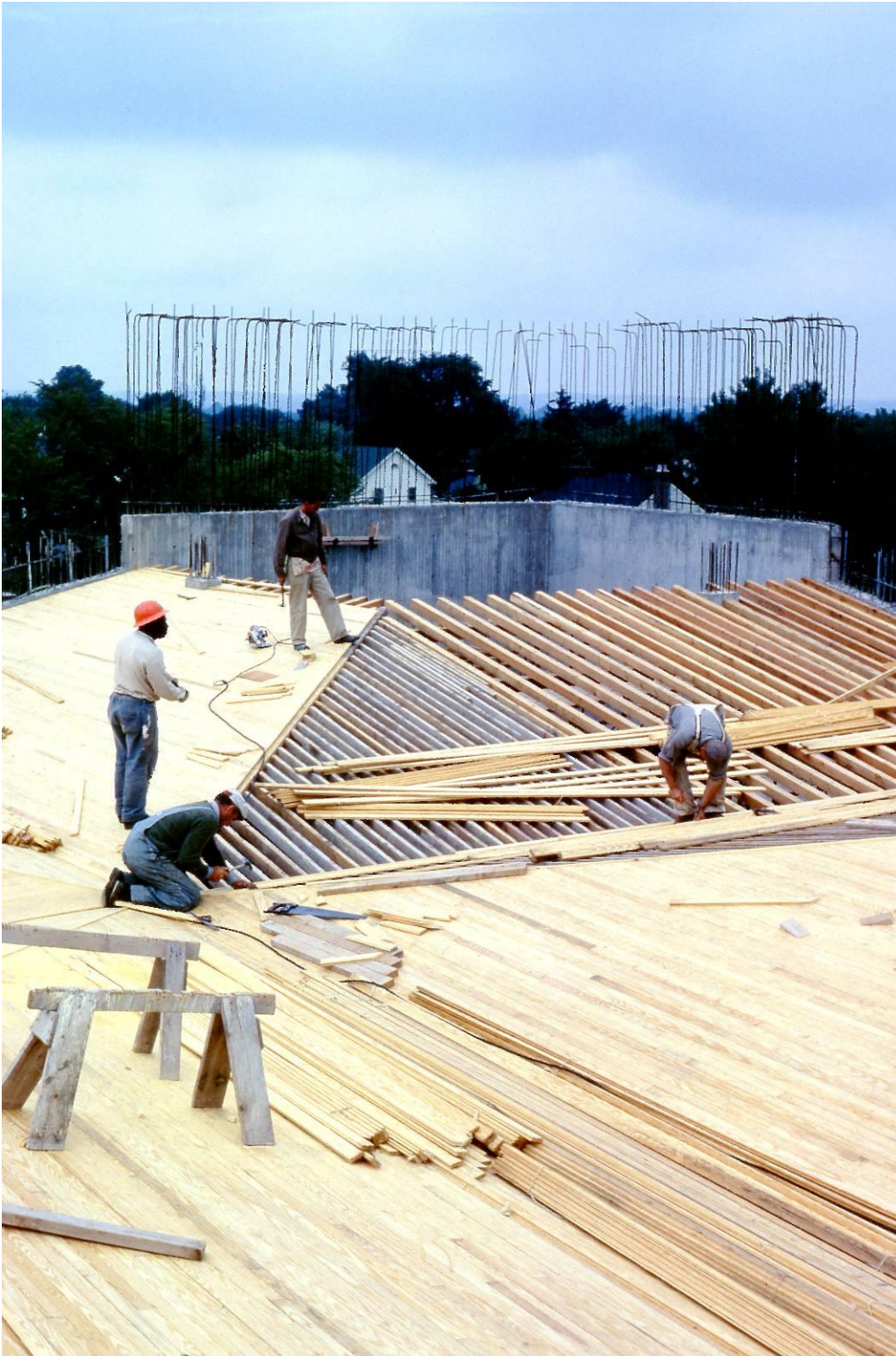
Figure 26: First Unitarian Church – Building Construction (ca. 1961)
