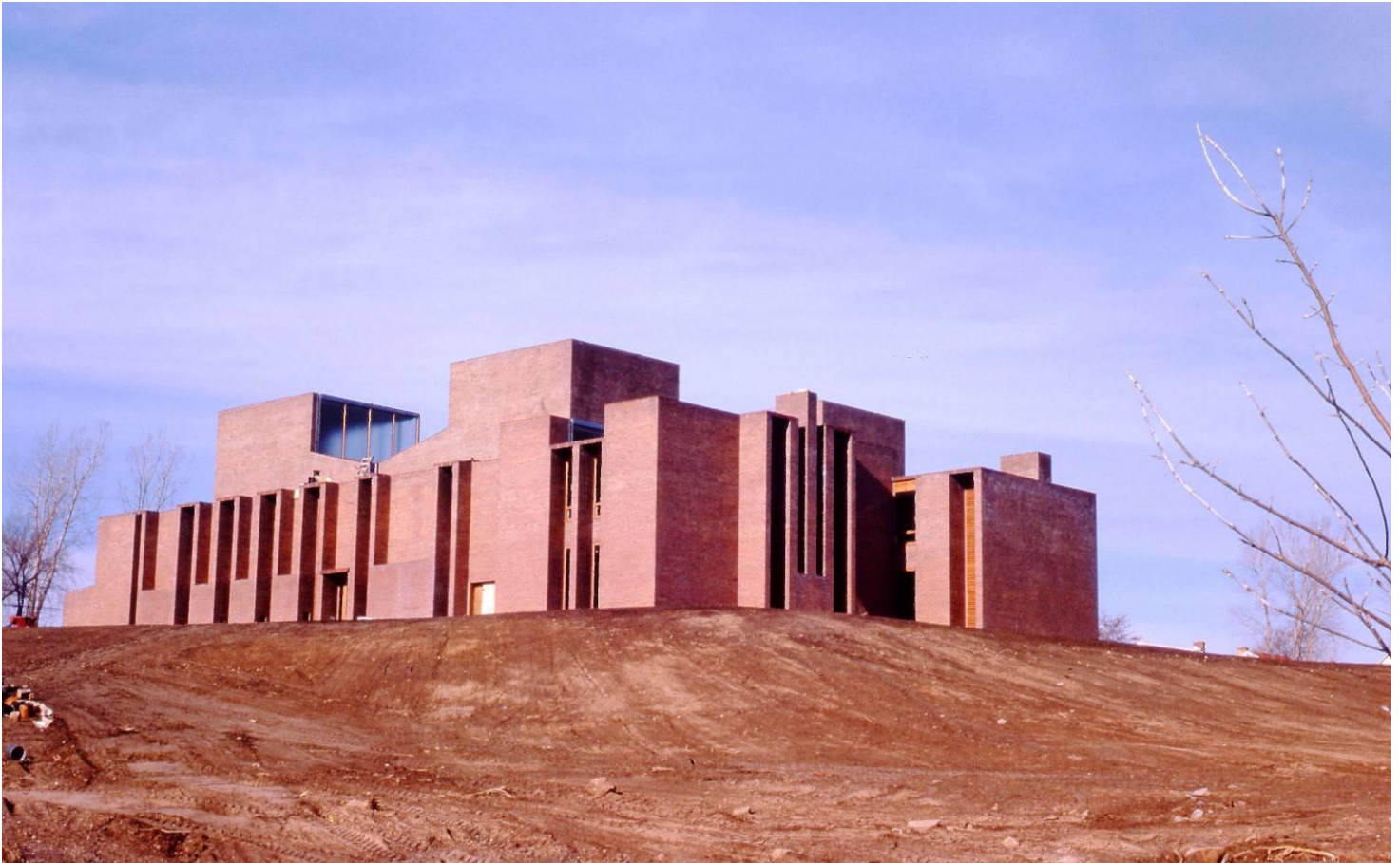
Figure 27: First Unitarian Church – Building Construction (ca. 1962)
