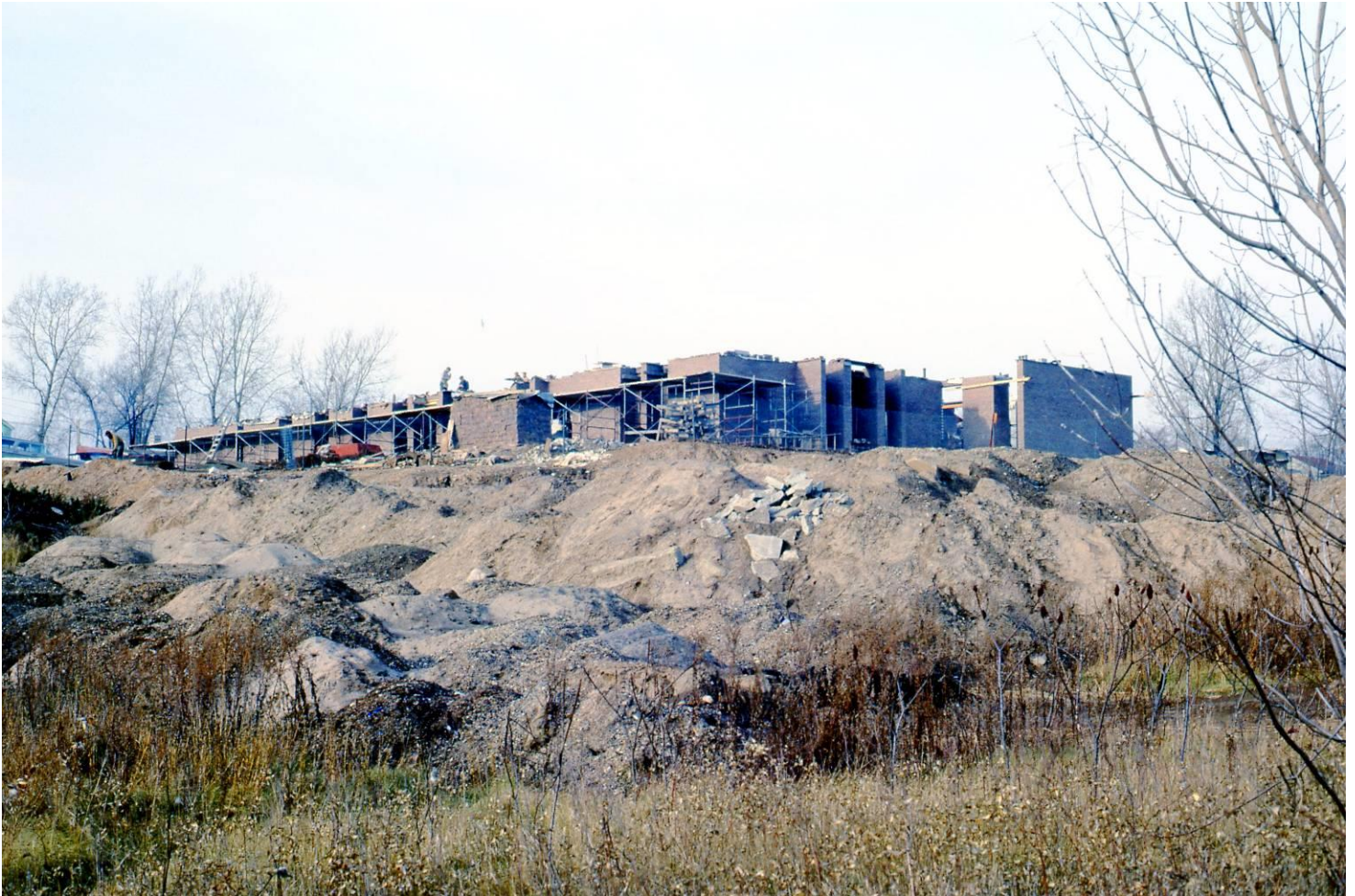
Figure 25: First Unitarian Church – Building Construction (ca. 1961)
