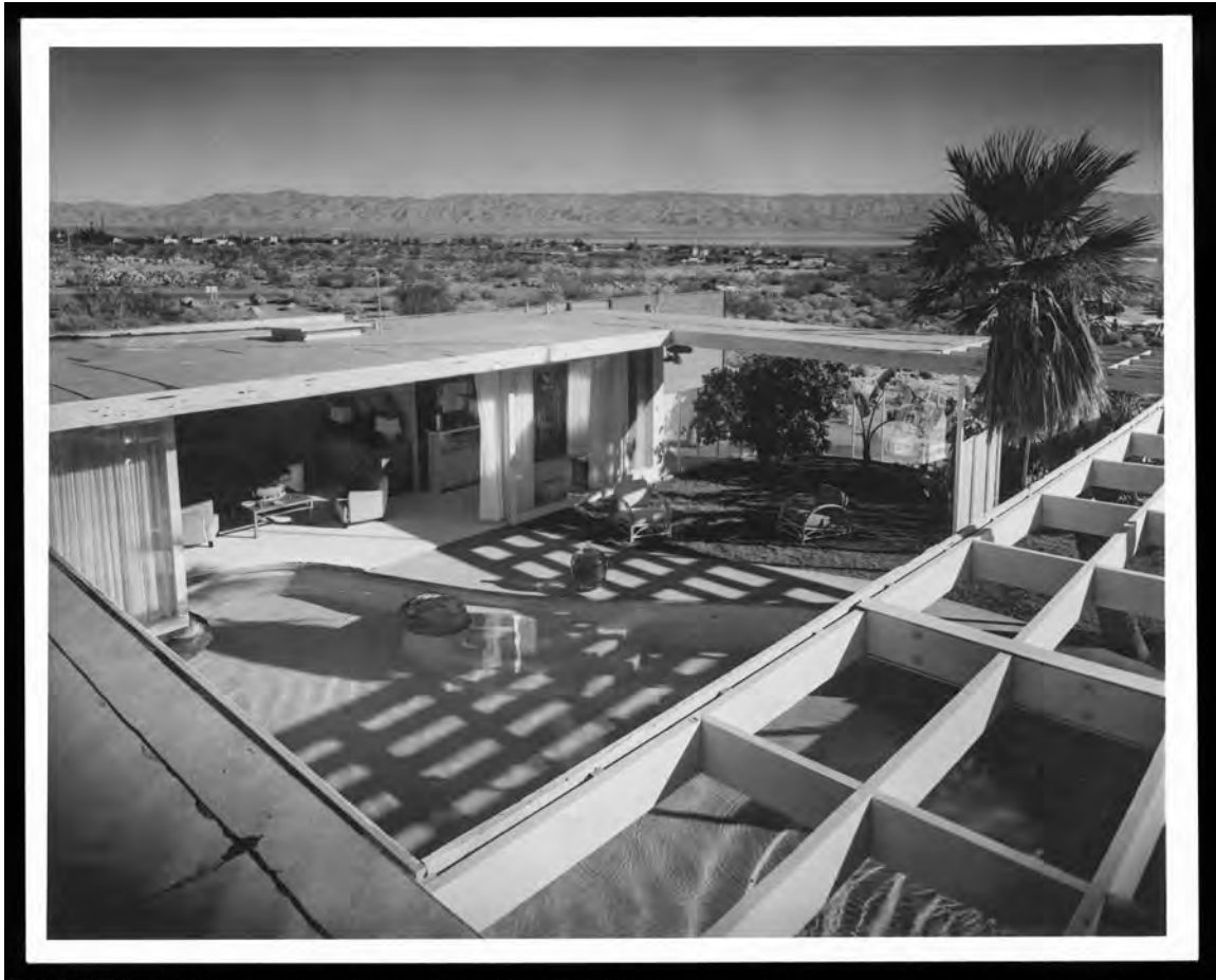
Figure 2. South and west elevations, looking northeast, 1947.
