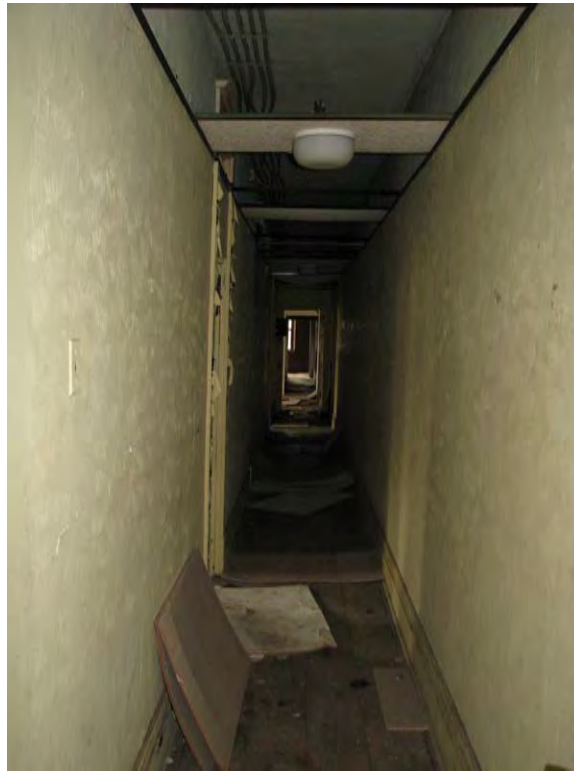
Photo 20. Second floor, looking south, showing the corridor and drop ceiling (P+A, 2018).
