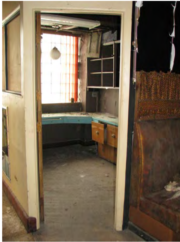
Photo 14. First floor, looking southwest, showing the office (P+A, 2018).
