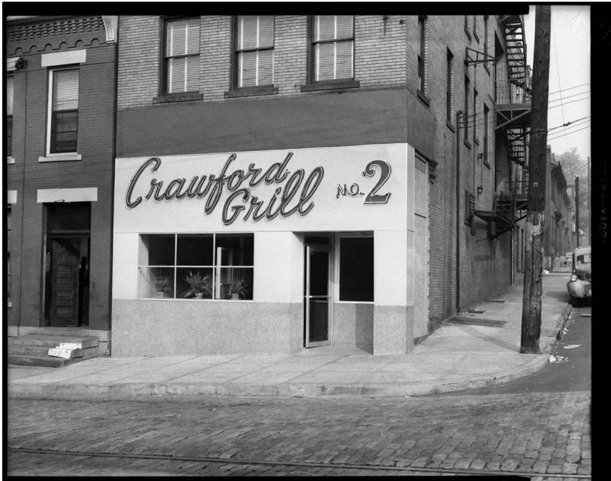
Figure 4. Front facade of the Crawford Grill No. 2 from 1953, showing the newly renovated storefront and neon sign on white Carrera Glass (© 2019 Carnegie Museum of Art, Charles “Teenie” Harris Archive— See full citation at end of Bibliography).
