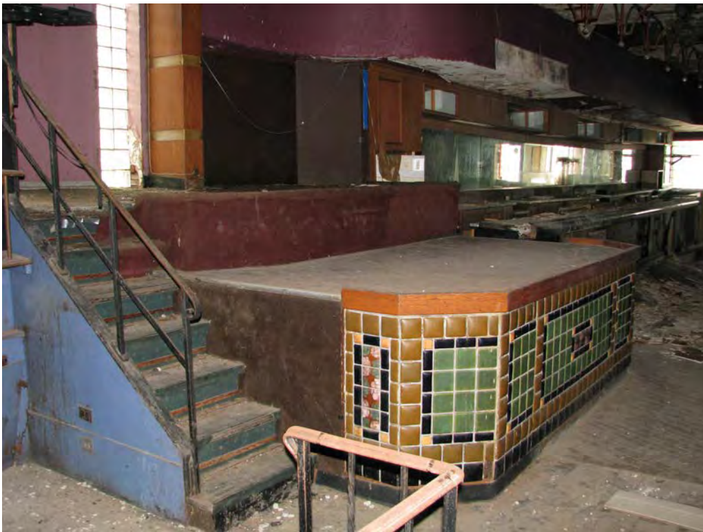
Photo 12. First floor, looking south, showing the stage, with stage door in upper left and bar beyond (P+A, 2018).
