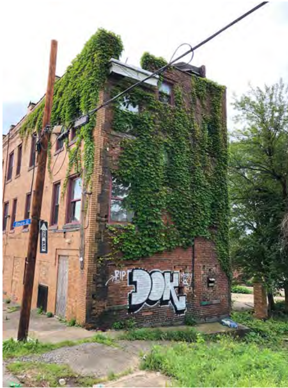
Photo 8. Rear facade, looking south, showing the door to the apartments at the rear of the east facade (T&P, 2019).
