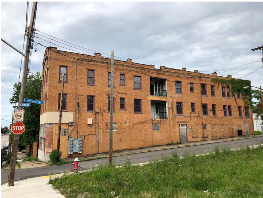
Photo 7. East facade, looking west, showing the stage door, center, and recessed porches of the second and third floor apartments (T&P, 2019).
