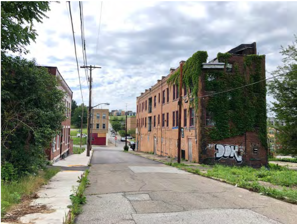
Photo 4. Elmore Street, looking south, showing the rear facade of the Crawford Grill No. 2 (T&P, 2019).
