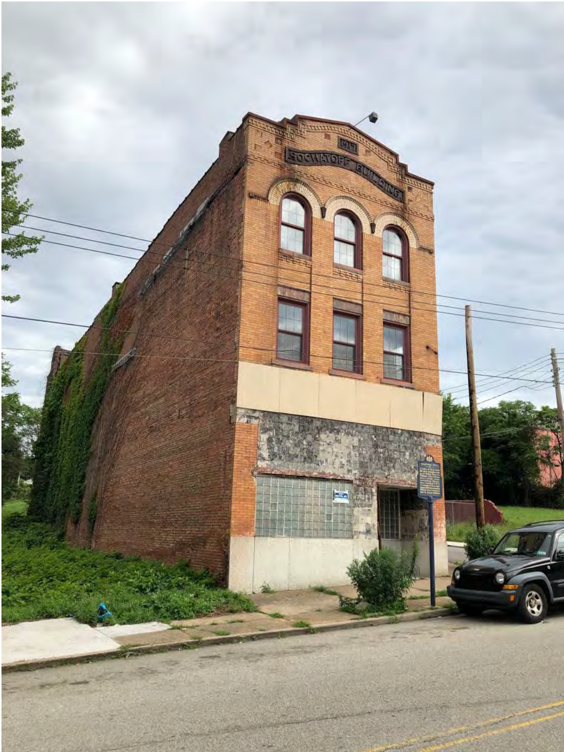
Photo 5. Front facade, looking north (T&P, 2019).
