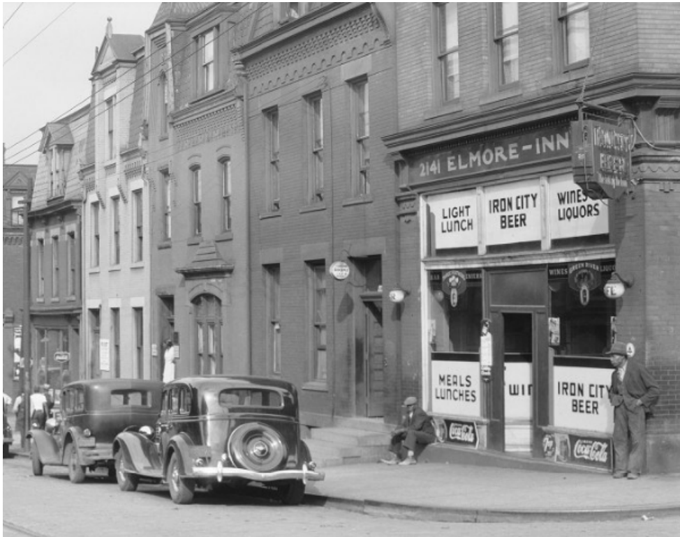
Figure 26. Exterior of 2141 Wylie Avenue (right) in 1937, showing how the Sochatoff Building looked around the time Gus Greenlee purchased it (Historic Pittsburgh, Pittsburgh City Photographer Collection).
