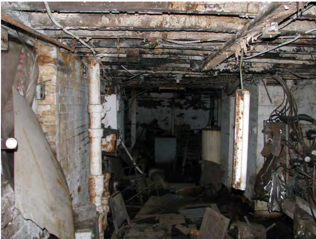
Photo 29. Basement, looking south into storerooms (P+A, 2018).
