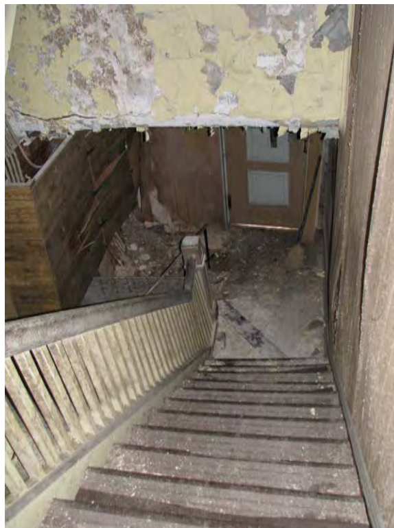
Photo 19. Second floor, looking east, showing the stairs for the apartments (P+A, 2018).
