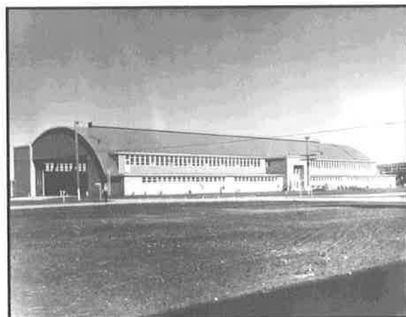
Figure 18 Drill Hall completed
