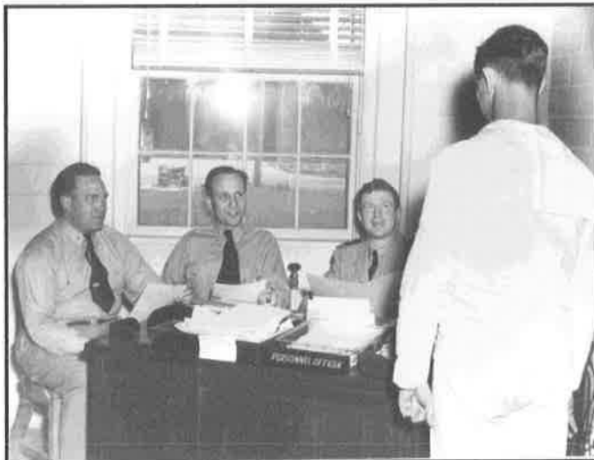
Figure 29 Personnel Office, first floor, south wing
