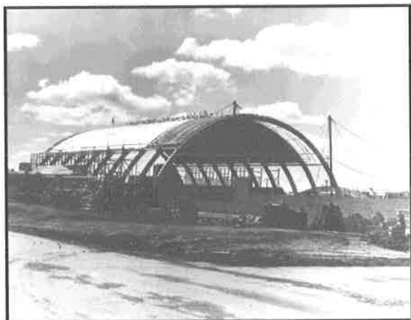
Figure 17 Drill Hall under construction
