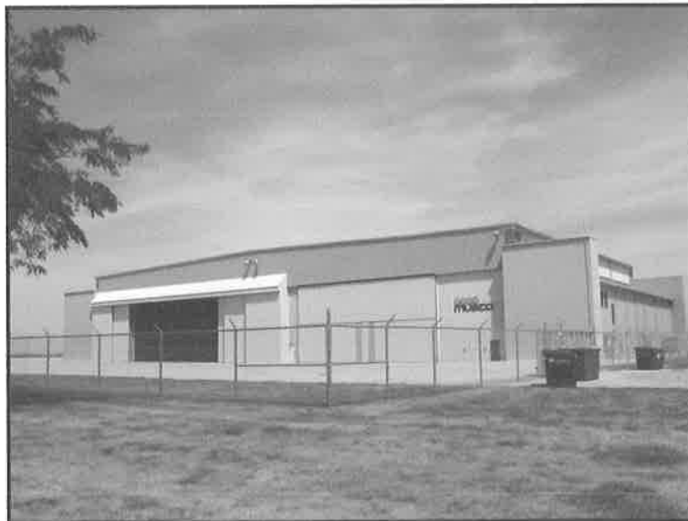
Figure 27 NAS Hanger #2 (#1 is non-extant), 2012 photograph
