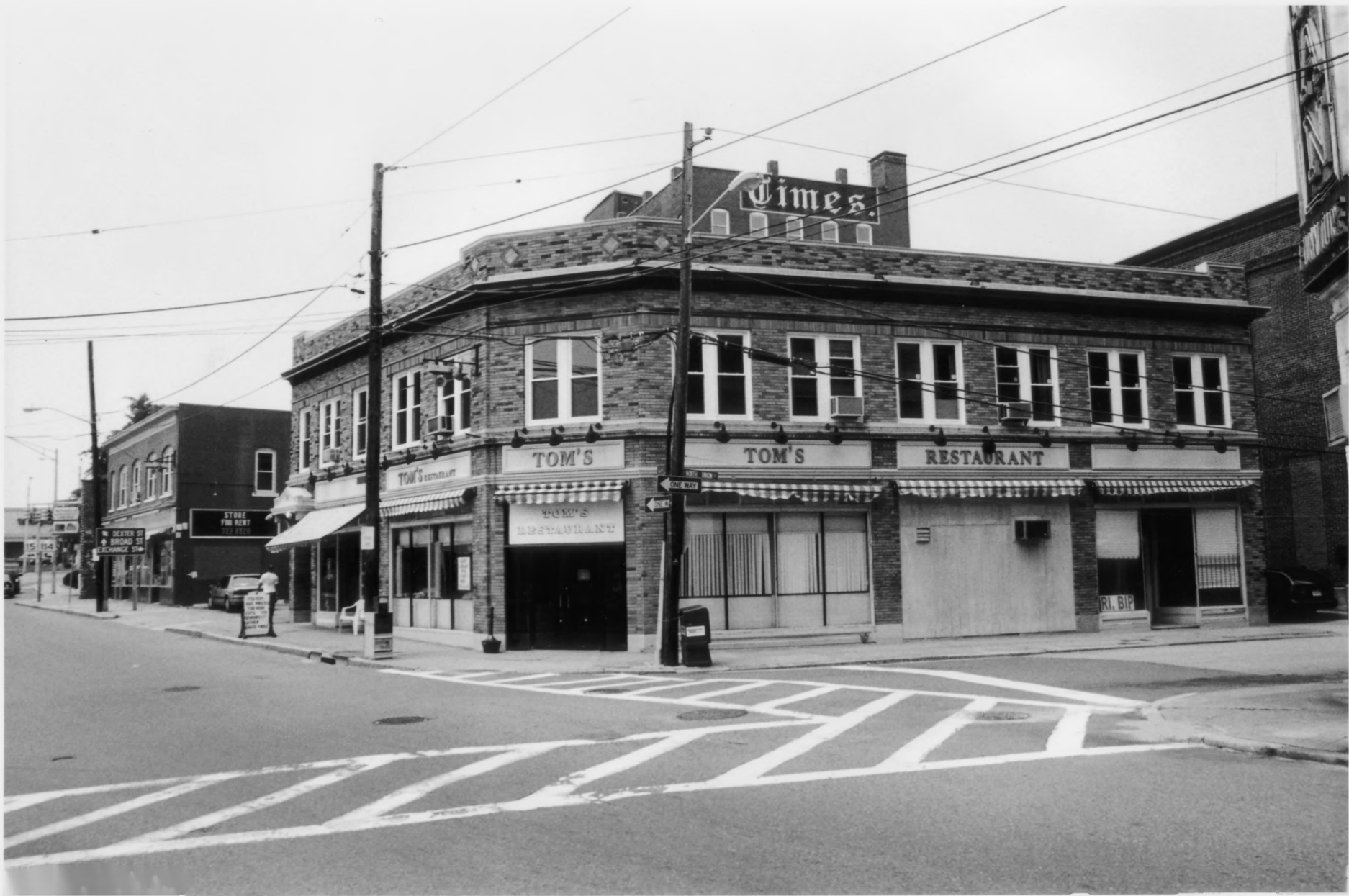
41-45 SUMMER ST. (LITTLE FURNACE BLDG.) + 29-33 SUMMER ST. (MORRIS PLAN CO. BLDG.) TOWNSHIP HISTORIC DISTRICT, PALMYRA, PA. PHOTO #10
