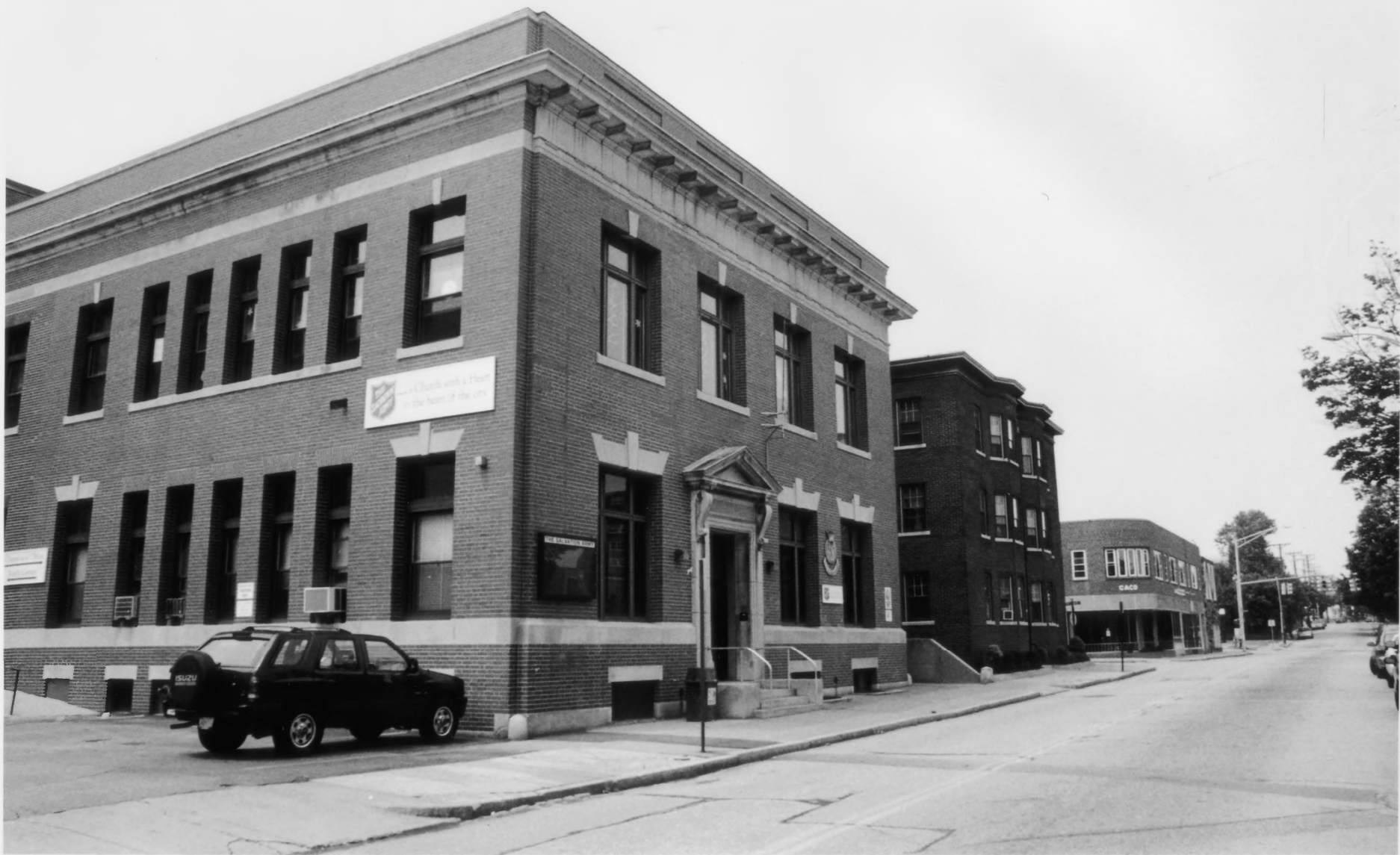
100 HIGH ST. (PROVIDENCE TELEPHONE CO.), 110 HIGH ST. (MONAST APTS.), 120 HIGH ST (DISANORO BLDG.) DOWNTOWN PAWTUCKET HISTORIC DISTRICT, PAWTUCKET, RI
