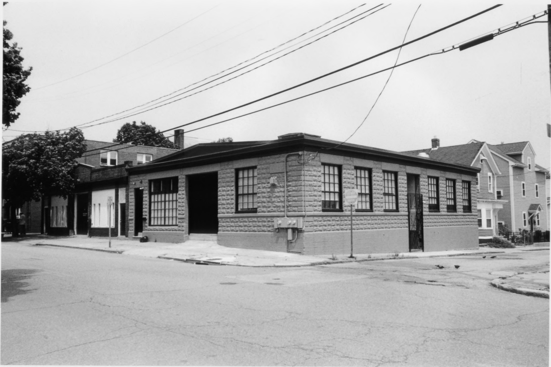
75 North Main St. (Rear View), 4 East St. (Houses - Apples House) Pawtucket Historic District, Pawtucket, RI Photo # 13
