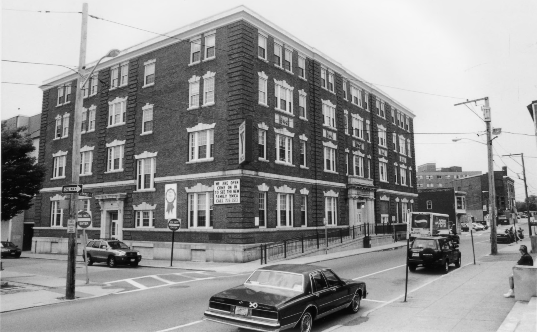
10 Building of YMCA Building 1000th Street, New York, New York, N.Y.
