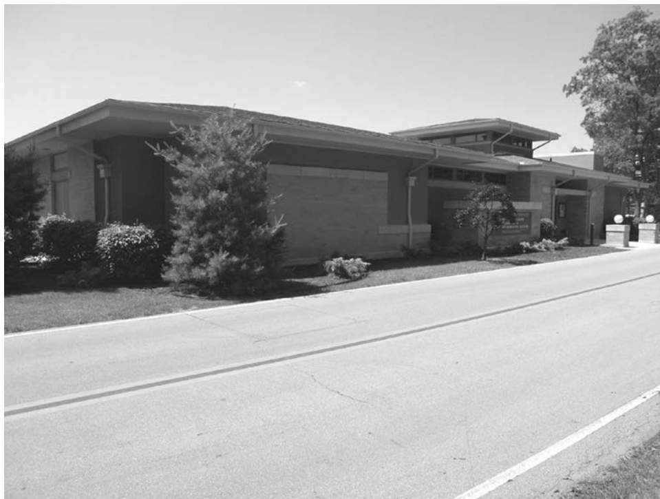
Photo 30. View of northeast corner of interpretive center located south of plaza, looking southwest
