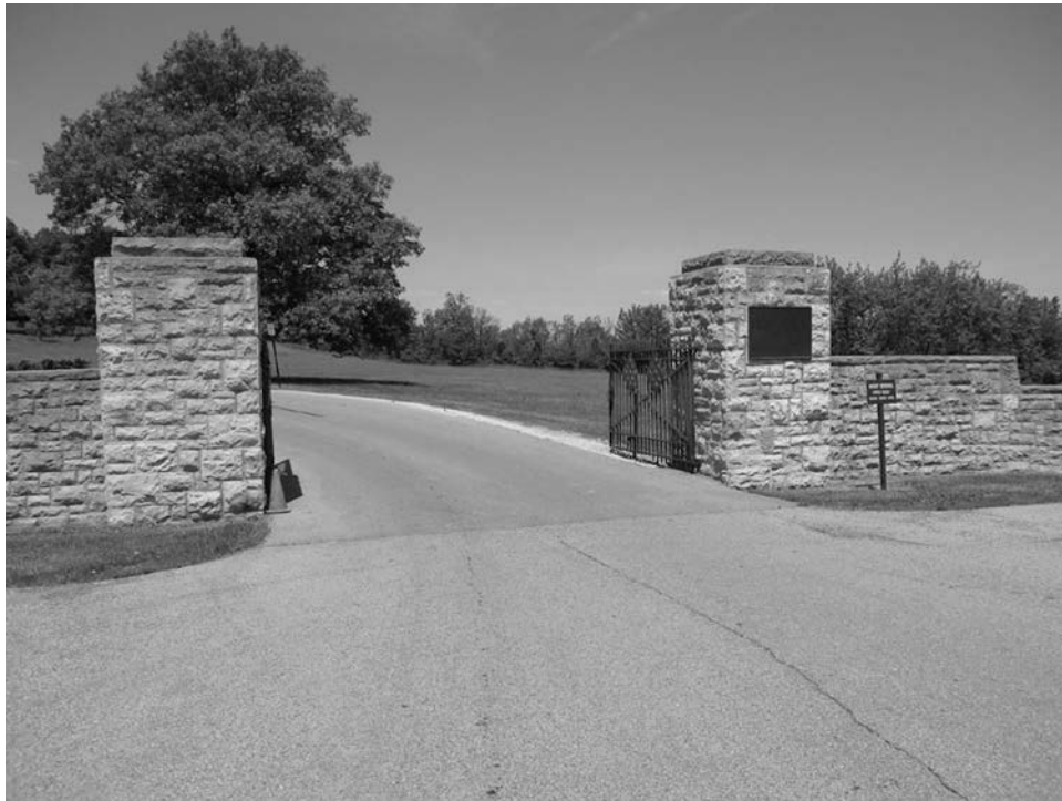
Photo 1. Stone entrance gates to Wright Brothers Hill, looking northwest from Skyline Drive
