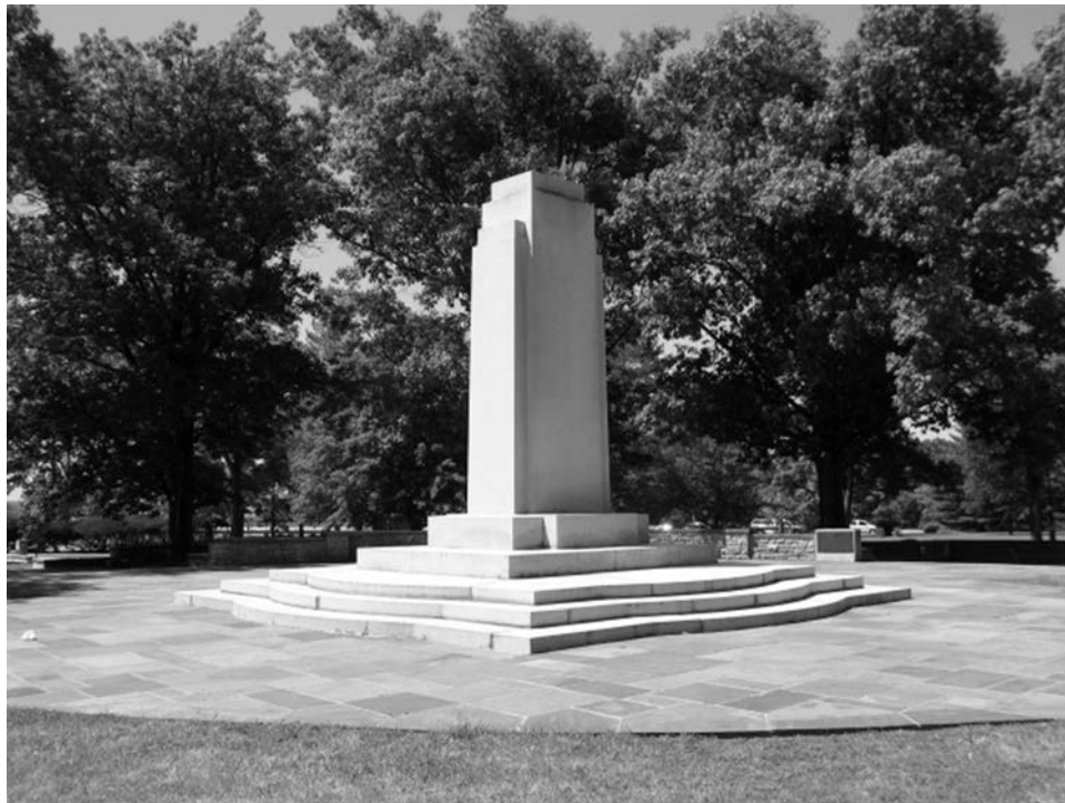
Photo 18. Northeast side of shaft, looking southwest from inner circle of plaza
