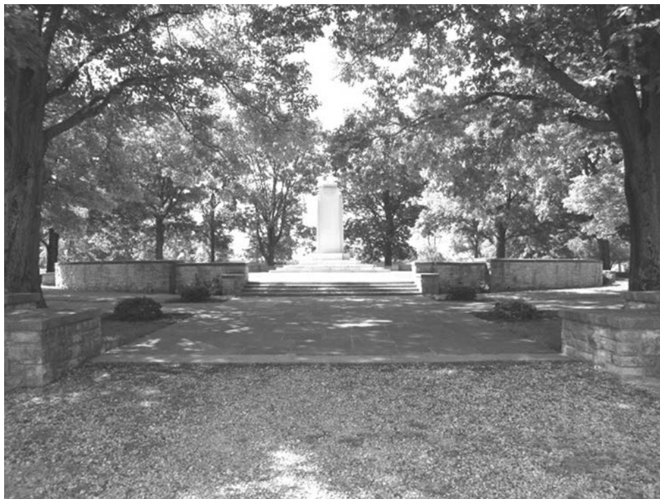
Photo 16. View of memorial plaza and shaft from north opening of plaza, looking south
