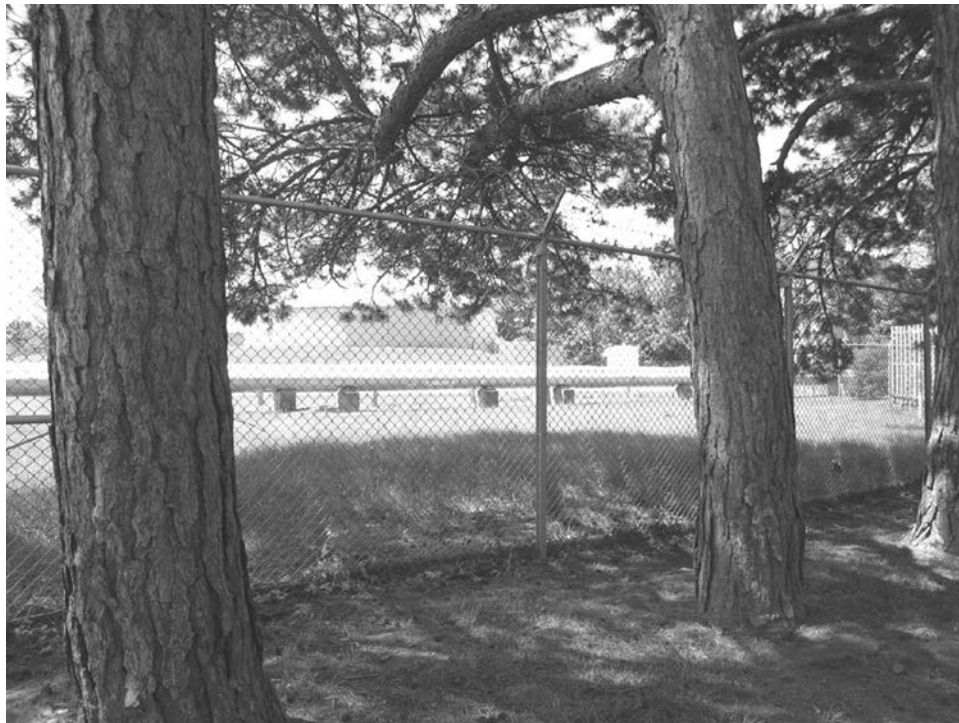
Photo 4. Wright-Patterson water treatment plant south of memorial park, looking southwest
