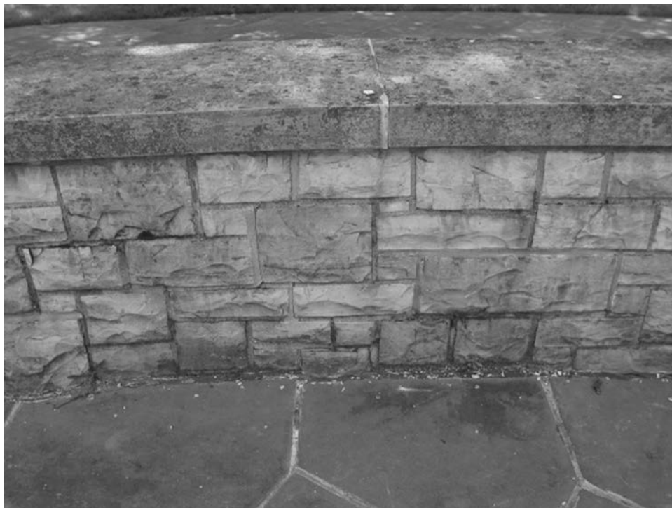
Photo 22. Detailed view of limestone inner wall located southeast of memorial shaft, looking southeast
