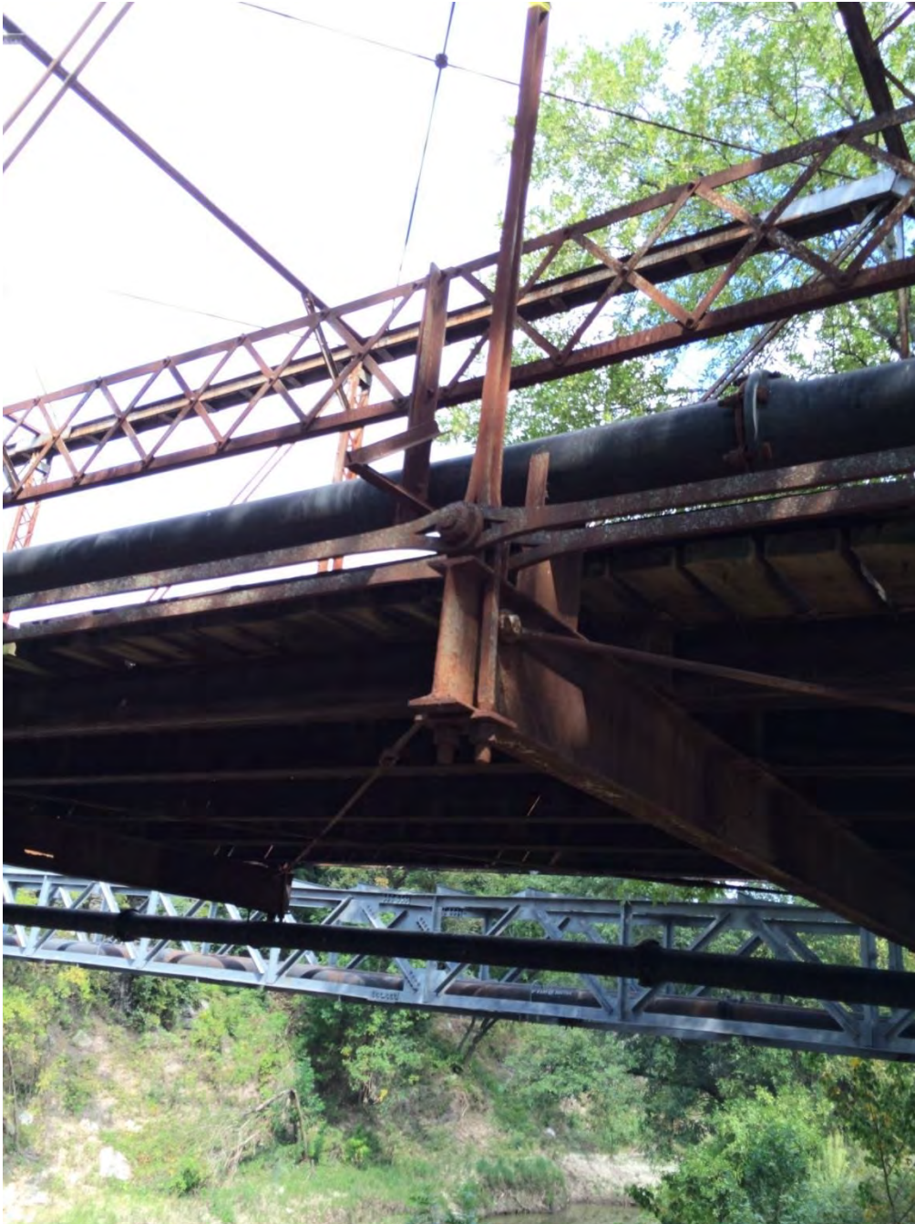
Photo 10: Pin connection. Camera facing north. Photo by Linda Henderson, Texas Historical Commission
