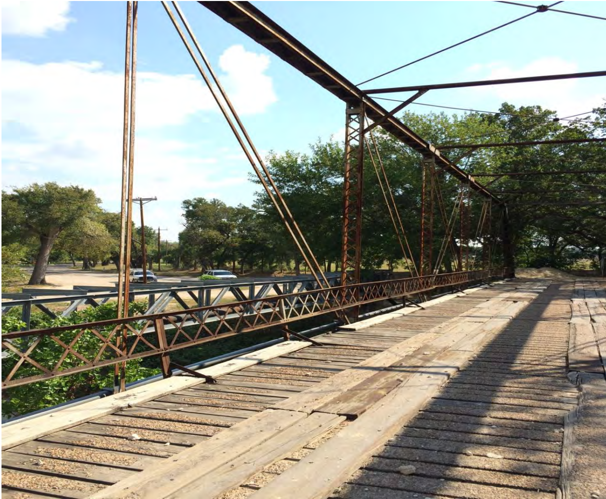
Photo 3: Latticed side railings. Camera facing northeast. Photo by Rebekah Dobrasko, Texas Department of Transportation
