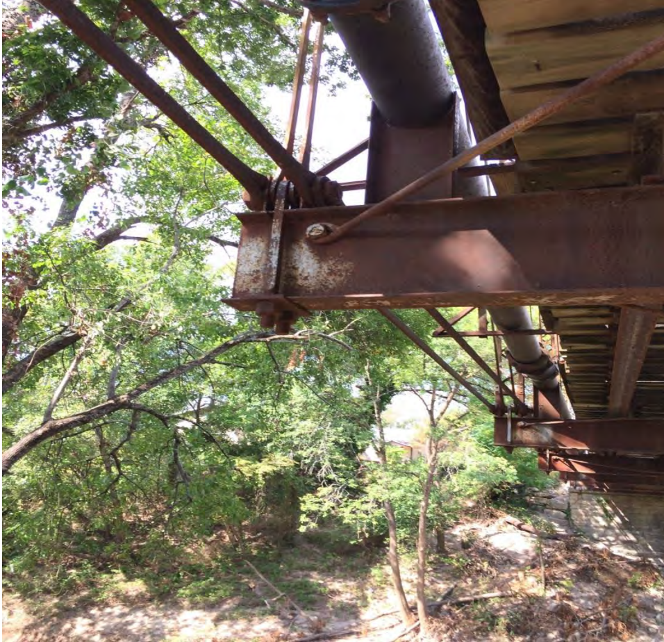
Photo 4: Pin connection. Camera facing west. Photo by Linda Henderson, Texas Historical Commission.
