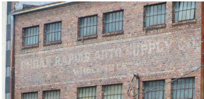
Image 31. 611 2 nd Avenue SE (rear signage)
