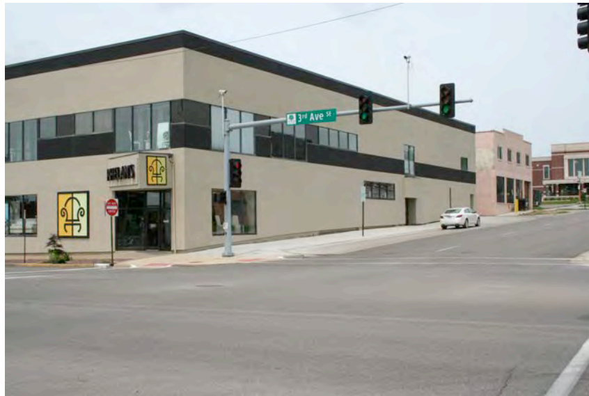
View of the northwest corner of the intersection of 3 rd Avenue SE and 8 th Street SE, looking northwest.
