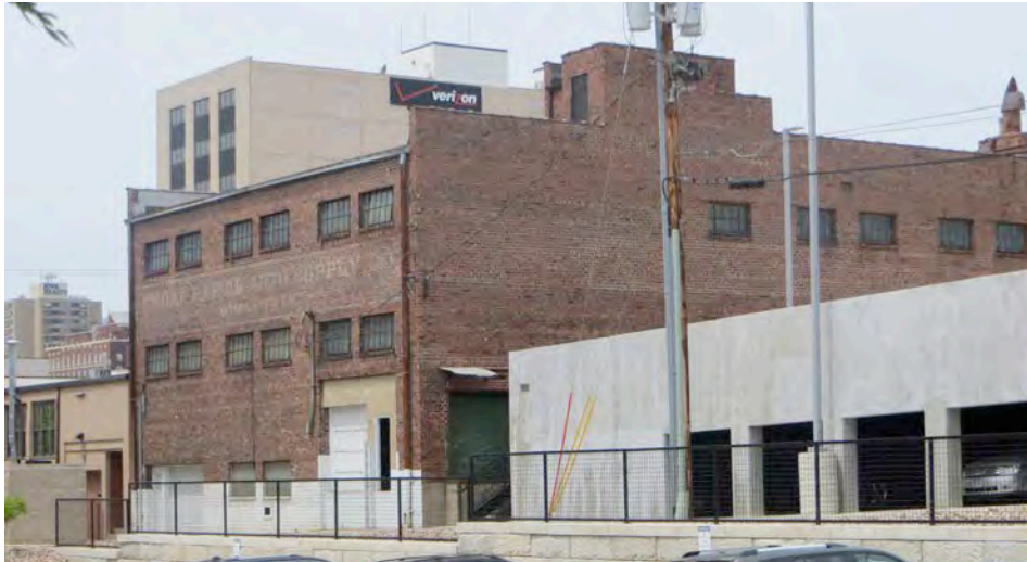
Image 30. 611 2 nd Avenue SE (rear elevation)
