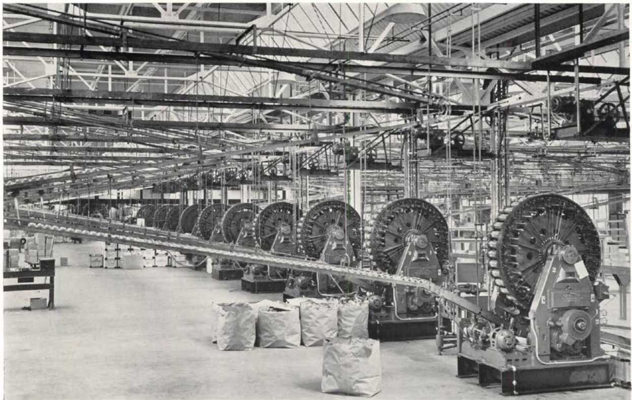
Figure 16 – Interior view showing can production in Building 1, from Architectural Record , February 1940.
