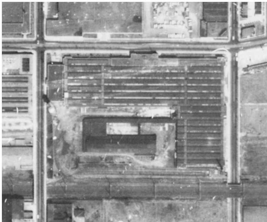
Figure 12 – Aerial view, 1965 (Delaware Valley Regional Planning Commission).
