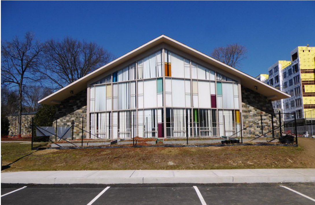
Figure 17: South elevation of Fellowship Hall, camera facing N from parking lot Photographer Wes Haynes, 2016
