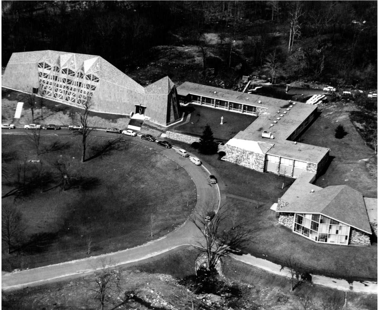
Figure 5: Sanctuary and parish unit (before tower construction), aerial view toward N Photograph DeLuca Construction, May 1966 Courtesy DeLuca Construction, Stamford, Connecticut
