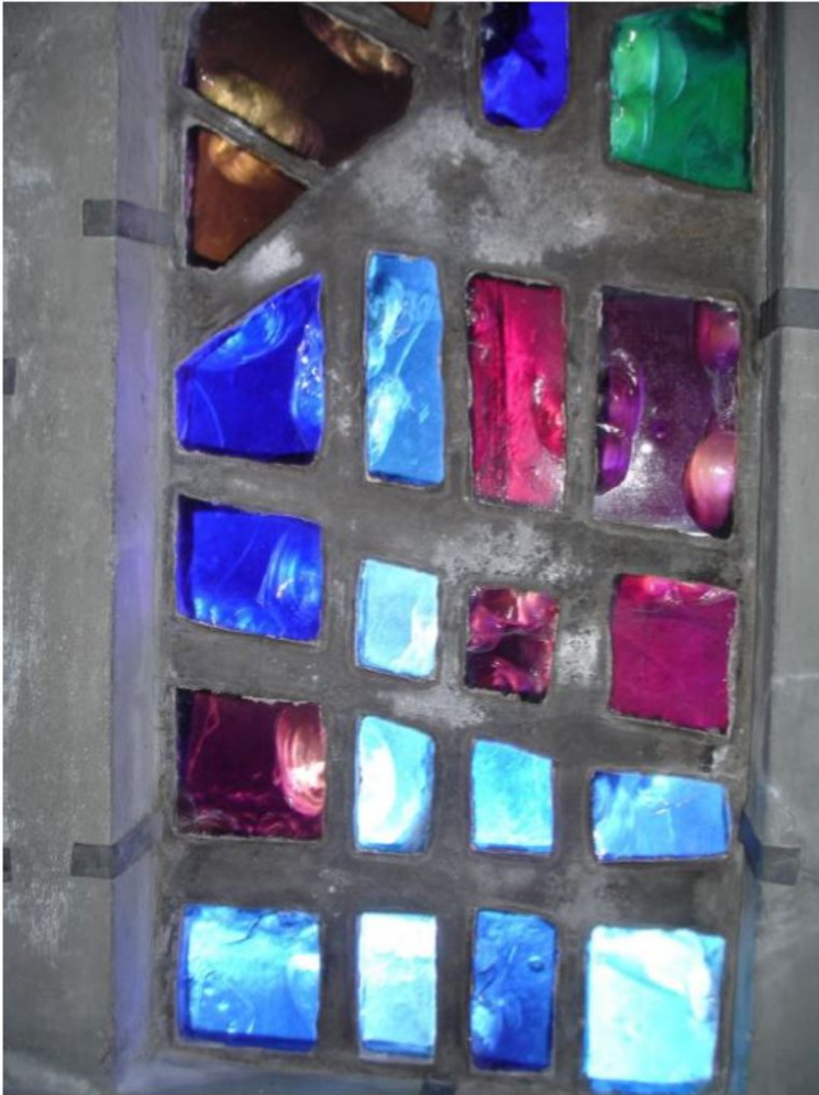
Figure 11 (L): Sanctuary detail of original dalle de verre in north claustra wall Photographer Jane Love, 2016
