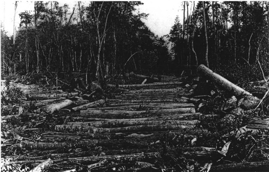
One method of railroad construction in Okefenokee, foundation ready for stringers (Hopkins, 45 Years with the Okefenokee Swamp , 1947).
