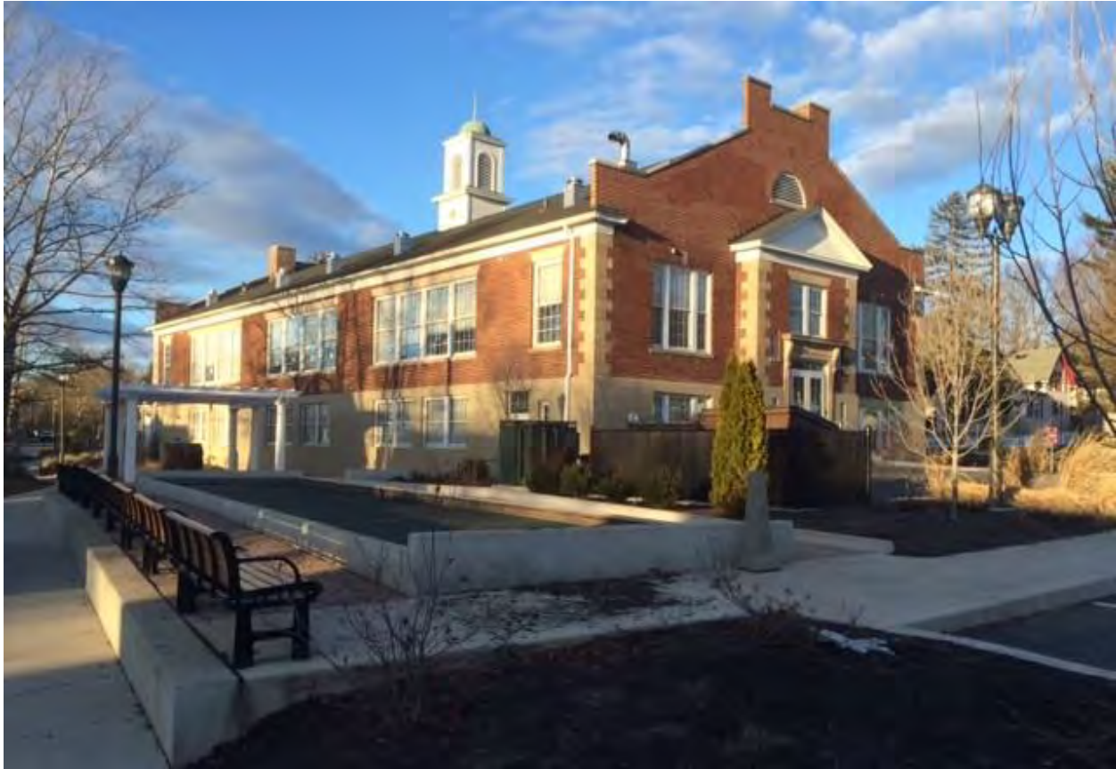
FIGURE 9 - Eckersley Hall School (61 Durant Terrace, Middletown, CT) c.1929, camera facing north.
