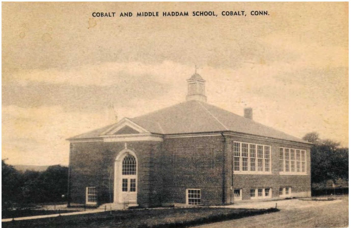
FIGURE 4: Middle Haddam School - south and east elevations of original 1931 block - from 1934 Postcard (mislabeled Cobalt, Connecticut), photographer unknown, published by the Cobalt General Store, camera facing northwest
