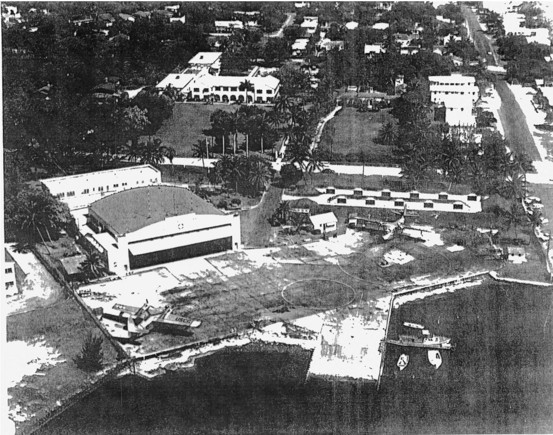
U.S. Coast Guard Air Station Hangar at Dinner Key, Miami, Miami-Dade Co., FL Photograph 21 of 21
