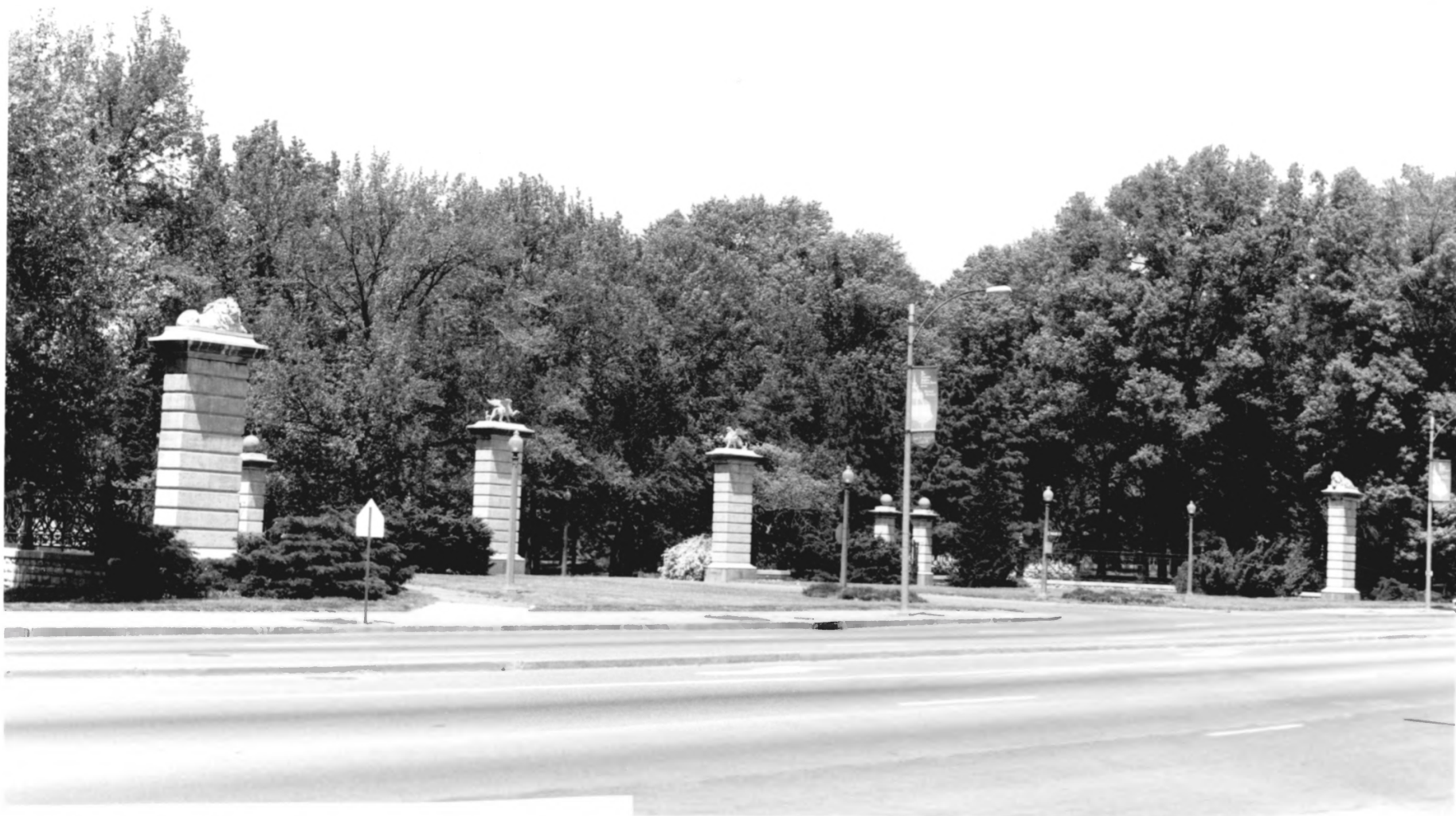
TOWER GROVE PARK, St. Louis, Missouri East Gate, Grand Avenue, view from southeast Esley Hamilton, 1988
