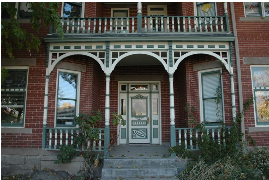
Photograph 2 East elevation of house, porch detail. Camera facing west.
