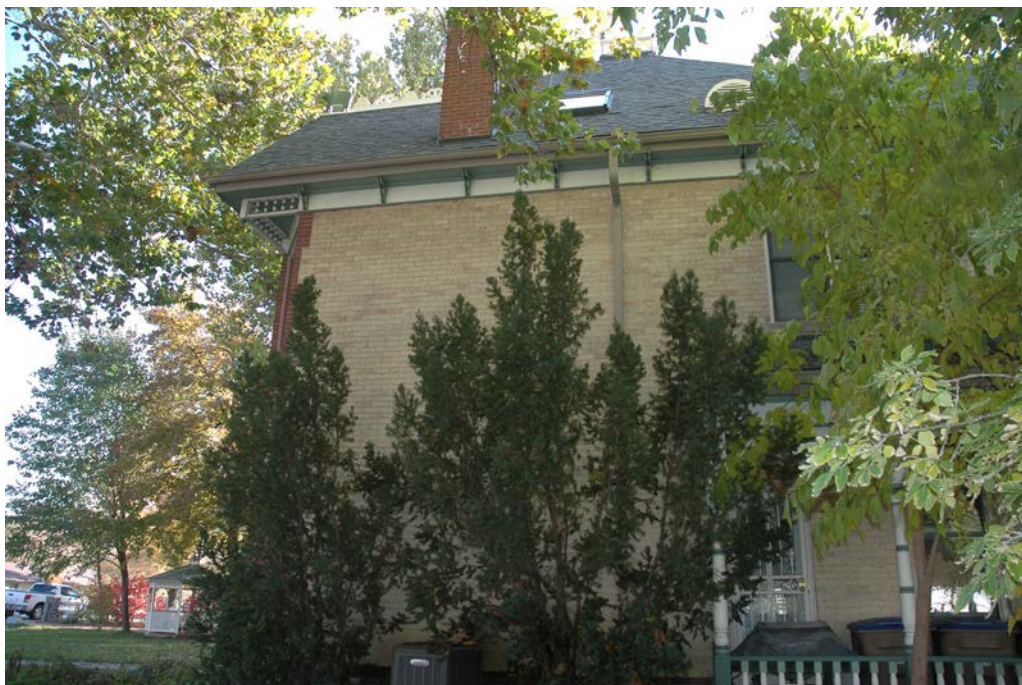
Photograph 4 North elevation of house. Camera facing south.
