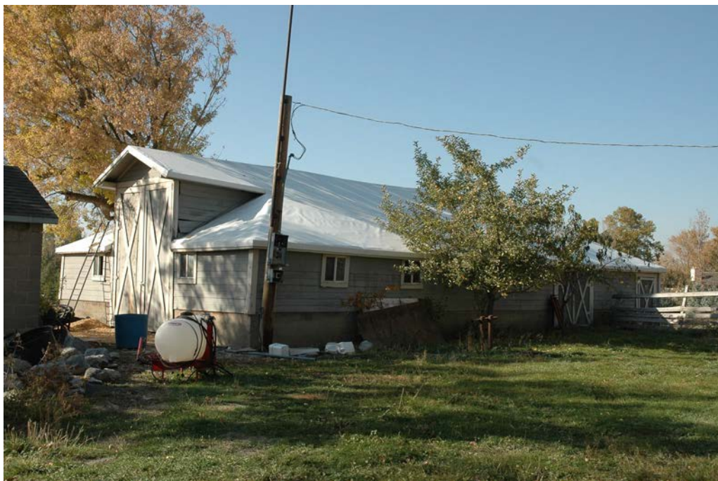
Photograph 14 Barn, circa 1942 (contributing building). Camera facing northwest.
