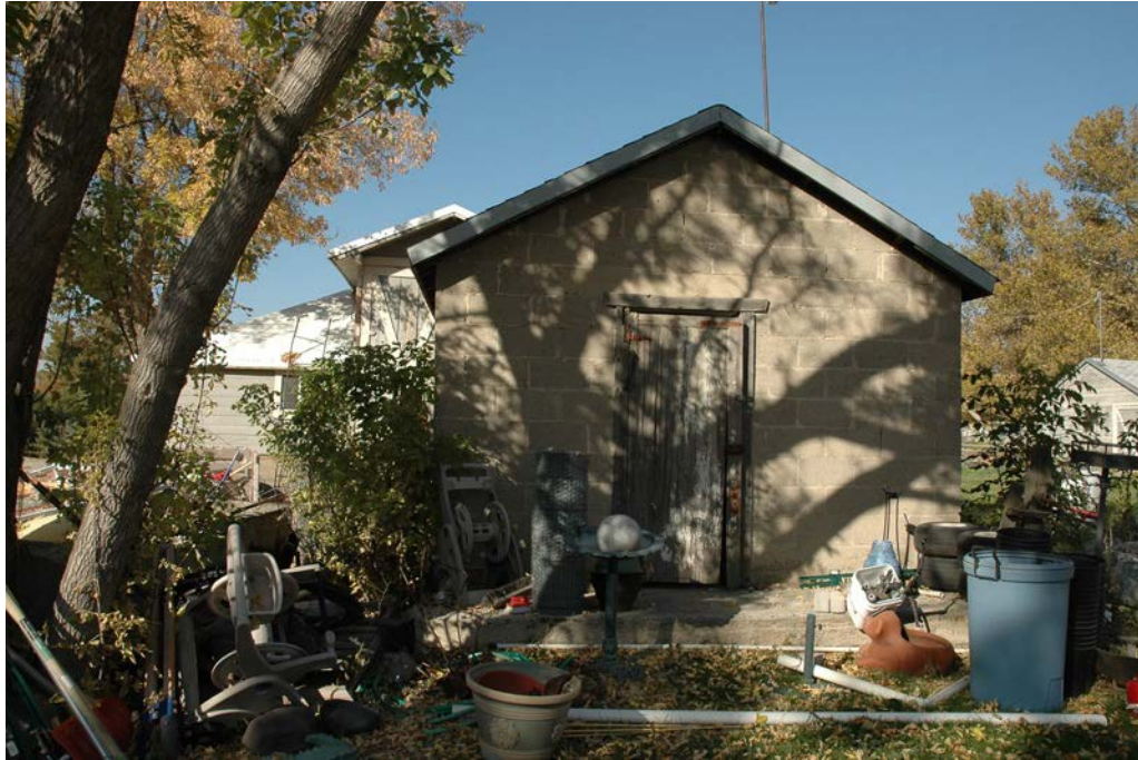
Photograph 15 Tool shed, circa 1956 (contributing building). Camera facing north.
