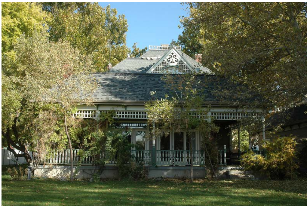
Photograph 6 West elevation of addition. Camera facing east.
