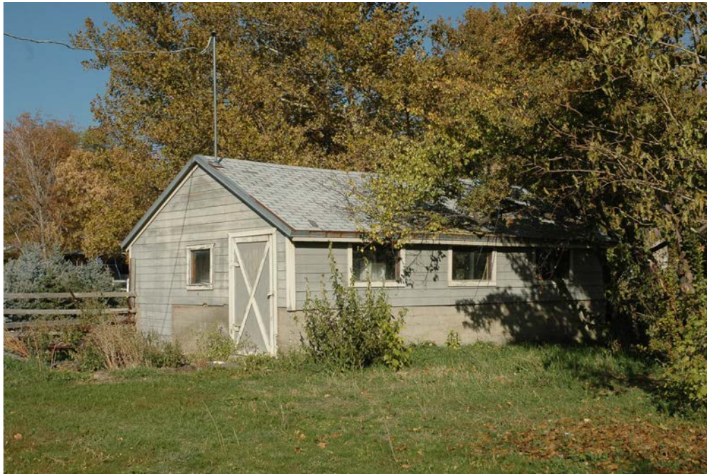
Photograph 13 Animal shed, circa 1942 (contributing building). Camera facing northeast.
