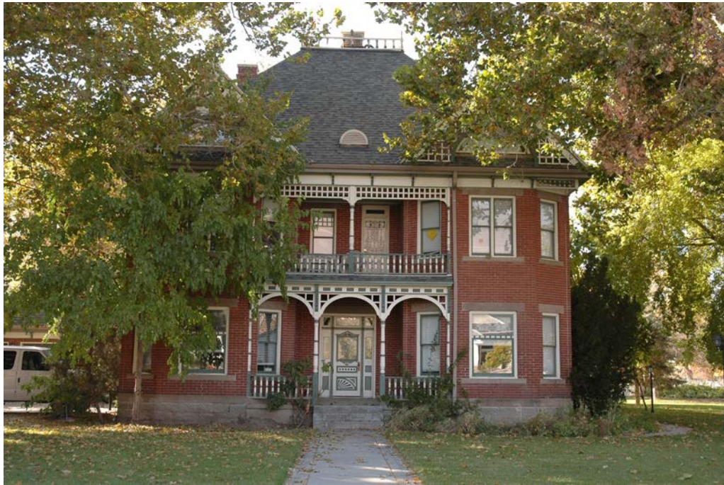
Photograph 1 East elevation of house. Camera facing west.
