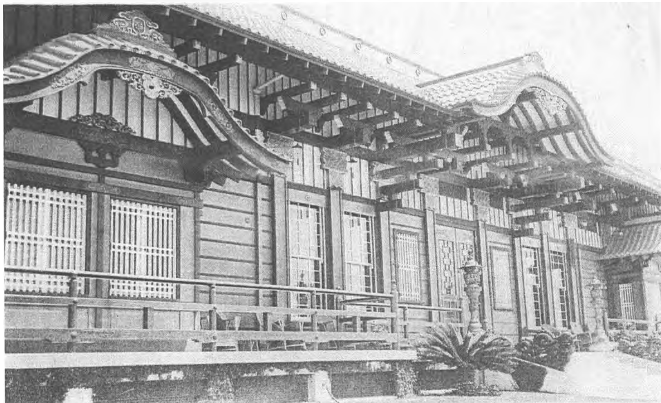
Main House, south façade detail, 1914. Source: Los Angeles Public Library.
