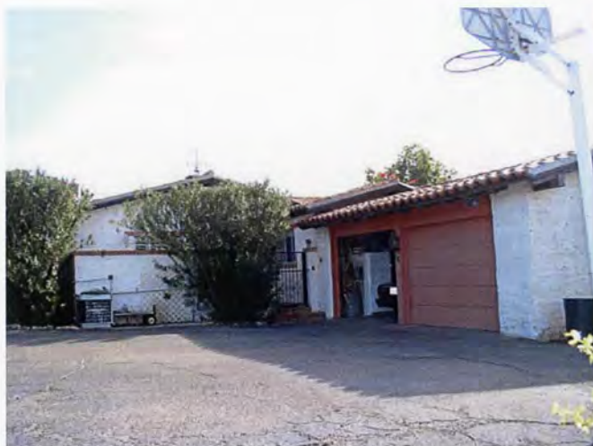
Photograph #3 View of west facade and garage looking east.
