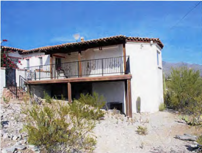
Photograph #5 Angled view of east facade and octagon addition looking north.
