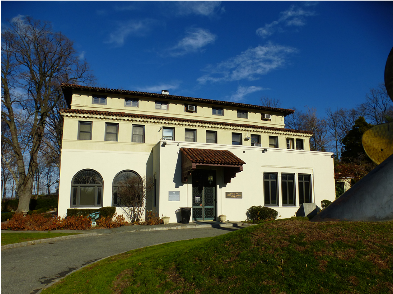
Photo 5. View to north of the front facade.
