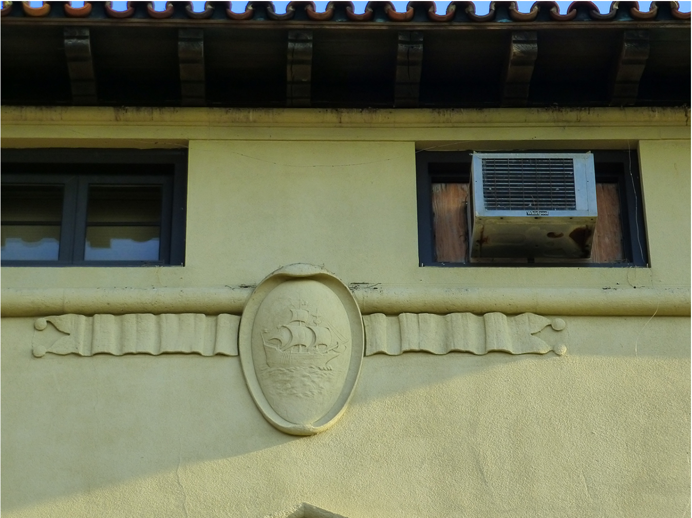
Photo 10. View to the east of the medallion on the third floor belt course.
