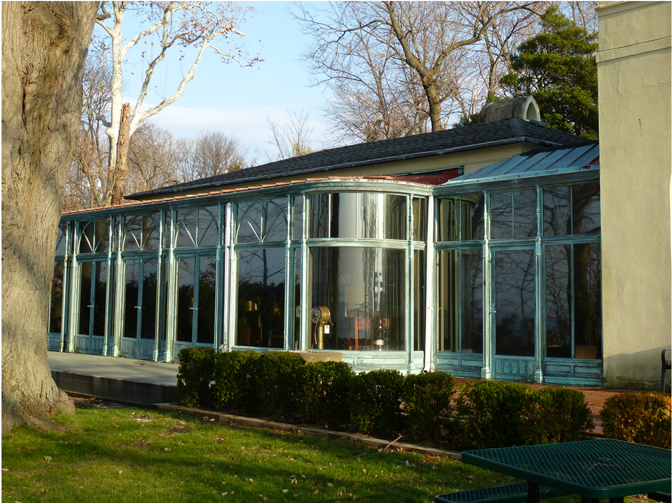
Photo 11. View to the northeast of the solarium on the west facade of the music room addition.
