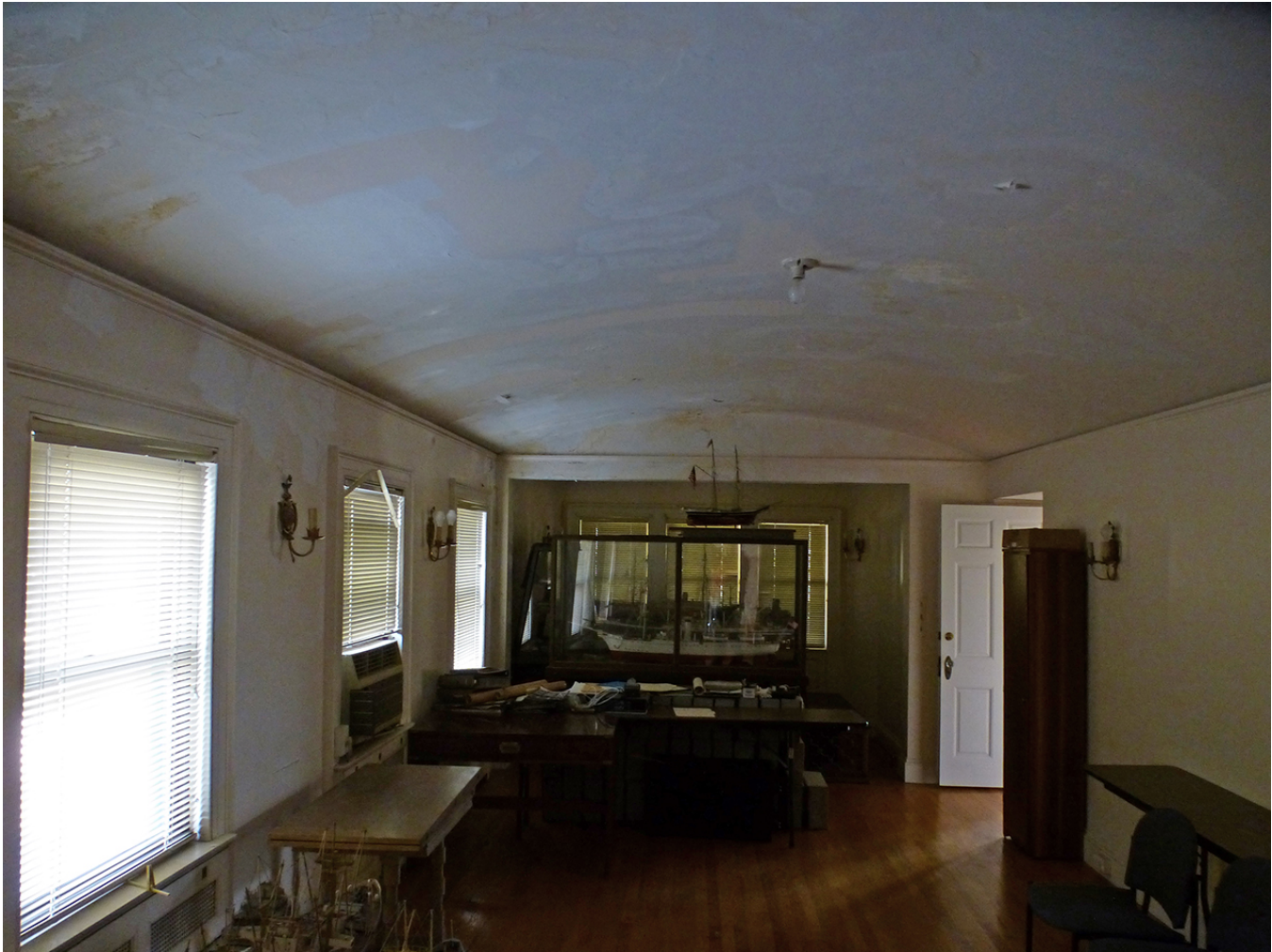
Photo 40. View to the east of the northeast bedroom.
