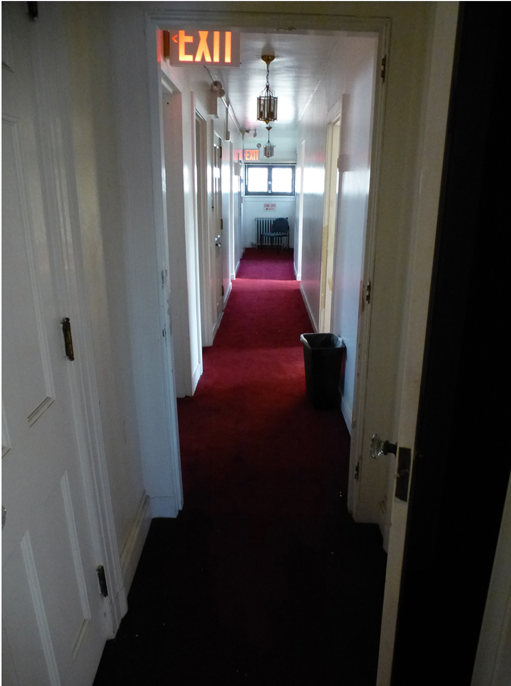
Photo 45. View to the east of the third-floor hallway.
