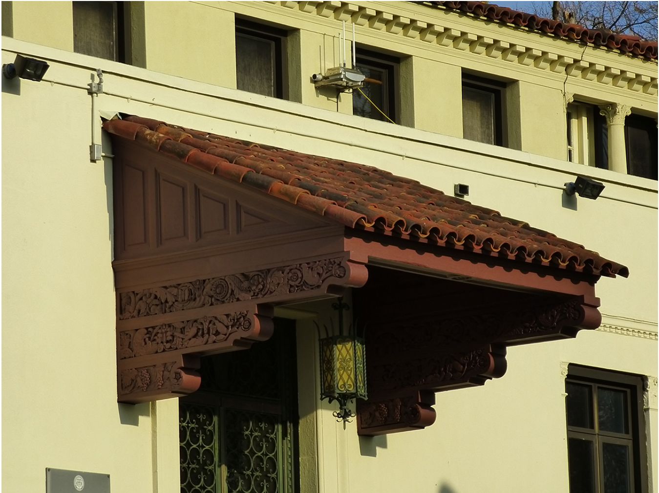
Photo 6. View to the north of the pent roof over the front door.
