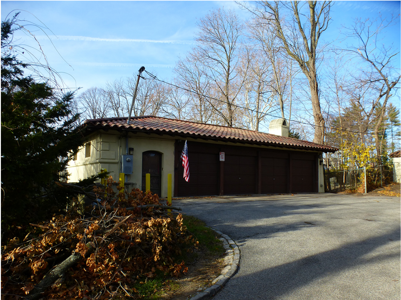
Photo 52. View to the northwest of the entrance door and garage doors on the east facade of the garage building.
