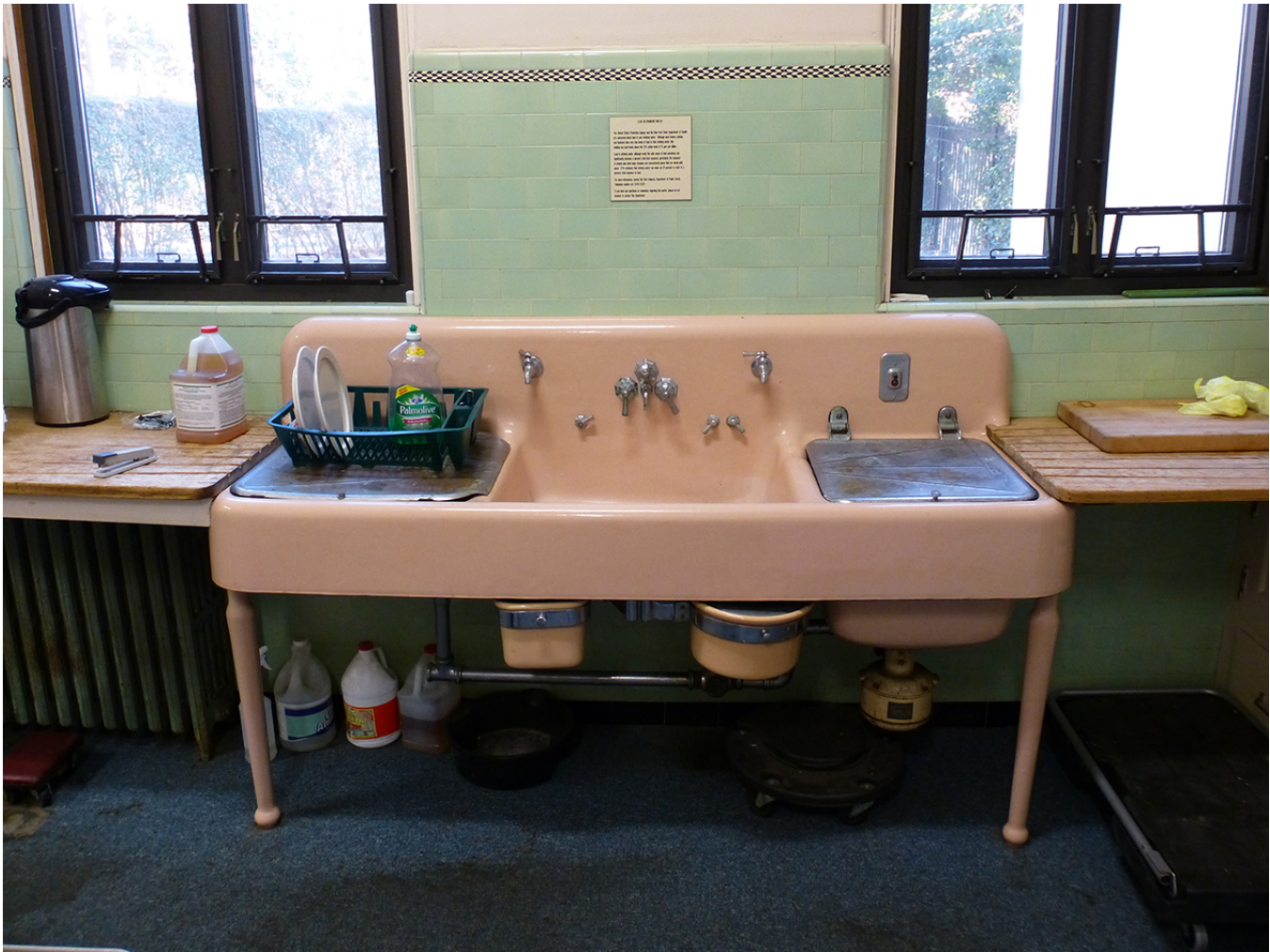
Photo 32. View to the east of the sink in the butler's pantry.
