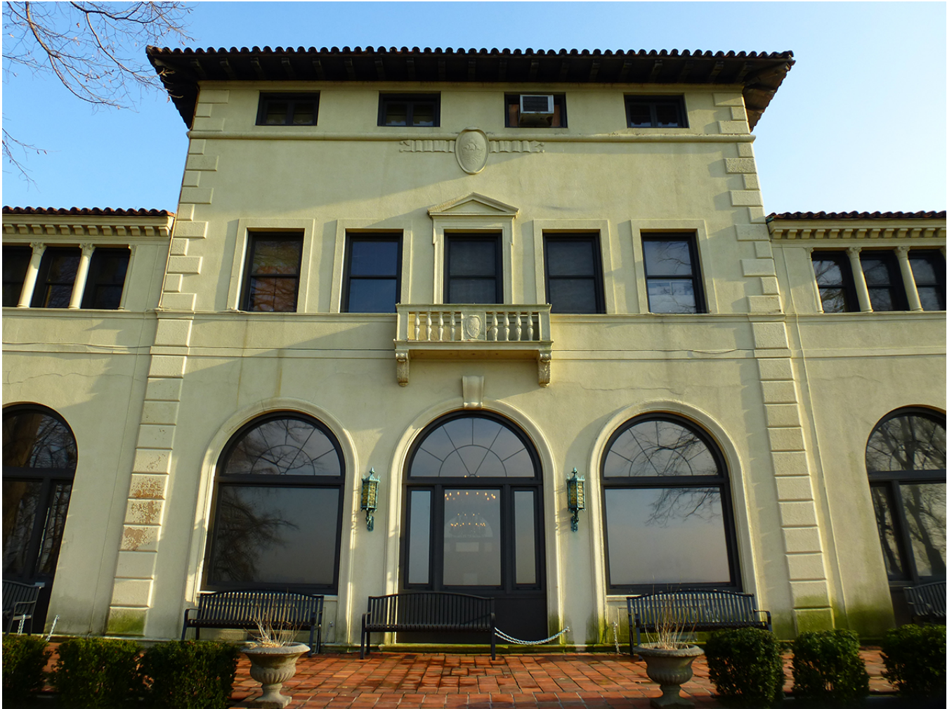
Photo 8. View to east of the west facade and the terrace.
