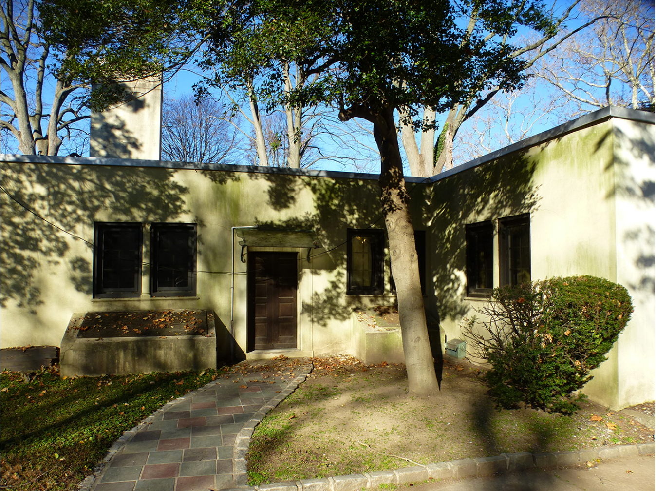
Photo 13. View to the west of the north entrance door into the music room addition.
