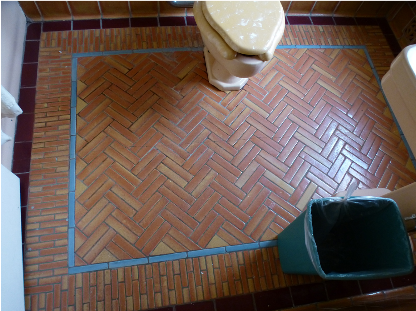
Photo 41. View to the west of the tile floor in the northeast bathroom.
