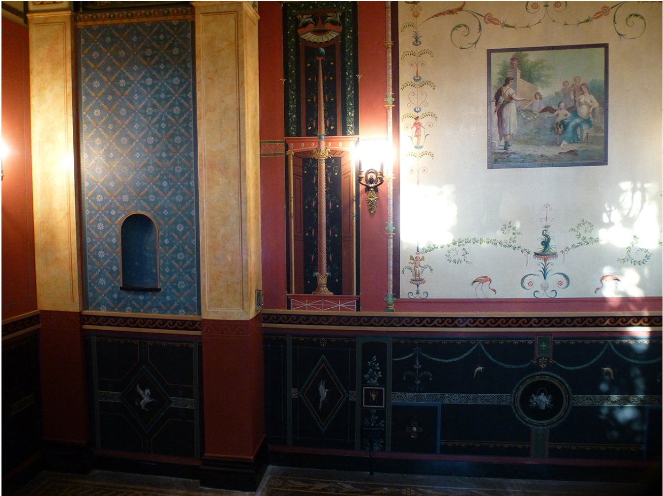
Photo 30. View to the north of painted wall in the breakfast room.
