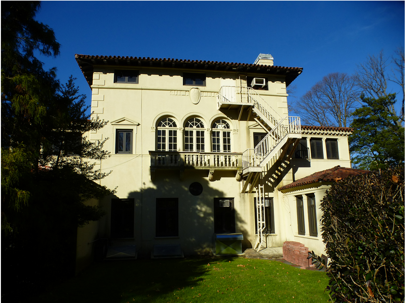
Photo 15. View to the west of the east facade.
