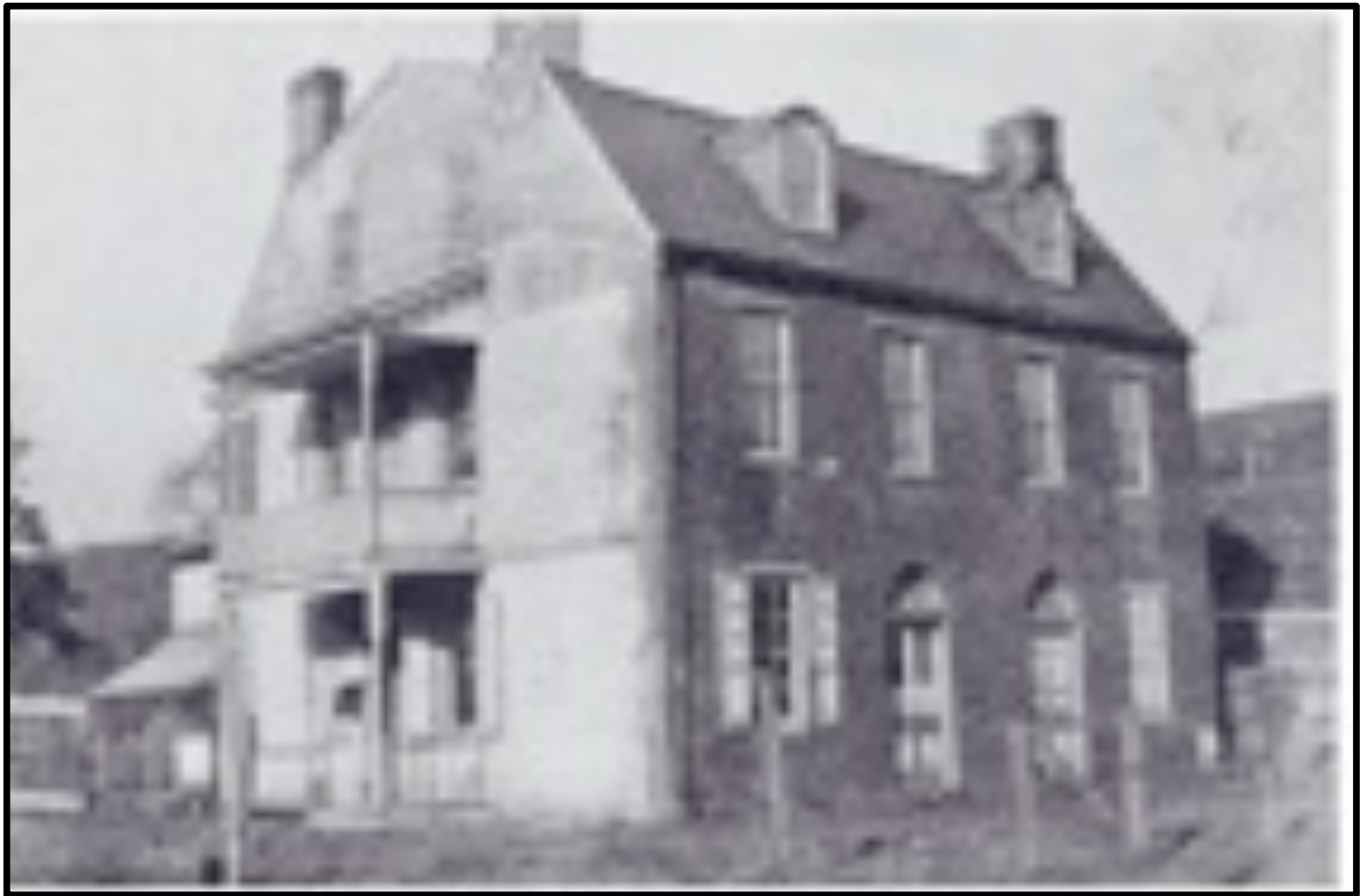
Figure 5. Hixson-Mixsell House, c. early 20th century. The ghost of an earlier full-width porch is clearly visible on the south facade. The paired entries and dormers on the east facade have been restored based on this photo and other evidence [Collection of Alice Hnat, as printed in Frank Leary, Pohatcong: the Prologue , page 62].
