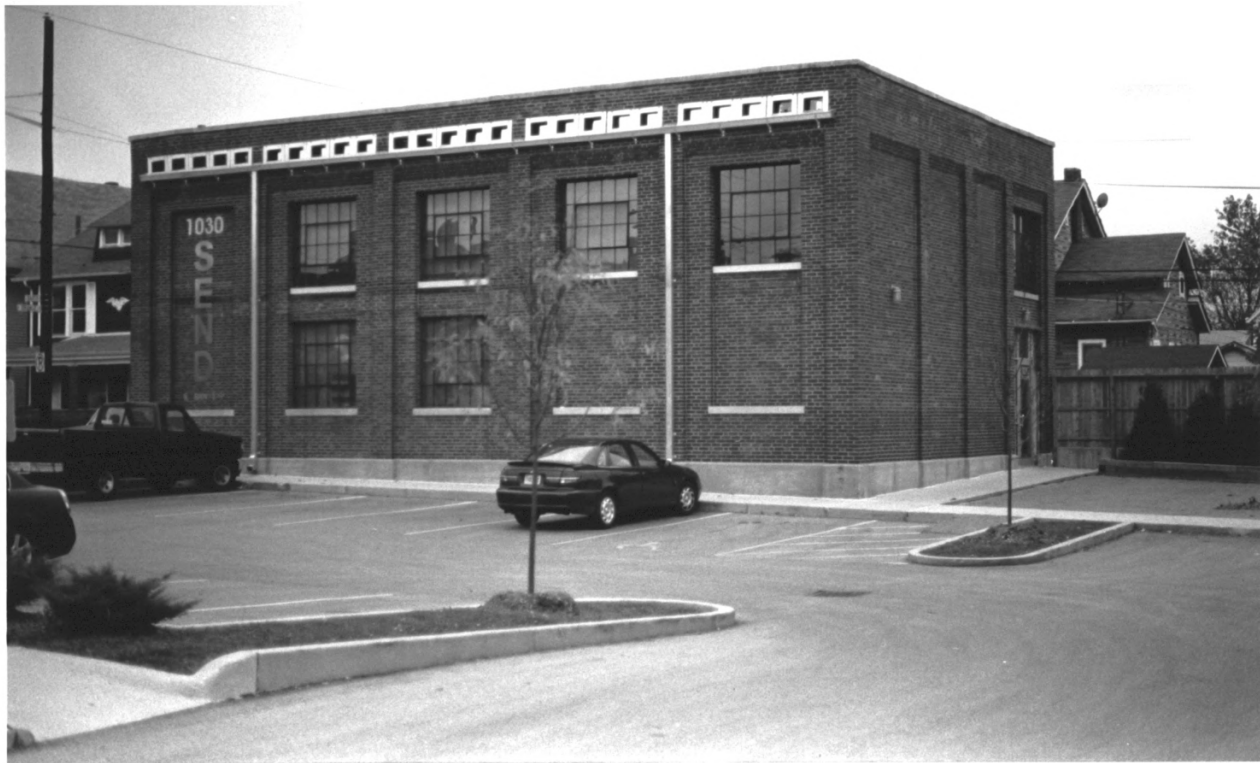
WHEELER ARTS BUILDING INDIANAPOLIS, MARION CO., INDIANA
