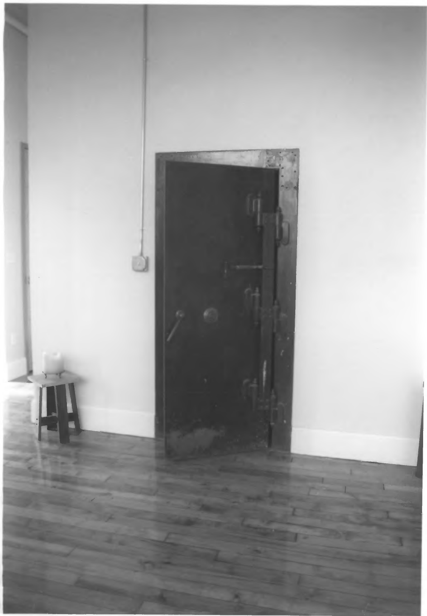
WHEELER ARTS BUILDING INDIANAPOLIS, MARION CO. IN. #4
